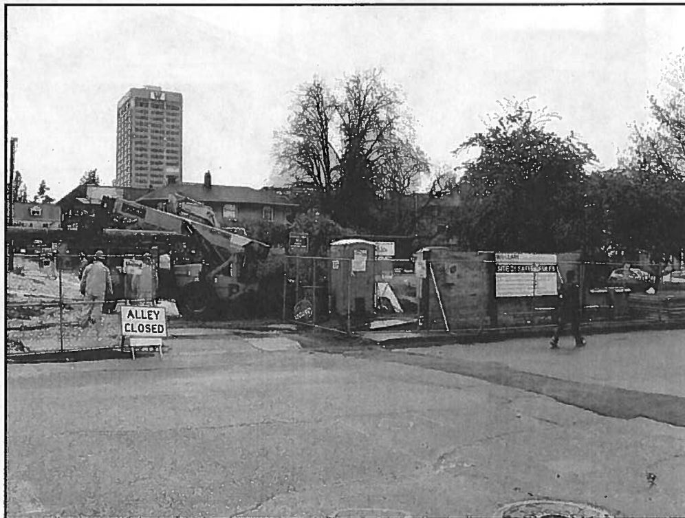
Figure 18. Site preparation work at Site 31W. Photograph faces north.
