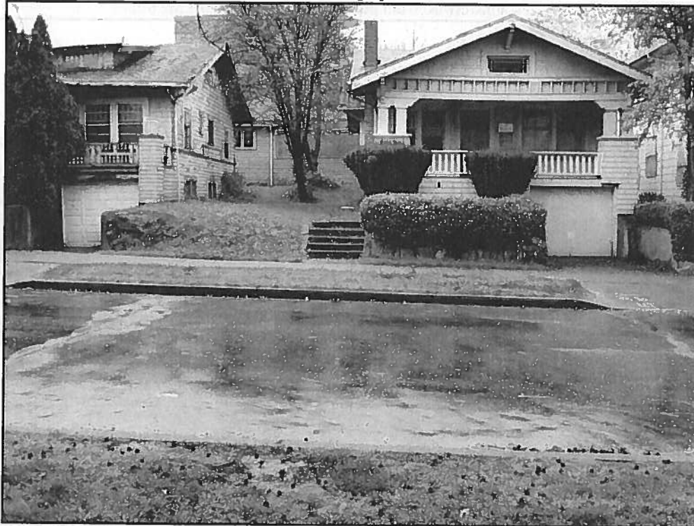
Figure 20. Conditions in the western half of Site 32W, where yards have been filled and graded above street elevation. Photograph faces east.
