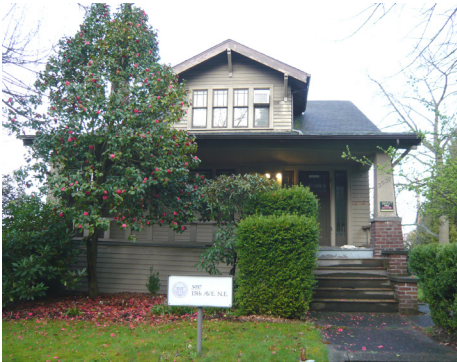
View of 3937 15th Avenue NE from Street
