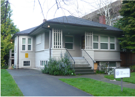
View of 3945 15th Avenue NE from Street
