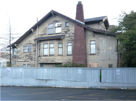
South Facade of 3937 15th Avenue NE
