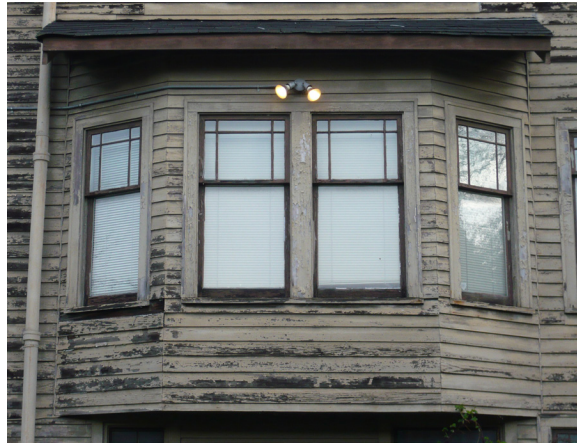
Closeup of South Facade of 3937 15th Avenue NE
