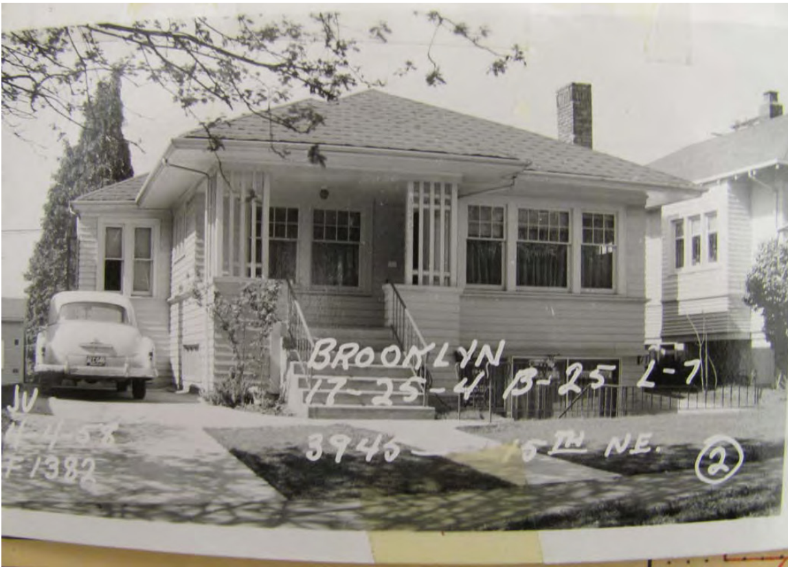
View of 3945 15th Avenue NE from Street
