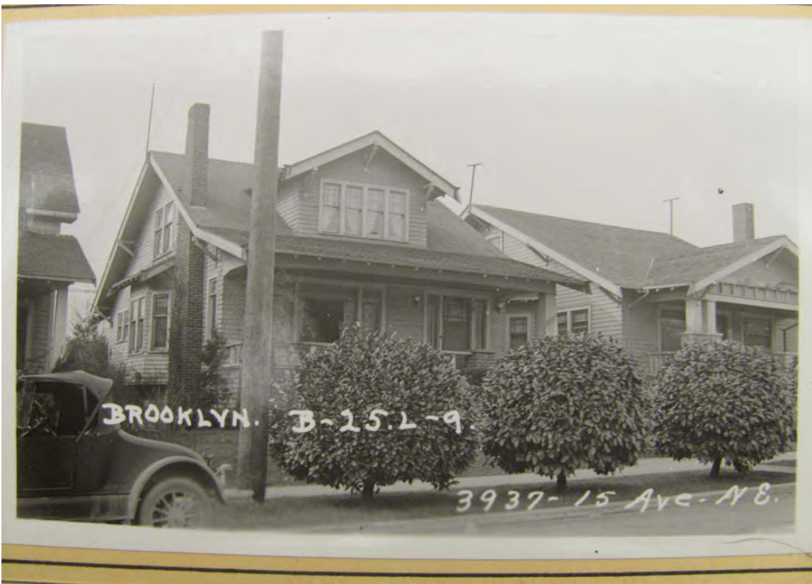
View of 3937 15th Avenue NE from Street
