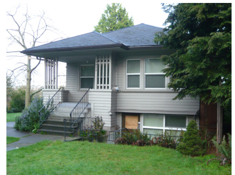
View of 3945 15th Avenue NE from Street
