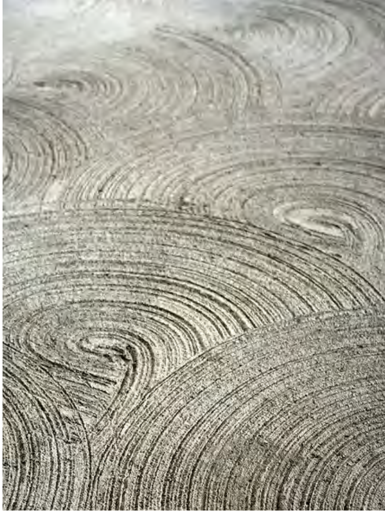
BRUSHED CONCRETE TEXTURE
