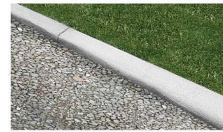
Restrained Concrete Curb
