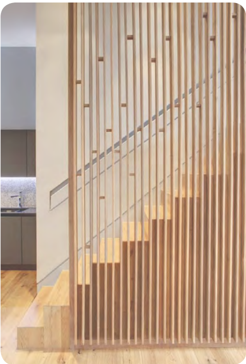
2. Wood screen on Basement 1 stairs carried through from exterior headhouse wall
