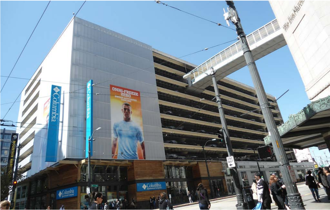
3 RD & PINE PARKING GARAGE DANPALON POLYCARBONATE
