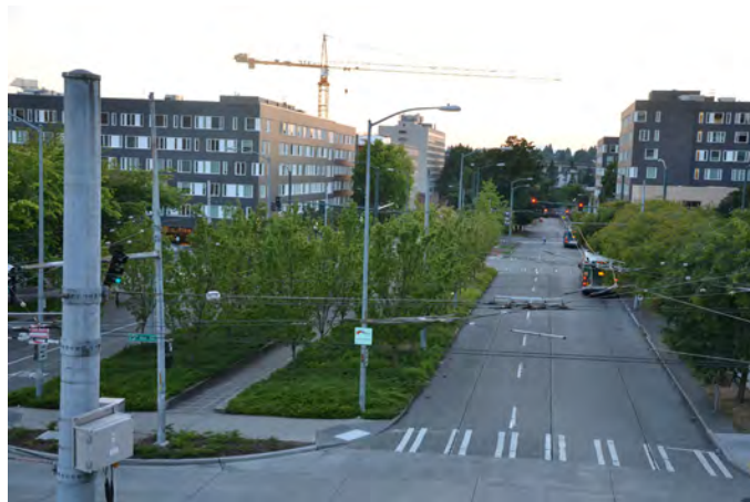
11. NORTH EAST CAMPUS PARKWAY POTENTIAL DISCUSSION: LANDSCAPE SPATIAL CONFIGURATION AND ECOLOGICAL FUNCTION, URBAN HYDROLOGY
