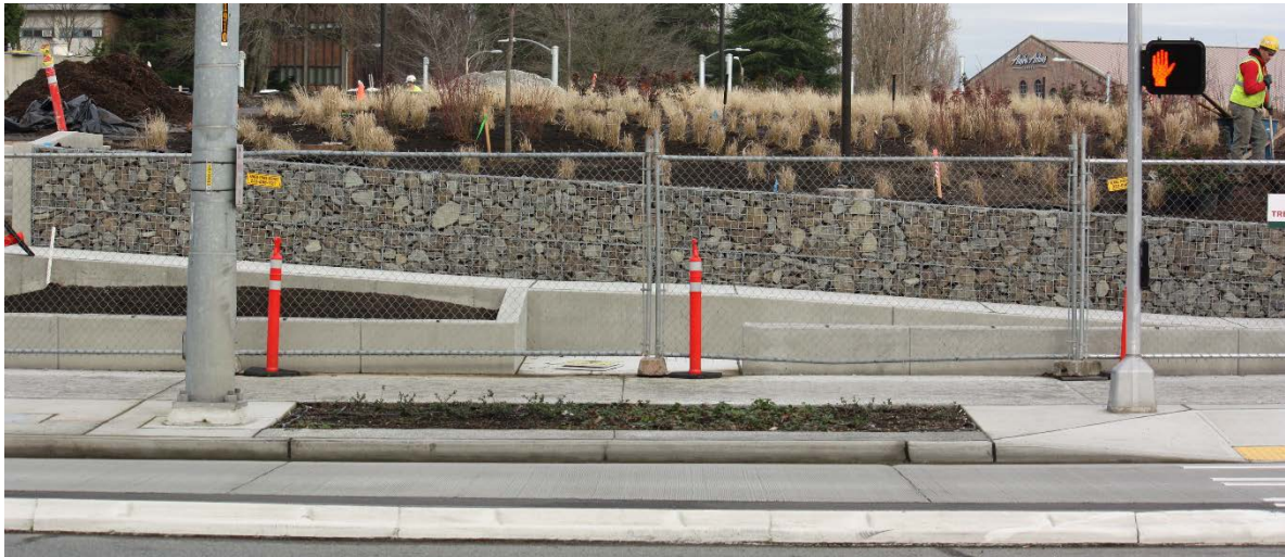
Montlake Triangle retaining walls
