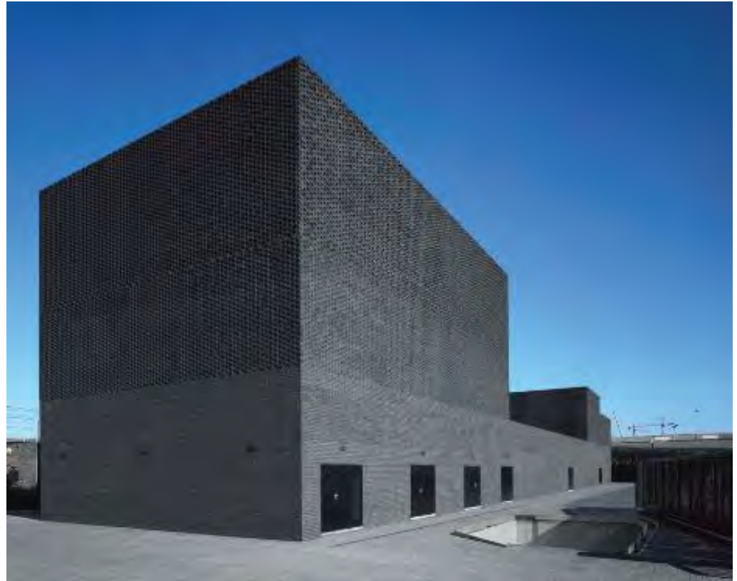
PRIMARY SUBSTATION 2012 OLYMPICS - NORD ARCHITECTURE
