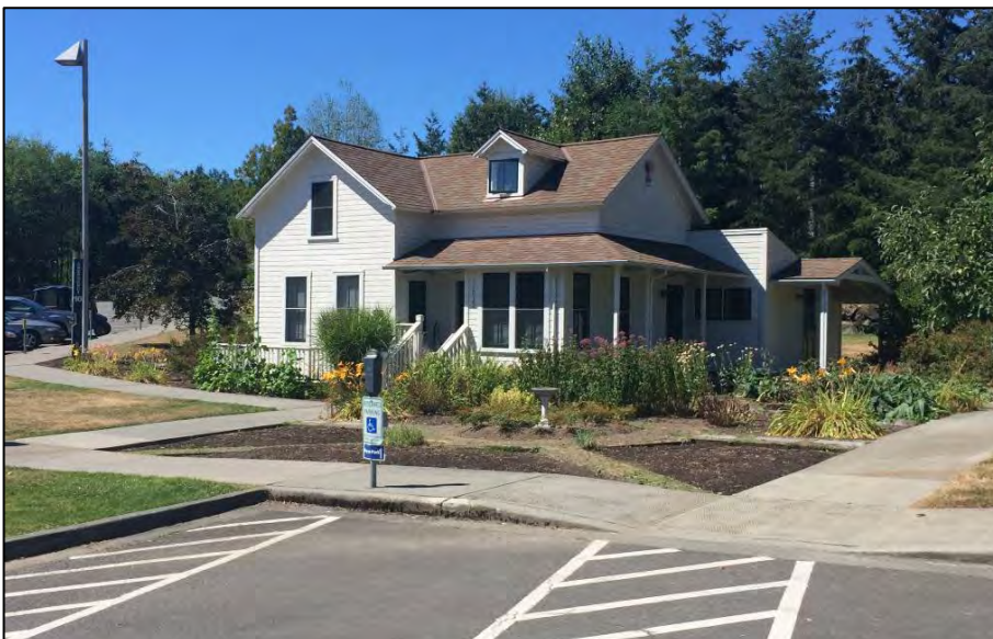
Below, the present day Chase Residence, view looking west (BOLA, July 29, 2016).
