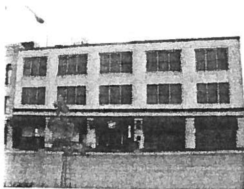
AUGUST 2007 VIEW OF THE WEST (FRONT) FACADE. CANOPIES OVER STOREFRONTS HAVE BEEN UPDATED. BUILDING HAS BEEN PAINTED. SOURCE: ARTIFACTS CONSULTING, INC.
