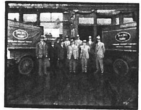
APRIL 30, 1927 VIEW OF THE EAST FACADE. YOUNGLOVE GROCERY CO. TRUCKS IN FRONT OF 1932 AND 1930 PACIFIC AVE. YOUNGLOVE GROCERY CO. OCCUPIED 1932 PACIFIC AVE. ON AND OFF OVER THE YEARS BETWEEN 1907-1914. SOURCE: TACOMA PUBLIC LIBRARY. BOLAND PHOTOGRAPH COLLECTION #816769
