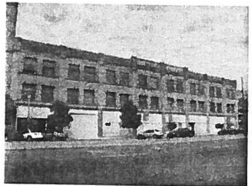
AUGUST 2007 VIEW OF THE EAST (FRONT) FACADE. THE STOREFRONTS ARE ALMOST ENTIRELY BOARDED UP AS THE BUILDING SITS VACANT TODAY. SOURCE: ARTIFACTS CONSULTING, INC.
