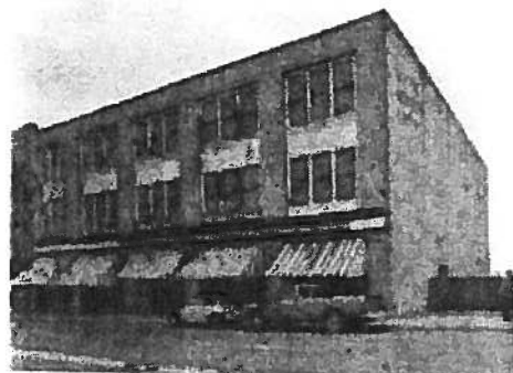
CA. 1970 VIEW OF THE WEST (FRONT) AND SOUTH FACADES. FLAT ROOF CANOPY HAS BEEN REMOVED. FIVE INDIVIDUAL CANOPIES OVER EACH STOREFRONT HAVE BEEN ADDED. WEST FACADE OVERHANG EXTENDING OUT FROM ROOF HAS BEEN REMOVED. BUILDING HAS RECEIVED A FRESH NEW PAINT JOB OF MUSTARD YELLOW. OUTDOOR ADVERTISING HAS BEEN PAINTED OVER, WITH A NEW ADVERTISEMENT FOR THE OLD SPAGHETTI FACTORY NOW ADORNING THE SOUTH FACADE. SOURCE: TACOMA PUBLIC LIBRARY. RICHARDS STUDIO PHOTOGRAPHY COLLECTION
