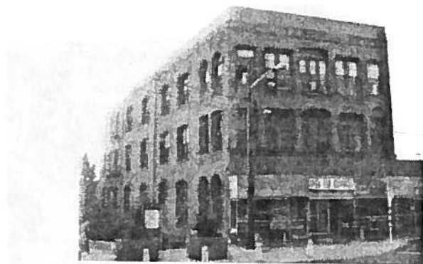
TOOGA BUILDING'S NORTH AND WEST FACADES. SOURCE: ARTIFACTS CONSULTING, INC.
