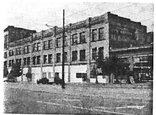
AUGUST 2007 VIEW OF THE EAST (FRONT) AND NORTH FACADES. NOTICE THE HEIDELBERG BREWERY OUTDOOR ADVERTISEMENT WHICH HAS ADORNED THE BUILDING SINCE THE 1930s. SOURCE: ARTIFACTS CONSULTING, INC.
