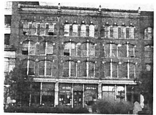
AUGUST 2007 VIEW OF THE EAST (FRONT) FACADE. SOURCE: ARTIFACTS CONSULTING, INC.
