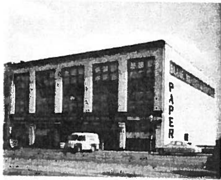
CA. LATE 1940S VIEW OF THE WEST (FRONT) AND SOUTH FACADES. OUTDOOR ADVERTISING FOR BLAKE, MOFFITT & TOWNE, INC. ADDITION OF FLAT ROOF CANOPY OVER TWO OF THE STOREFRONTS. SOURCE: TACOMA PUBLIC LIBRARY, RICHARDS STUDIO PHOTOGRAPHY COLLECTION.
