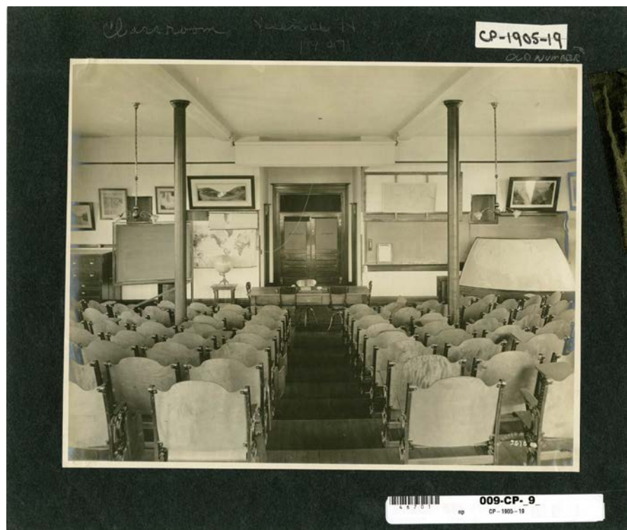
Figure 39. Geology Lecture Room, 1907 (likely 1st floor). UW Facilities Library.
