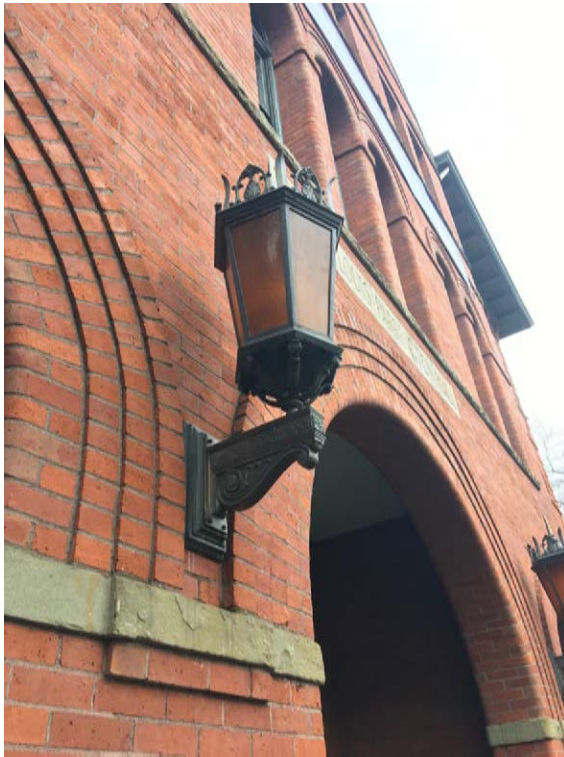
Figure 28. Detail of brickwork and lantern at primary entrance on south elevation.
