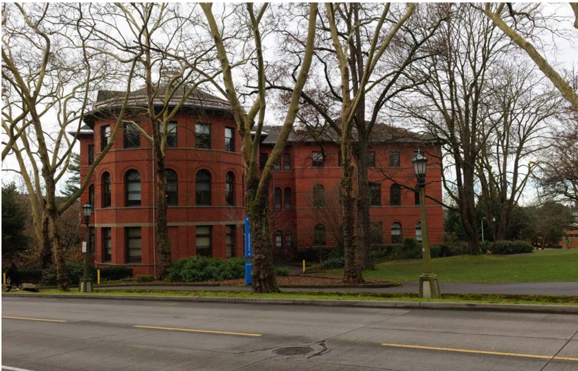
Figure 22. View looking south and west towards the building's east elevations.
