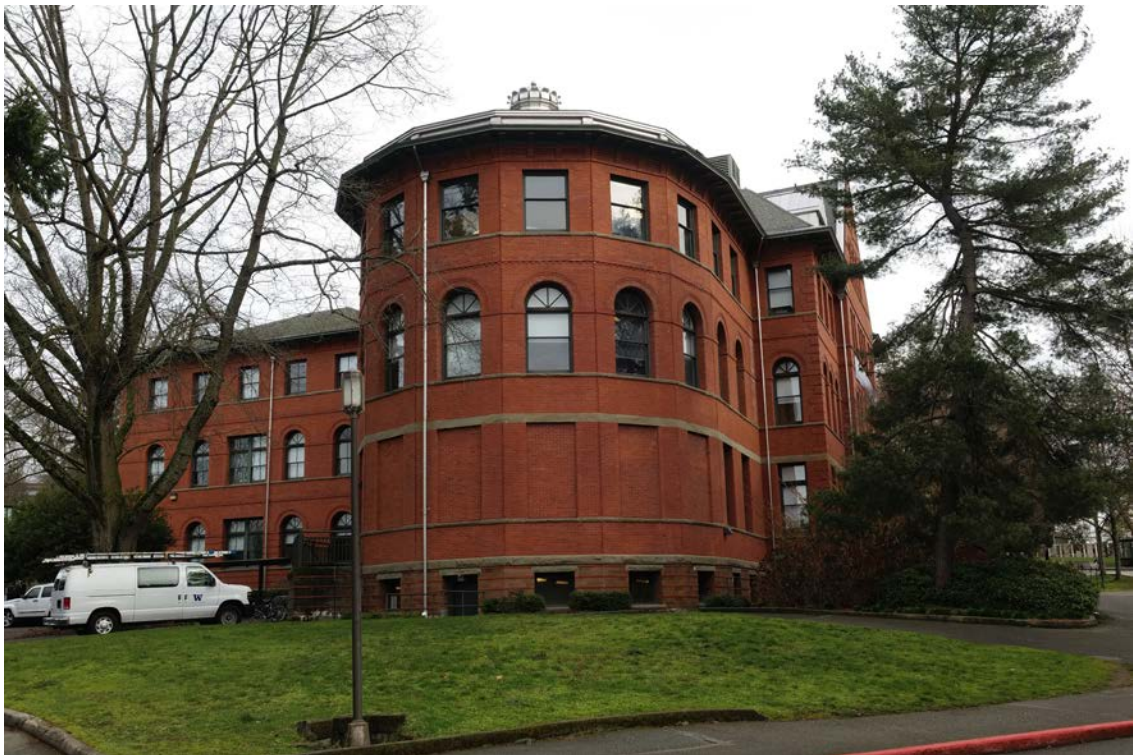
Figure 27. View looking east at the building's eastern curved wing.
