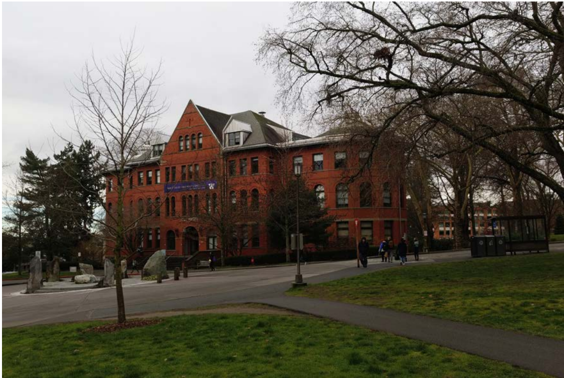
Figure 20. View looking northwest towards Parrington Hall showing its primary elevation and the eastern curved wing. A similar, historic view, is below.
