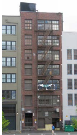
Figure 60. Front and rear elevations of the Bornstein and Sons, Inc. Warehouse, 526 1st Ave S (1909). (WISAARD, HPI form).
