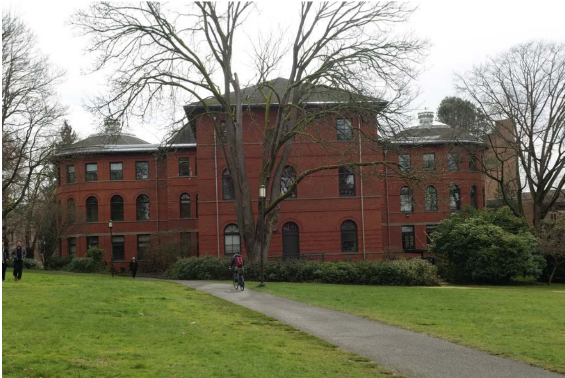
Figure 26. View looking south at the building's north elevation.
