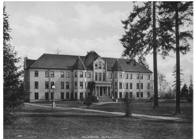
Figure 53. Exterior of Clarke Hall, University of Washington, ca. 1900-1936. (UW Special Collections UWC3210).
