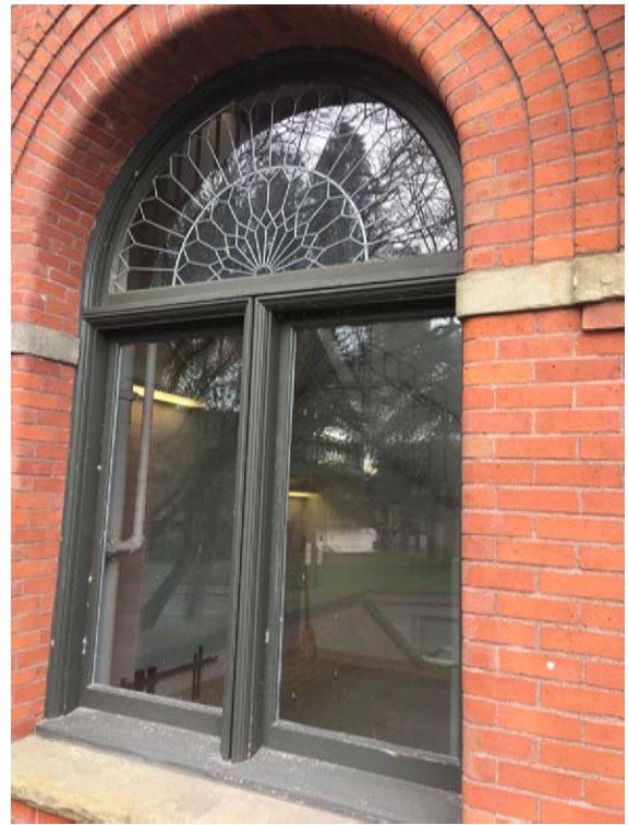
Figure 29. Detail of window with leaded glass arched transom, south elevation.
