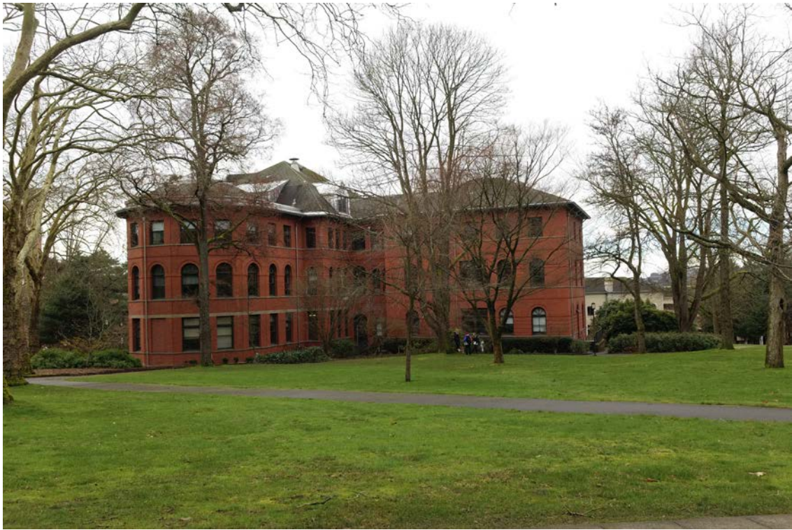
Figure 24. View looking west, across Parrington Lawn, at the building's east and north elevations.
