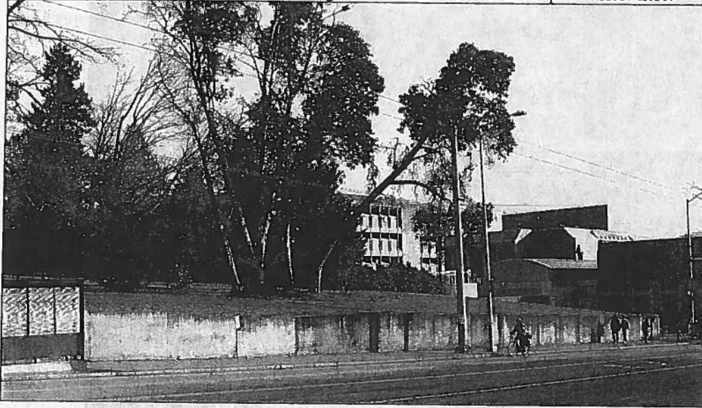
View southeast across 15th Avenue NE, showing the concrete retaining wall that forms the west edge of Parrington Lawn. A cluster of madronas are visible on the Lawn. (Photo by SvR Design.)
