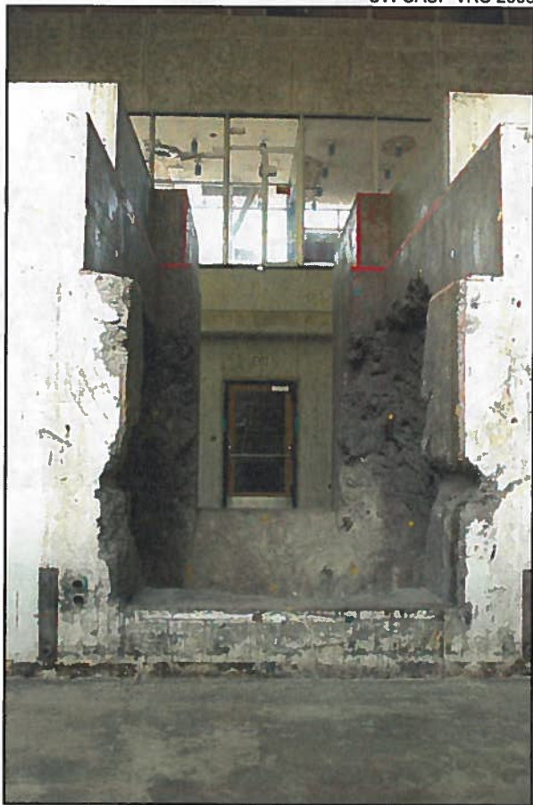
Figure 12 • Reactor room, viewing east
