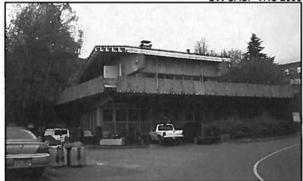
Figure 9 • East and partial south façades, lower level
