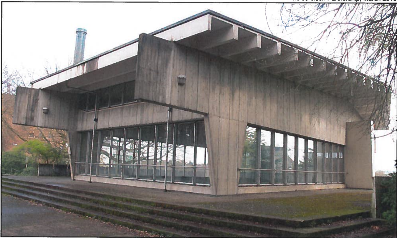
Figure 2 • More Hall Annex, northern and southern façades
