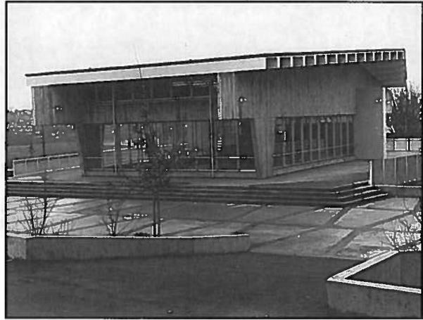
Figure 15 • West and east façades, 1963
