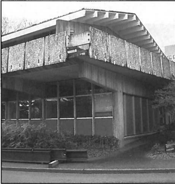
Figure 6 • Partial east and north façades, lower level
