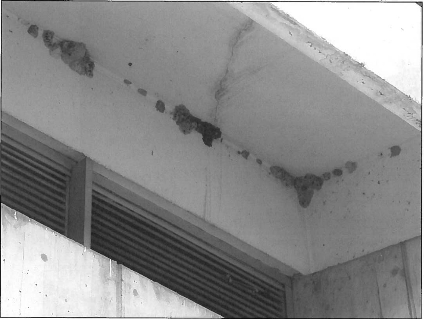
Figure 5 • More Hall Annex, detail of southern façade overhang
