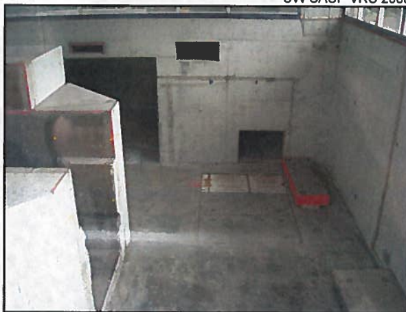
Figure 13 • Reactor room, viewing south
