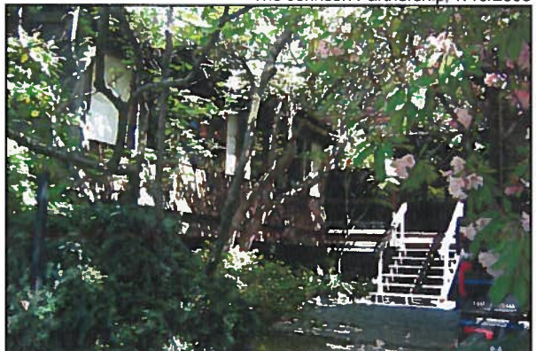
Figure 51 • Zema Office Building and Japanese Antique Gallery, Eastlake and Boston, Seattle, Zema, 1968
