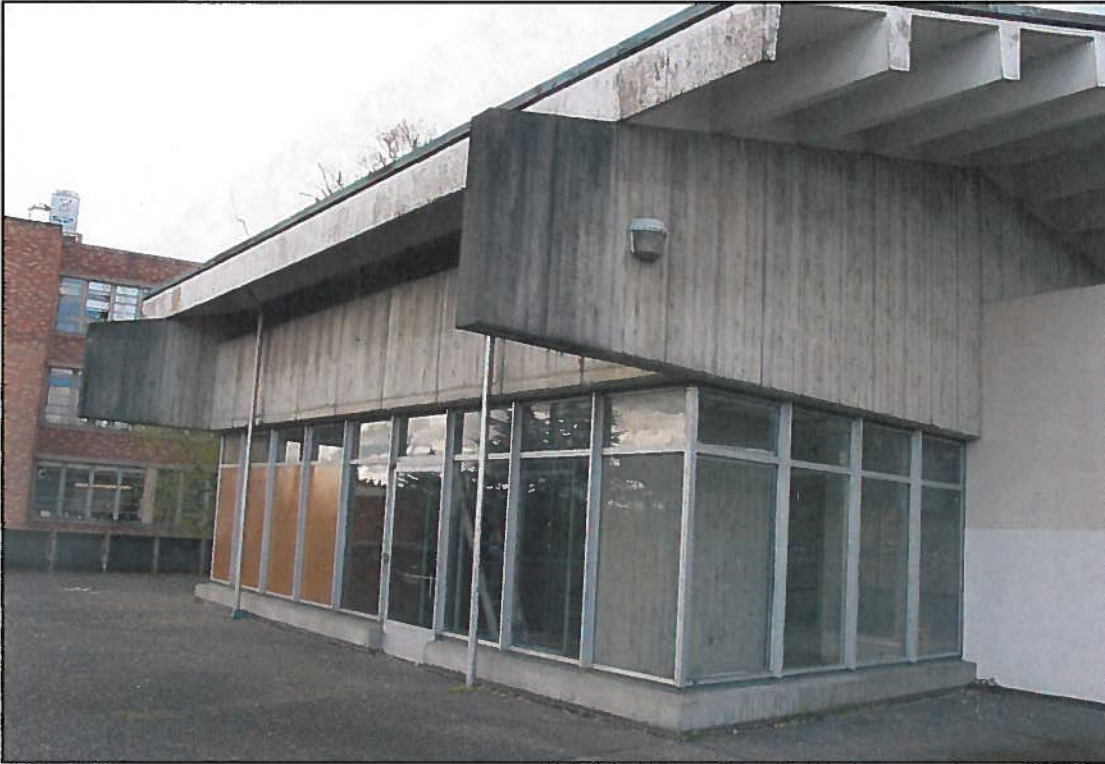
Figure 3 • More Hall Annex, eastern façade
