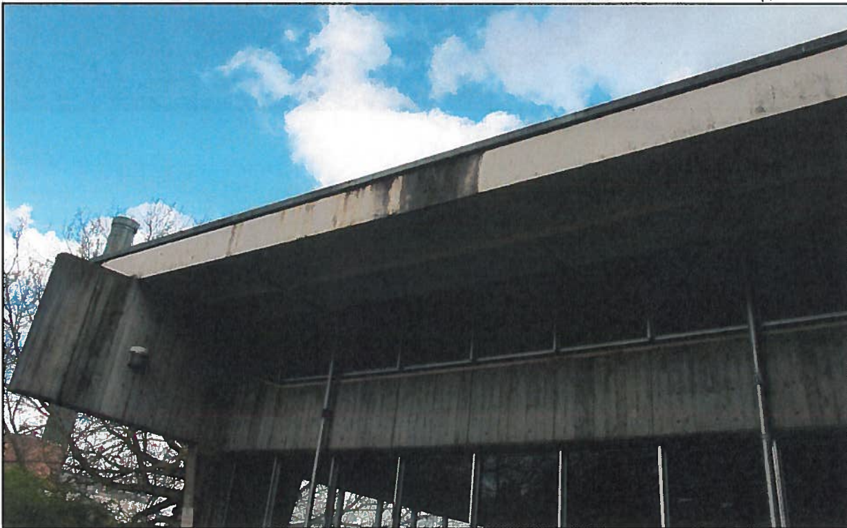
Figure 4 • More Hall Annex, detail of western façade overhang
