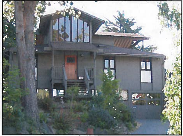
Figure 47 • 4234 51st Avenue NE, Seattle, Zema, 1962
