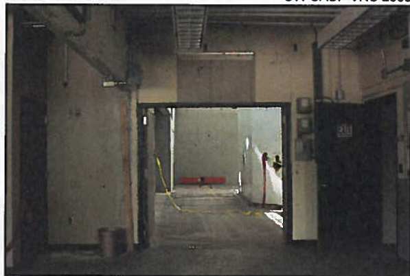
Figure 10 • Viewing west through dirty shop to reactor room beyond
