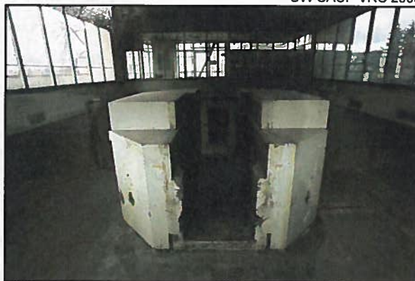
Figure 11 • Reactor room, viewing east from exterior
