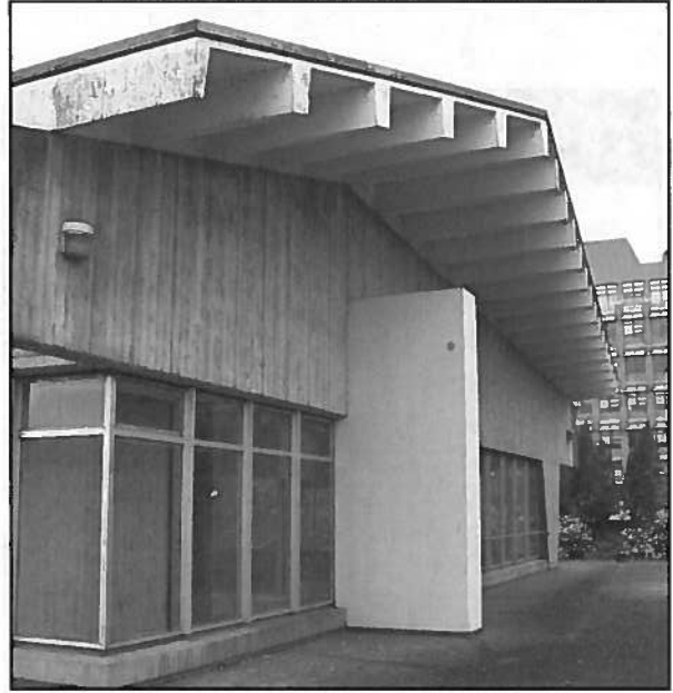
Figure 7 • North and partial east façade
