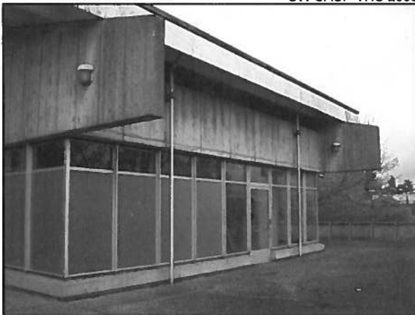
Figure 8 • East and partial south façades
