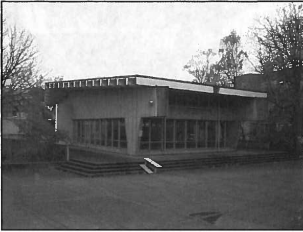
Figure 4 • North and west façades
