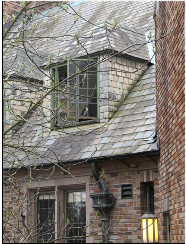
Above left, a view looking northwest at the south roof slope of the west wing of the building, showing the varied color, size and exposure of the original slates. Above right, views of two small slate-clad dormers on the back of the building, where the material was used for wall cladding as well as roofing. Note the copper gutters, downspouts, and scupper boxes in both views. Below, a detail view of the slate roofing near the small dormer.
