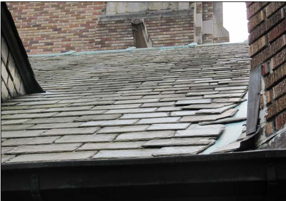
Above left, a view looking northwest at the south roof slope of the west wing of the building, showing the varied color, size and exposure of the original slates. Above right, views of two small slate-clad dormers on the back of the building, where the material was used for wall cladding as well as roofing. Note the copper gutters, downspouts, and scupper boxes in both views. Below, a detail view of the slate roofing near the small dormer.
