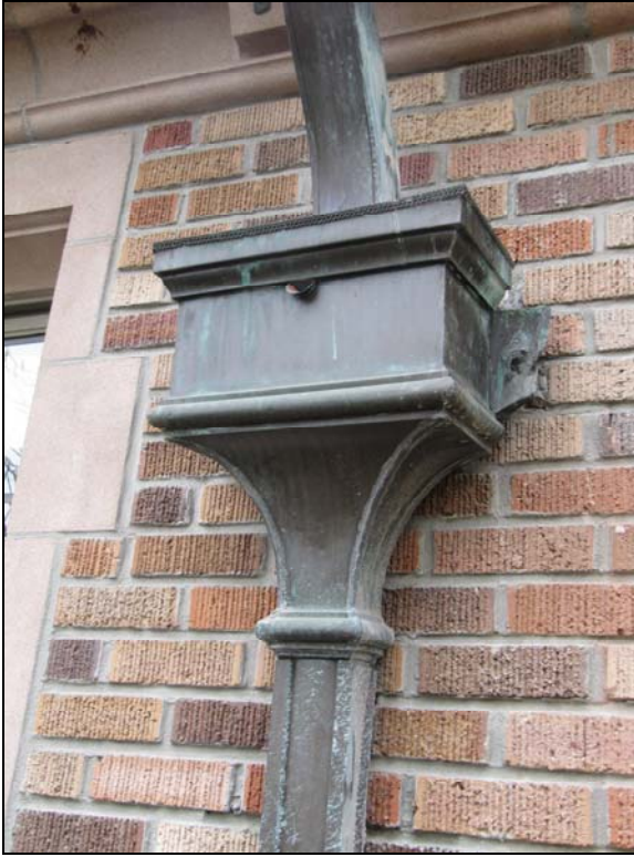
Above, views of copper downspouts and typical scupper boxes. Below, detail views of copper roof flashing, cast stone parapet cap, and copper ridge cresting.
