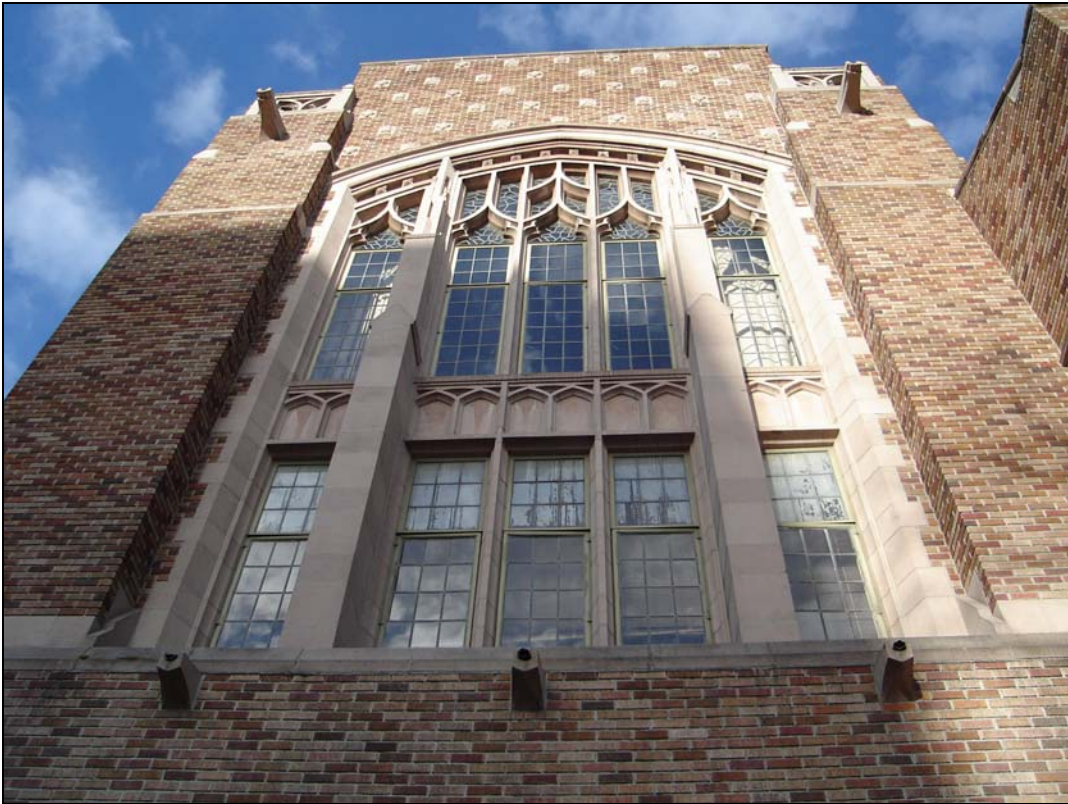
Top, the north facade. Directly above, view looking up at a large window assembly on the tower's west facade. The arched opening, tracery, cast stone surround and trim, and projecting scuppers are Gothic Revival features.
