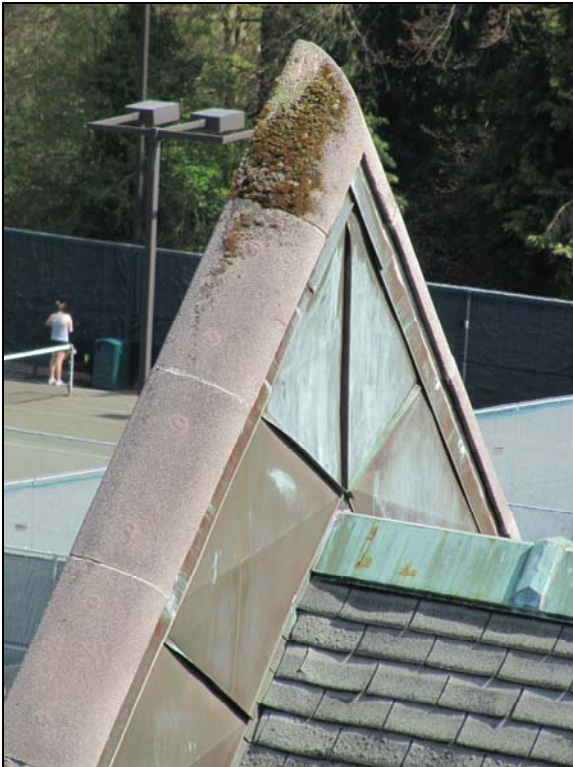
Above, views of copper downspouts and typical scupper boxes. Below, detail views of copper roof flashing, cast stone parapet cap, and copper ridge cresting.
