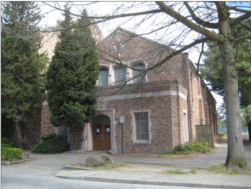
Top, partial view of the central part of the building's west facade. Above, oblique view of the entry and the west and south facades of the swimming pool wing. This wing currently contains Drama School studios and laboratory spaces. Note the close proximity of evergreen trees along the building's perimeter walls.
