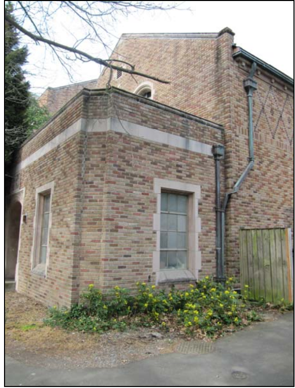
Above, views of copper downspouts and typical scupper boxes. Below, detail views of copper roof flashing, cast stone parapet cap, and copper ridge cresting.
