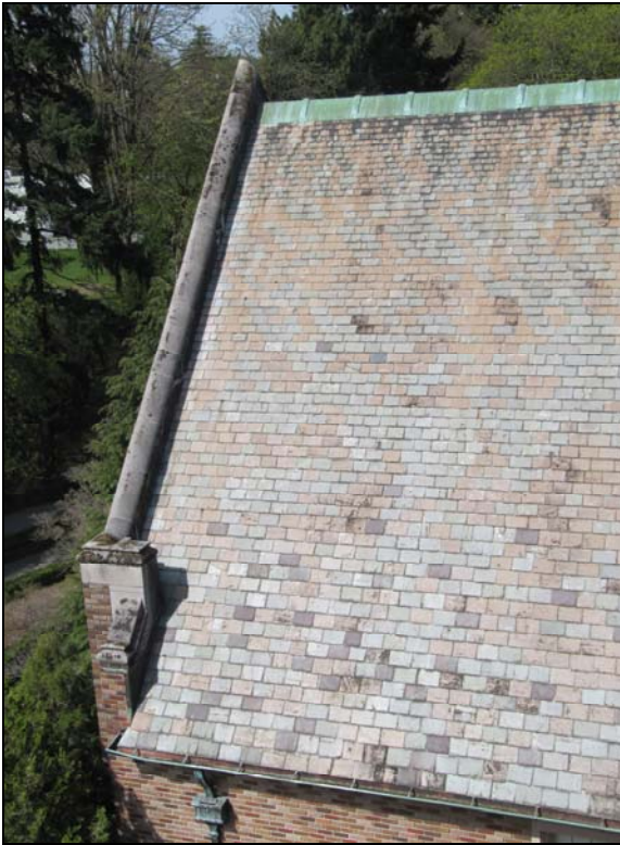
Above left, a view looking northwest at the south roof slope of the west wing of the building, showing the varied color, size and exposure of the original slates. Above right, views of two small slate-clad dormers on the back of the building, where the material was used for wall cladding as well as roofing. Note the copper gutters, downspouts, and scupper boxes in both views. Below, a detail view of the slate roofing near the small dormer.
