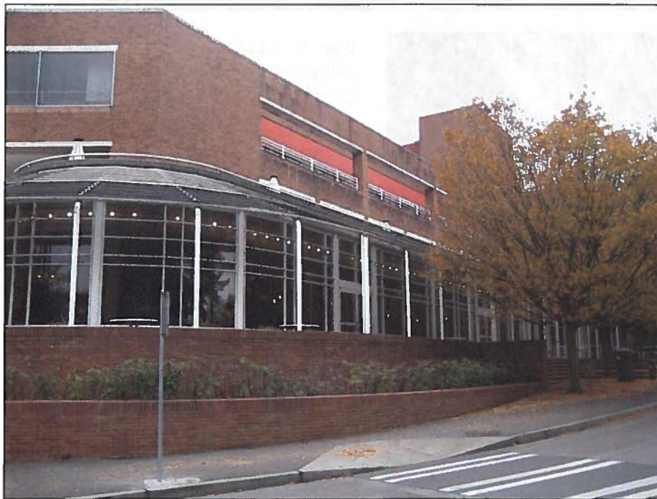
A closer view of the Husky Den at the southeast portion of the HUB.
