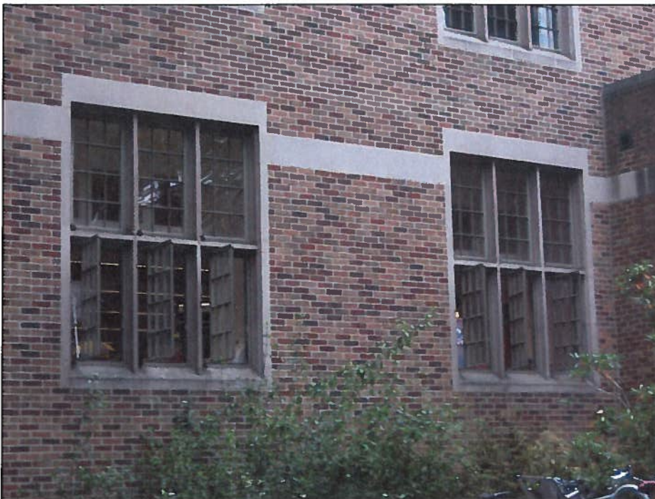
Detail view of window groupings on the north façade, 1949 wing.
