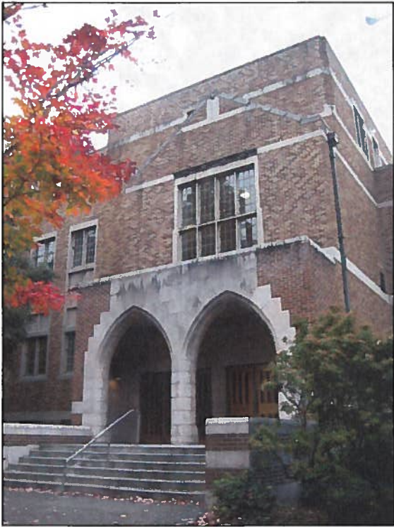
Left: View of the entry near the south end of the west façade, 1952 wing. This entrance was not original to the 1952 wing but was added ca. 1973 as a fire and life safety improvement.
