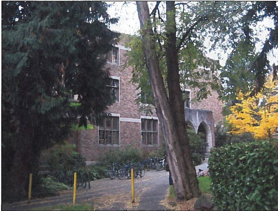
Looking southwest at the north end of the 1949 wing. The entry originally had a single arched opening but was widened in the mid-1970s fire and life safety improvements.
