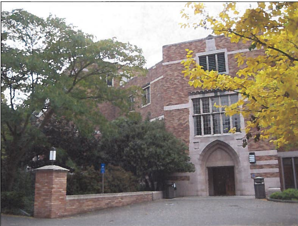
Below: Looking northeast at the entrance at the south end of the 1952 wing, where the building orientation turned diagonally.
