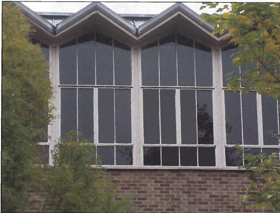
Detail view of the glazed wall and folded plate roof.
