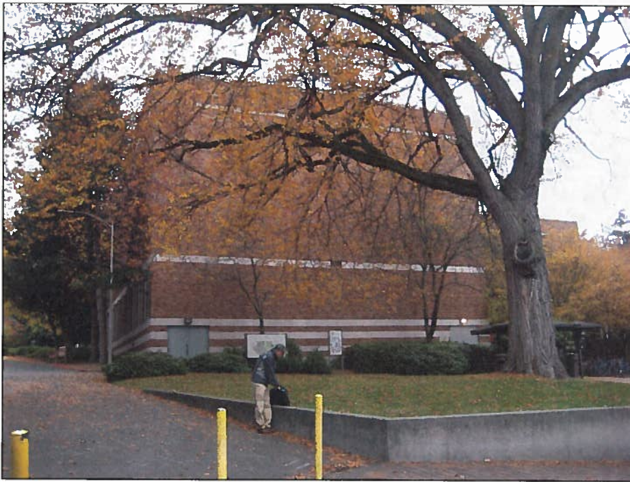
View looking northwest toward the southern end of the 1963 auditorium addition.
