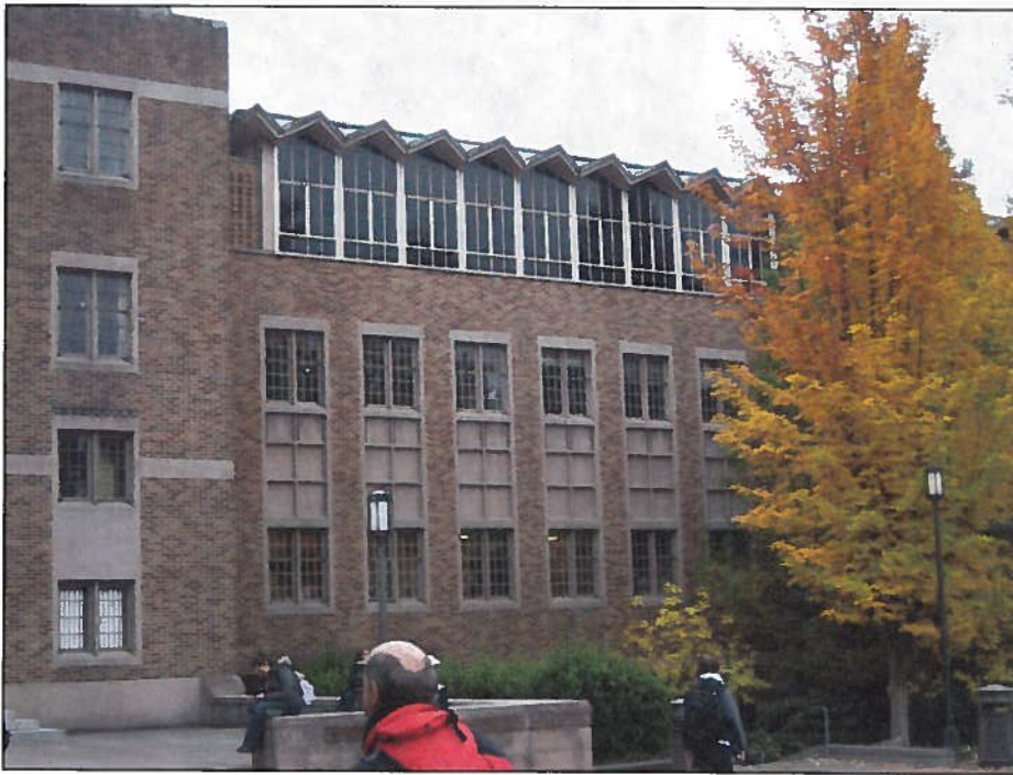
Looking southeast at the northern portion of the 1952 wing (two stories). The third story was enclosed in 1959 and capped with the folded plate roof.
