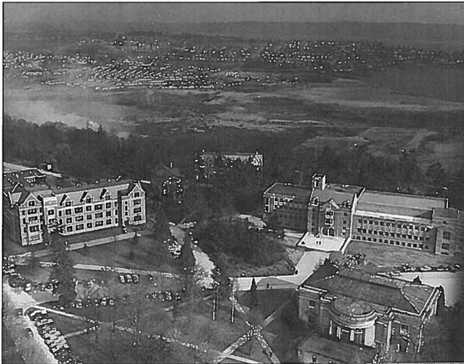
Aerial looking northeast over HUB Yard, 1955. This photograph shows lawn, criss-crossing paths, scattered trees—many of them volunteers, and vehicle parking in the HUB Yard area. The Washington State Museum is visible at the lower right, the HUB in the mid-ground center, and Thomson Hall at the far left. (UW Libraries Special Collections, neg. no. UW 19721z.)
