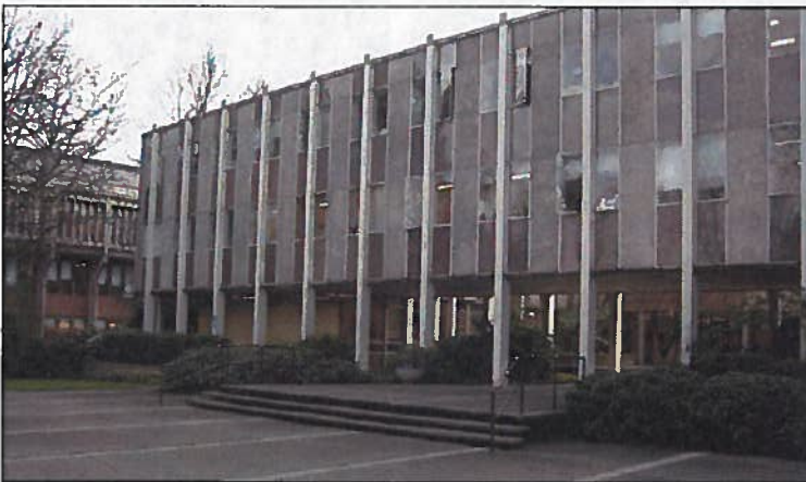
Left, oblique view of the north facade, MacKenzie Hall.
