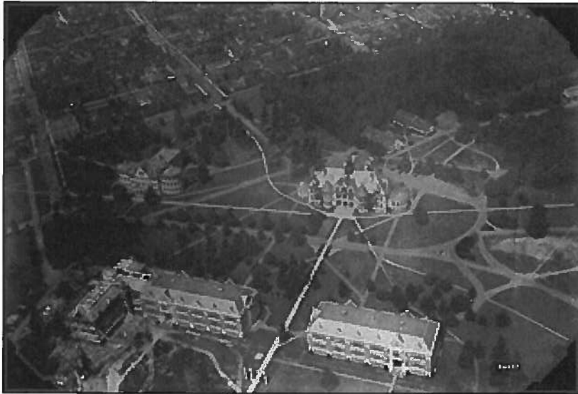
Above, an aerial view looking northwest at Denny Hall, in the center of the photo. To the far right of it the site of Hutchinson Hall remains open. The two gable roofed structures to the northwest of Denny appear to be temporary buildings, perhaps constructed during World War II. The two buildings near the bottom of the photo are Savery and Raitt Halls, which form the west edge of the Liberal Arts Quad. (University of Washington Special Collections)
