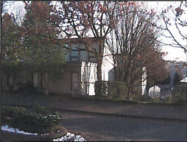
Figure 15 • Ethnic Cultural Center viewing south along western facade
