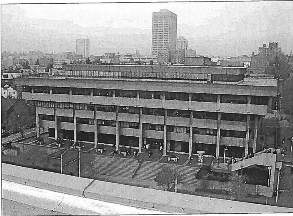
View of Schmitz Hall looking northwest from the roof of the Duchess across the street, November 2004. It is more evident in this image the way the upper stories of the building project over the plaza. The penthouse is also visible here.
