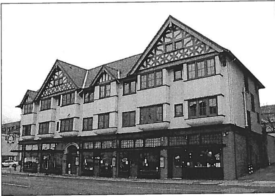
College Inn, view from southeast, October 2004. Clearly visible in this image is the decorative half-timbering in the gable ends, so characteristic of Tudor Revival buildings. The relatively low scale and nice rhythm of the structure, as well as the expanse of invitingly glazed ground-floor commercial spaces, make a positive contribution to the neighborhood and pedestrians who pass the College Inn.
