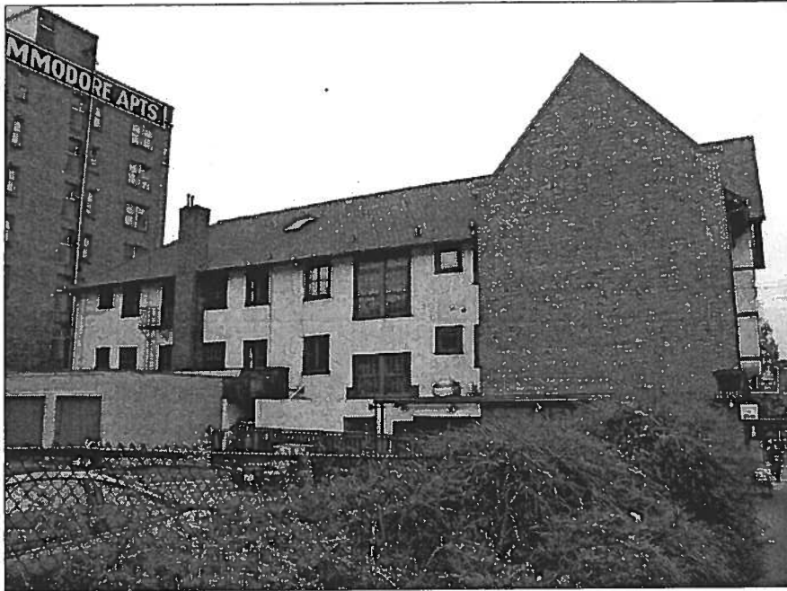
College Inn, north elevation, October 2004. The brick expanse that now presents a solid face would have served as a fire resistant break when there was a building immediately to the north. Although it no longer serves its original purpose, the wall harmonizes with the use of brick masonry in the University District and on the University campus.
