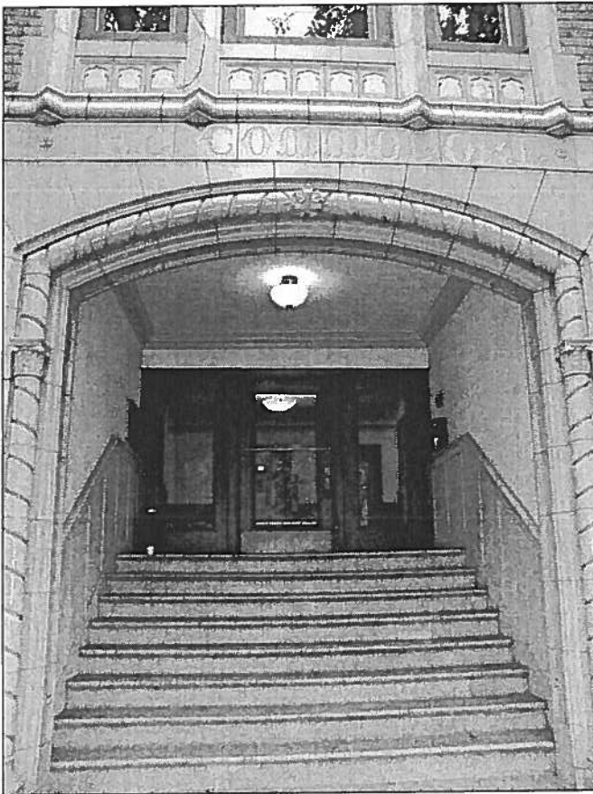
Original entry of Commodore showing terra cotta surround and decorative detailing, October 2004.
