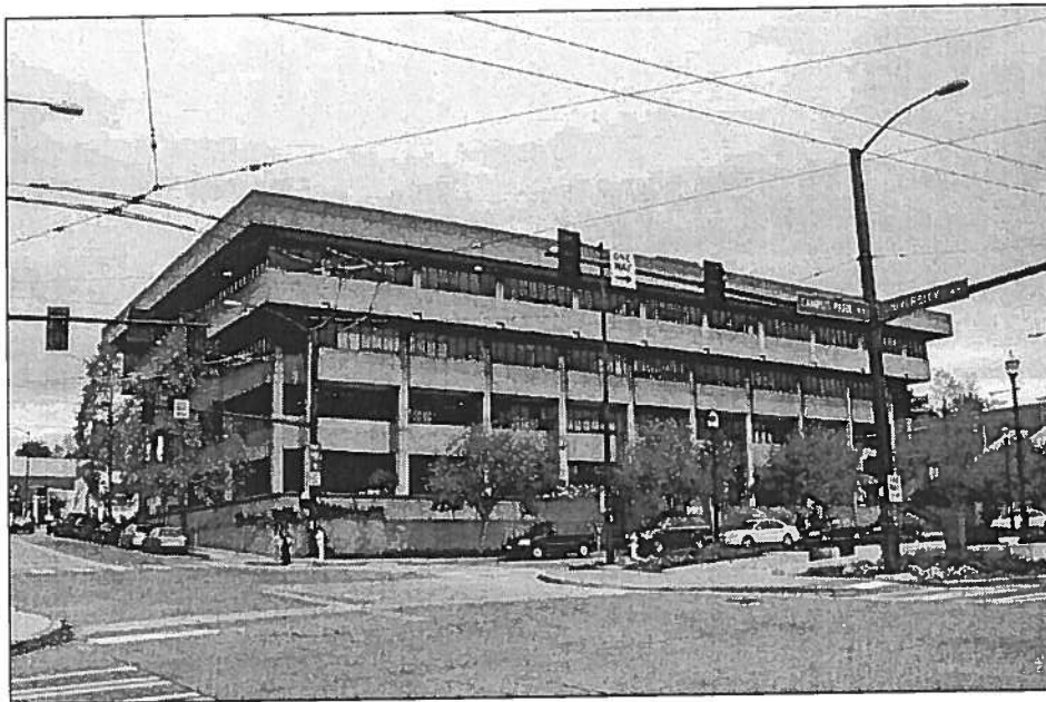
Schmitz Hall, view from southwest, October 2004.
