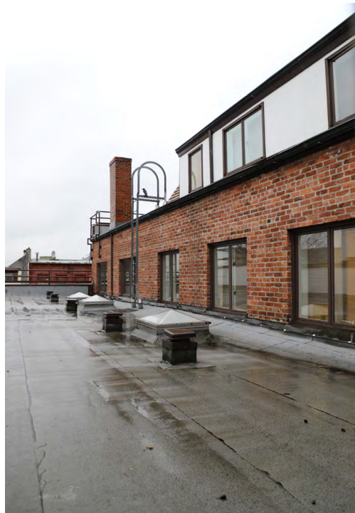
Figure 40. Roof over the southwest portion looking west along the back side of the north ell.
