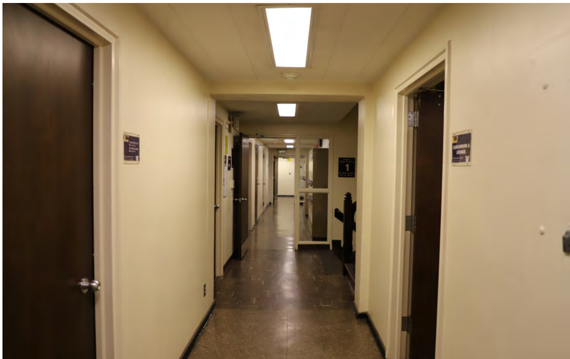
Figure 42. First floor, north ell looking east along the corridor.
