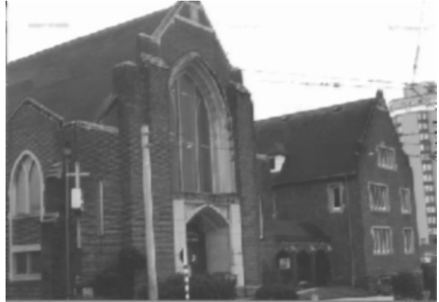
Figure 74. University Baptist (now Cross & Crown Church), 4554 12th Ave NE, designed by Schack, Young and Myers, built by Daniels & Turnquist, 1925.
