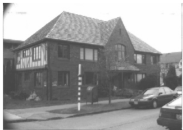
Figure 70. 711 NE 43rd St, designed by Frederick Anhalt, 1928.
