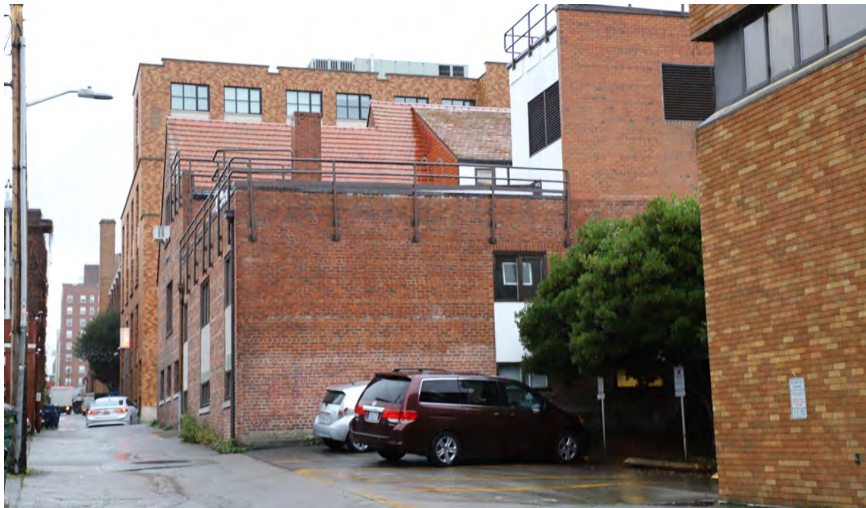
Figure 33. Southwest corner looking north.
