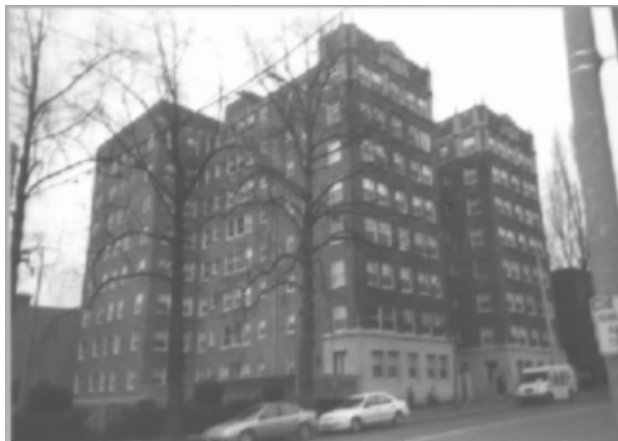
Figure 66. Malloy, 4337 15th Ave NE, designed by Earl Roberts, 1928.
