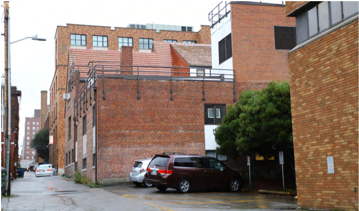
Figure 33. Southwest corner looking north.
