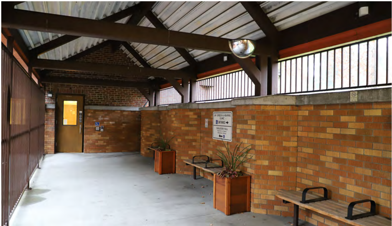
Figure 28. Covered breezeway connection on the south facade, looking north towards the building.
