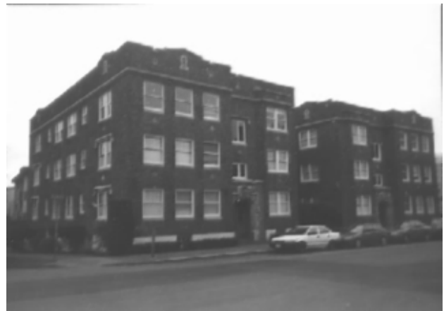
Figure 69. Roberta and Carol Apartments, 1115 & 1119 NE 43rd St, designed by E.C. Rising, 1929.
