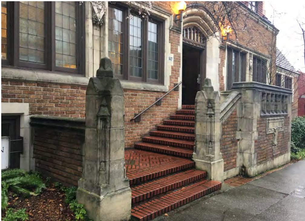
Figure 37. Main north entrance looking southwest.
