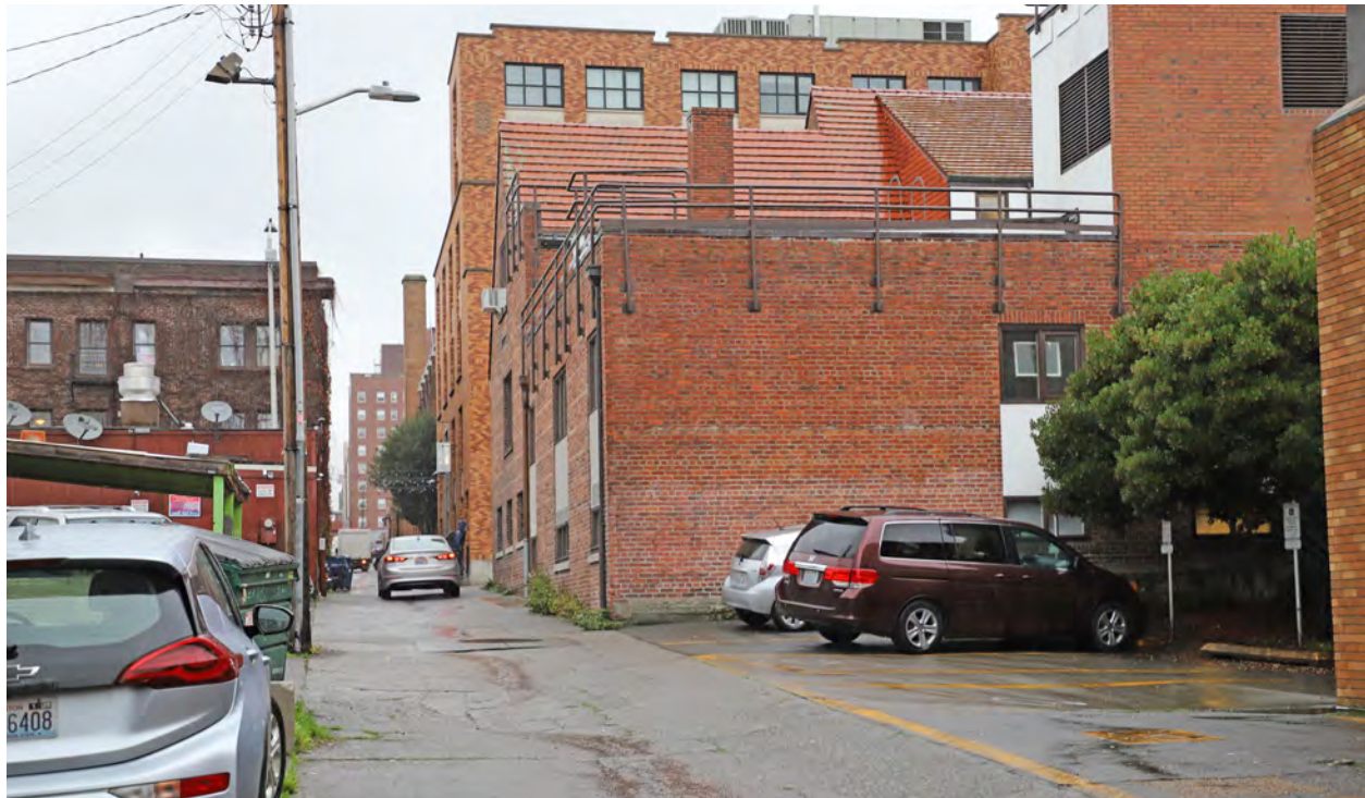
Figure 96. Vicinity, looking north along the alley.
