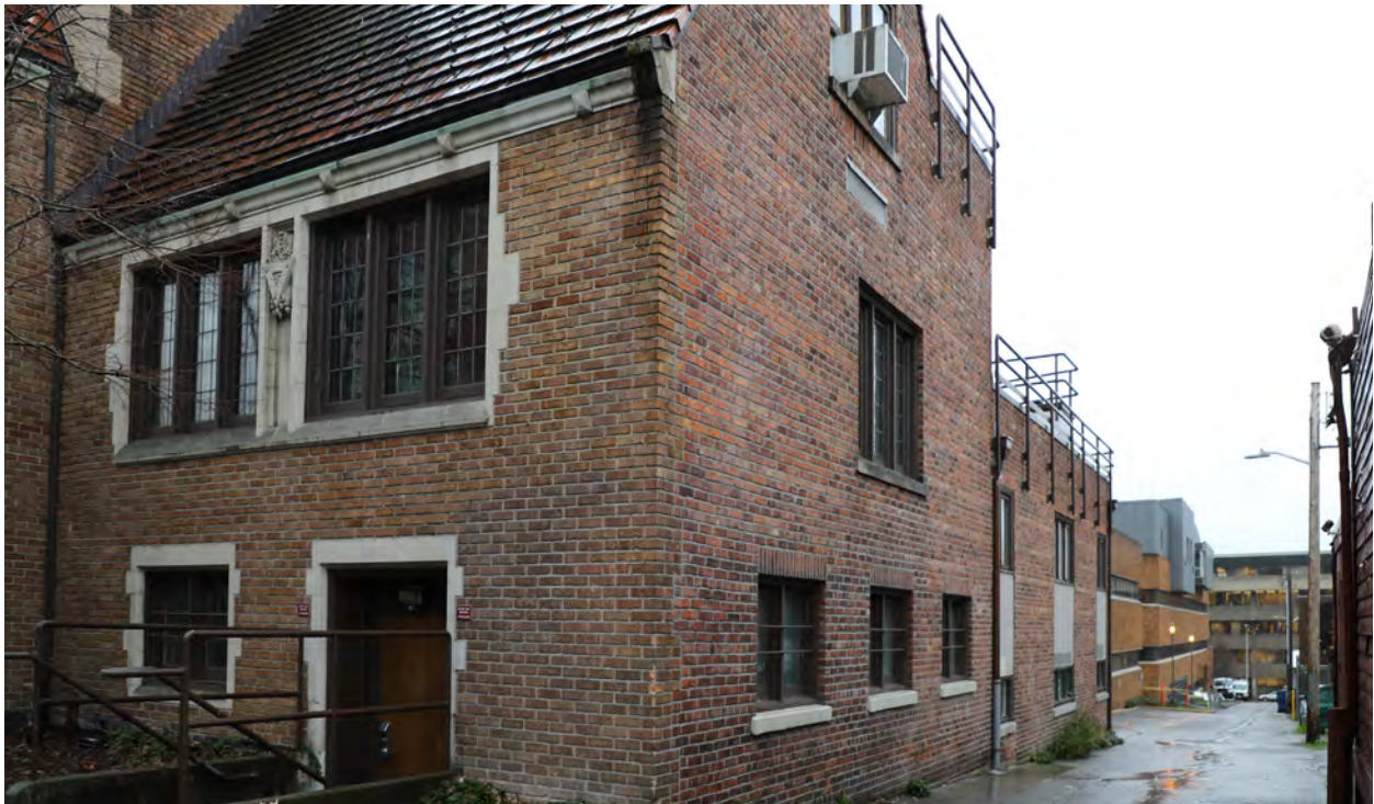
Figure 29. Northwest corner looking south along the alley.
