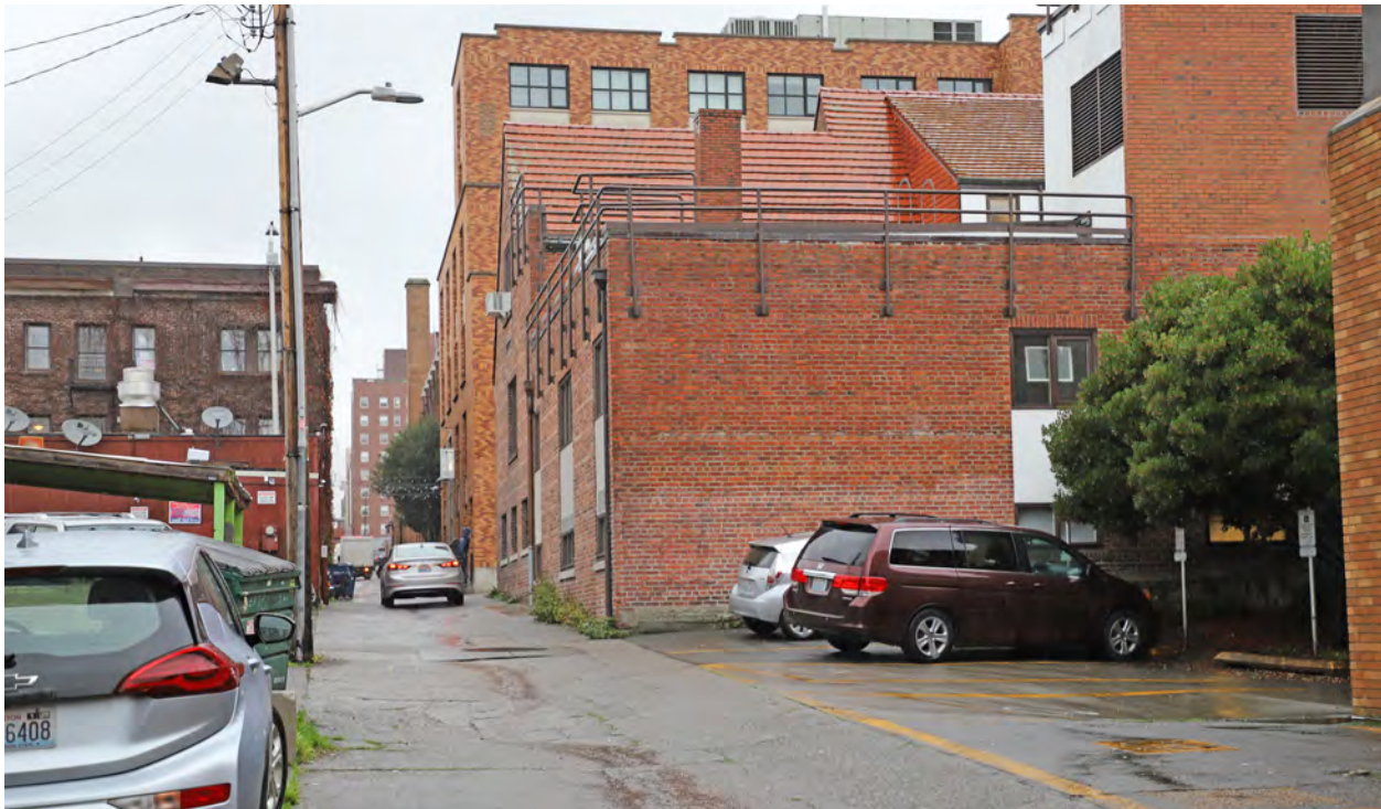
Figure 96. Vicinity, looking north along the alley.
