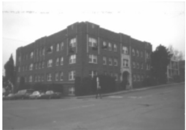
Figure 68. Gellesley Apartments, 4203 Brooklyn Ave NE, 1925.
