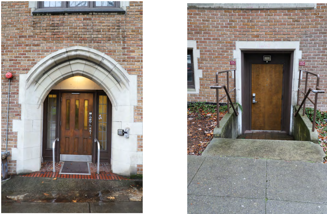
Figure 36. East entrance (left) and north first floor entrance (right).
