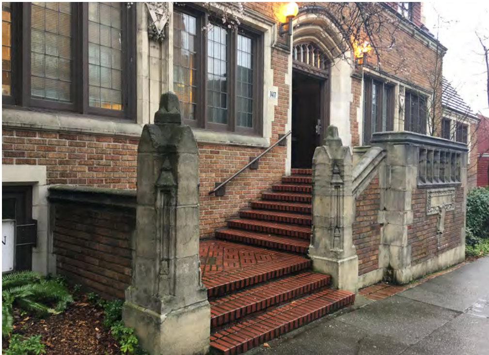
Figure 37. Main north entrance looking southwest.
