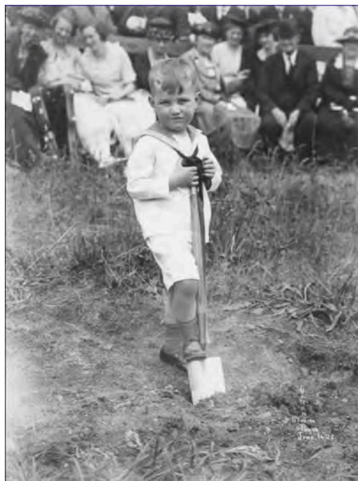
Figure 19. Groundbreaking ceremony for Eagleson Hall showing the son of James M. Eagleson with spade, University of Washington campus, June 1922. Cowhn Studio. University of Washington Libraries, Special Collections, Order No. UW37703.
