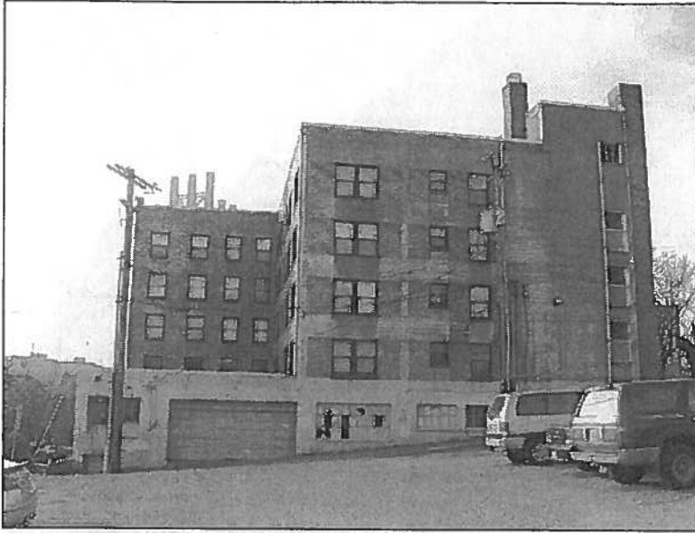
Cavalier Apartments, 1309 NE Campus Parkway, East Elevation
