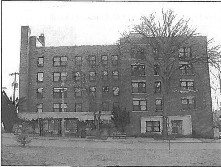
Cavalier Apartments, 1309 NE Campus Parkway, North Elevation
