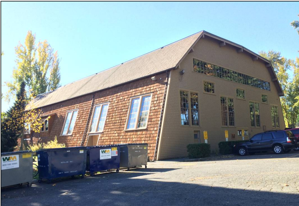
Figure 13. Looking southwest toward the north and east façades.
