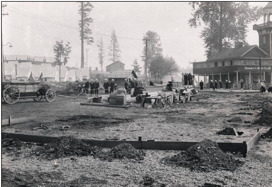
Figure 28. Construction site at U.S. Naval Training Station on the south end of the UW campus, 1917-18. (MOHAI image no. 1993.35.1.16)
