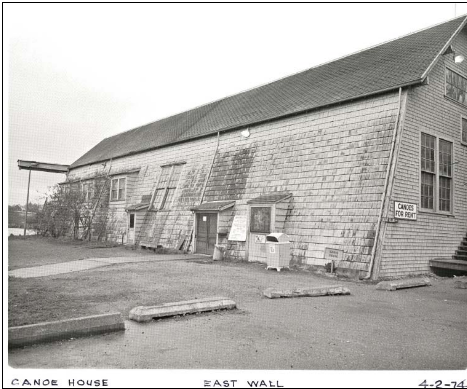
Figure 7. View looking southwest along the east side. (UW Facilities Records)
