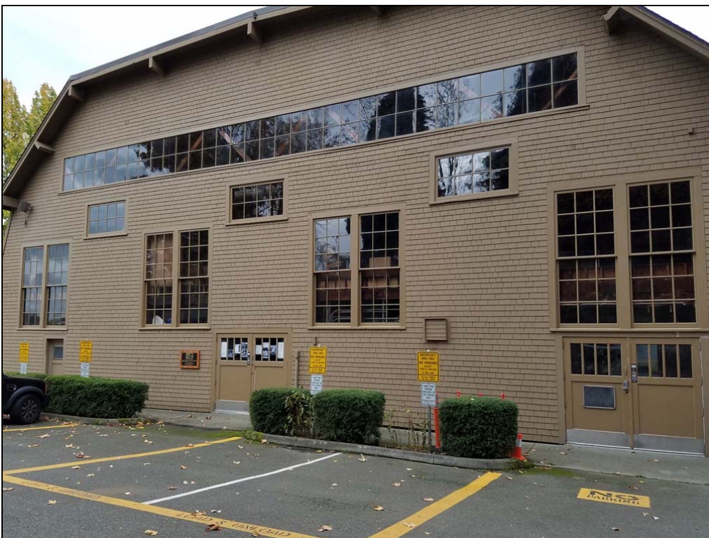
Figure 14. View of the north façade. (Courtesy University of Washington)
