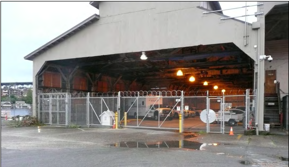
Figure 17. Below, view looking west at the interior space in Building D.
