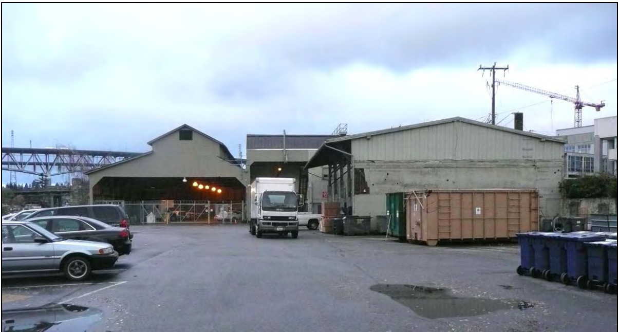
Figure 15. Below, view looking west at the east facades of Buildings D (to the left), and G (right), and a portion of Building B between them.
