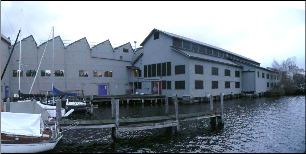
Figure 20. Above, view looking northeast at the south facades of Buildings D (with saw tooth roof) and an oblique view of the south and west facades of Building B.
