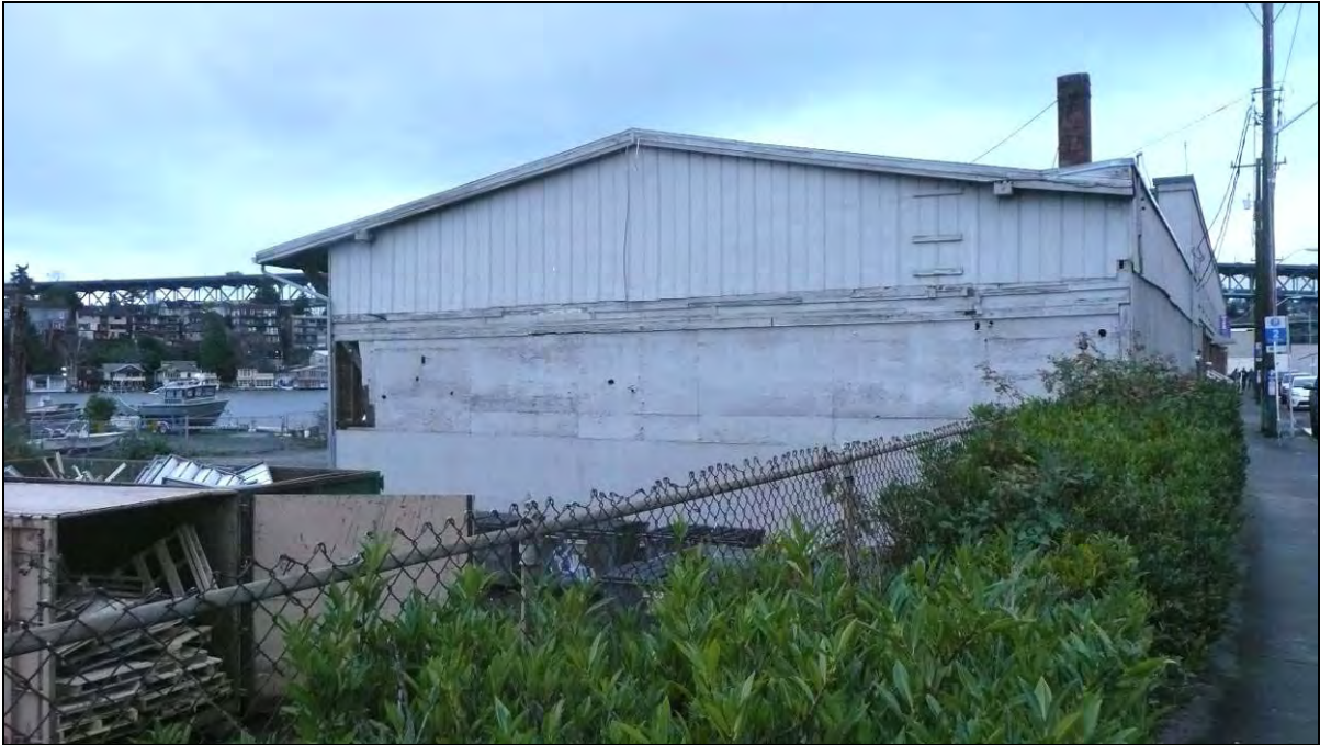
Figure 14. Above, view looking southwest at the east facade of Building G and a portion of Portage Bay beyond.
