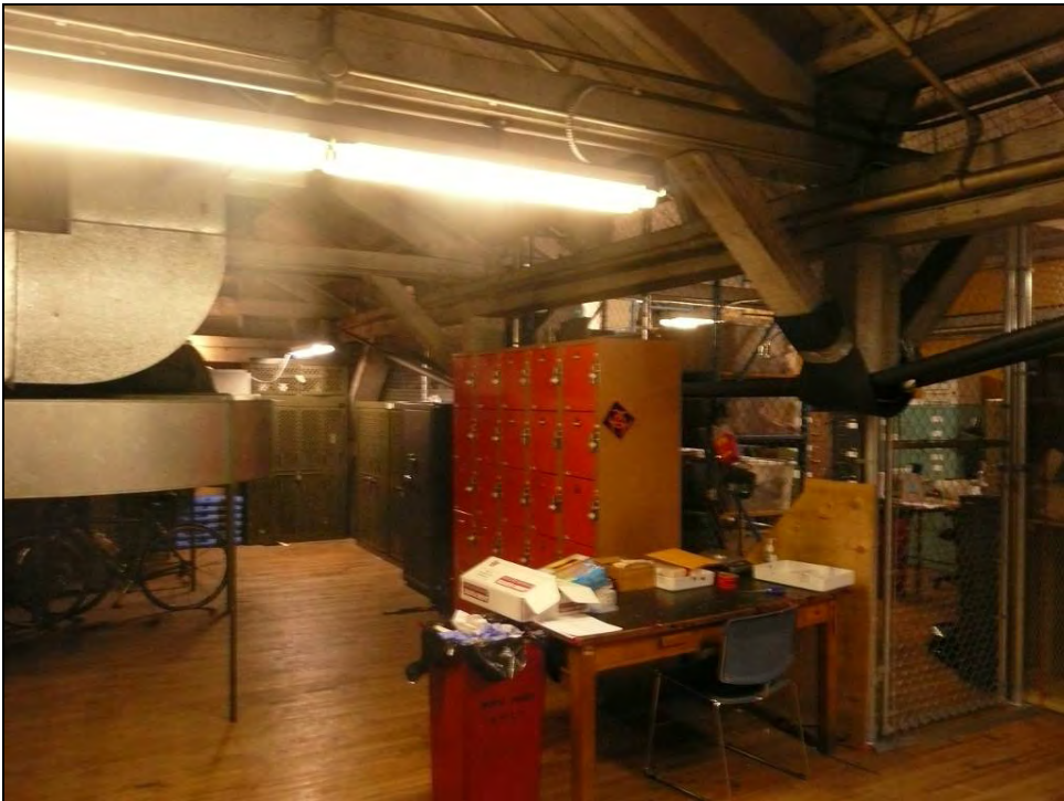
Figures 28 – 29. Above, view of a conference and meeting room in Building B. Below, view of a typical upper floor storage and locker room space in this building. Heavy timber framing and mechanical ductwork are typically exposed. Finishes, fixtures, partitions and mechanical/electrical system elements are non-original.
