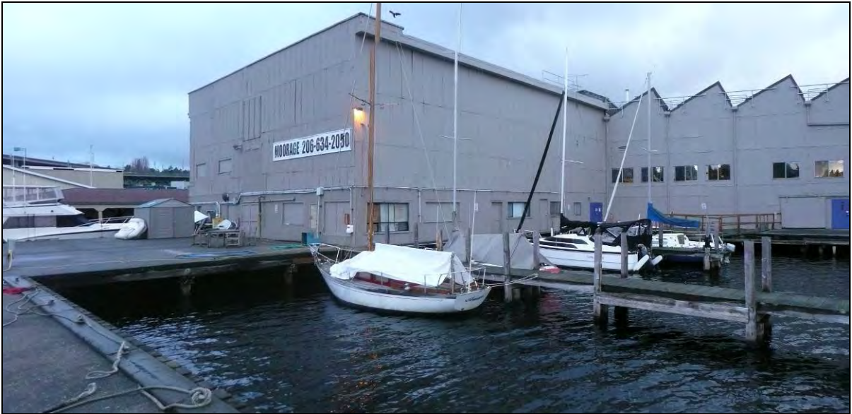
Figure 21. Below, a view looking northwest at the south and east facades of building C and a portion of Building B. These views also show the current marina docks.
