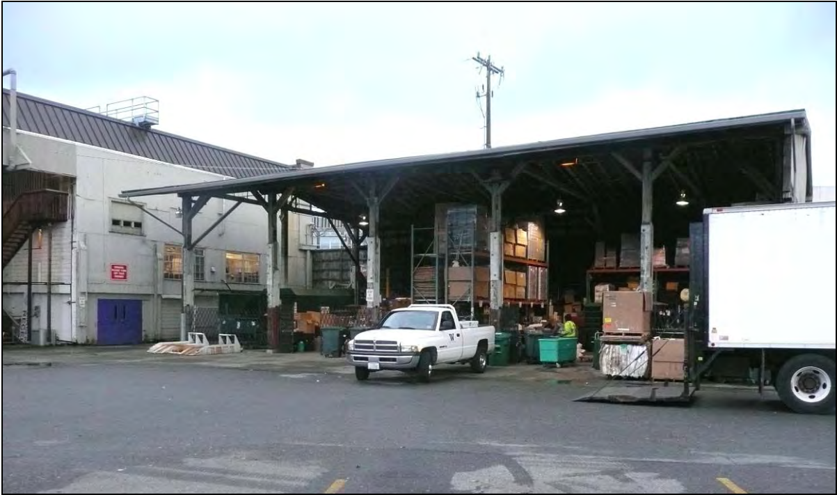
Figure 16. Above, view looking northwest at the south opening on the south side of Building G, showing the heavy timber framing and covered interior space.
