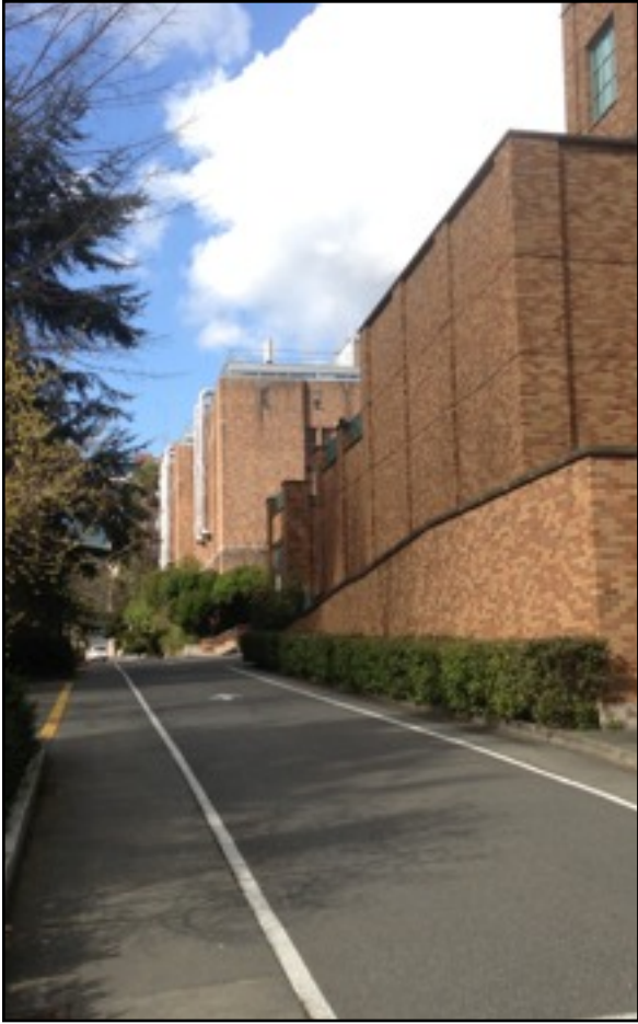
Existing view from Okanogan
