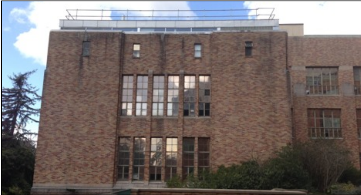
View of typical existing west wing parapet wall condition
