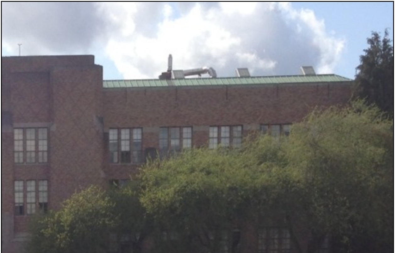
Viewing roof monitors and mechanical equipment located on the northern end of the east wing
