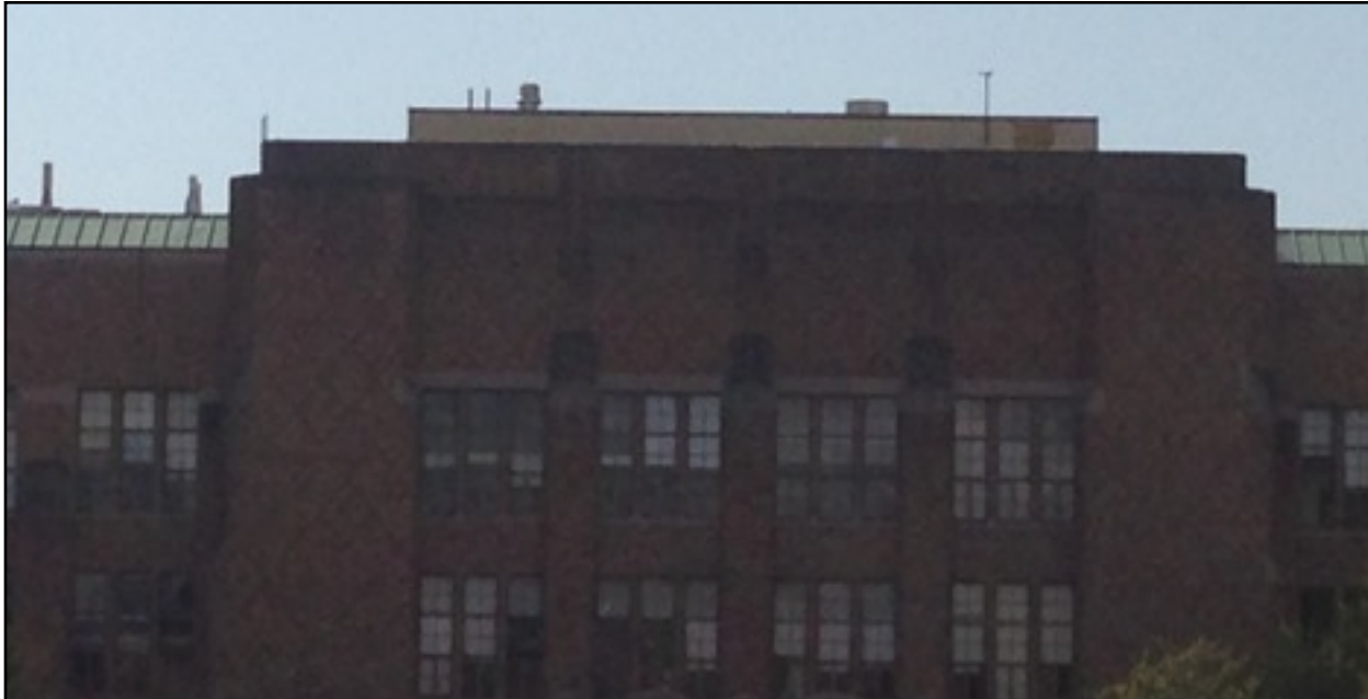
View of existing east wing penthouse from across Rainier Vista
