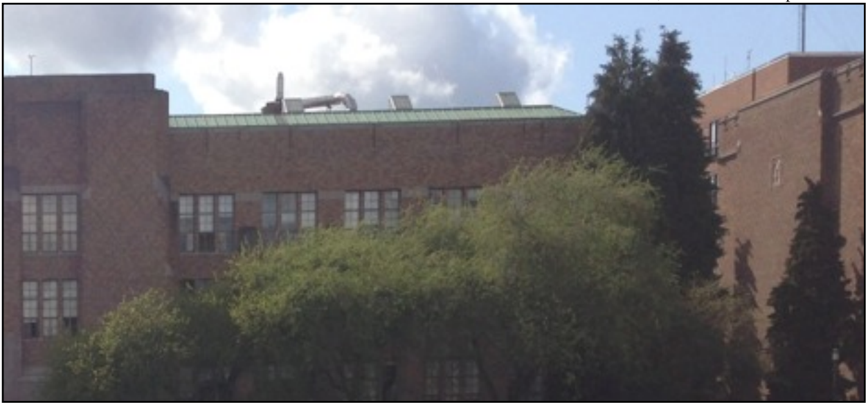
View of existing roof monitors and mechanical equipment from Drumheller Fountain
