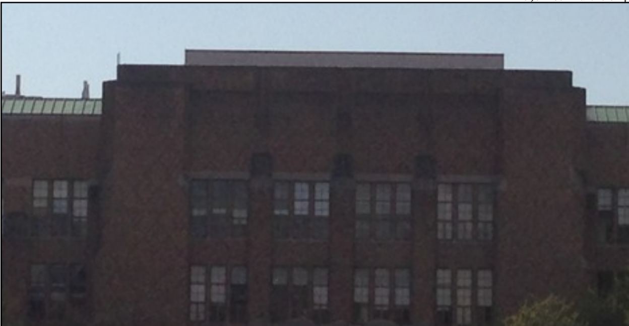
View of proposed changes to east wing penthouse from across Rainier Vista
