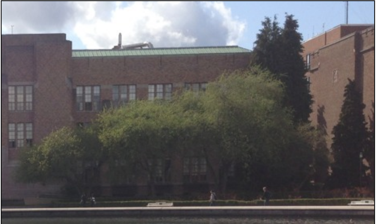
View of proposed copper gutter and mansard roof condition from Drumheller Fountain - after patina or green metal.
