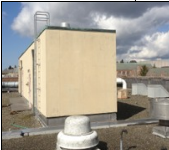
Viewing penthouse from east wing roof
