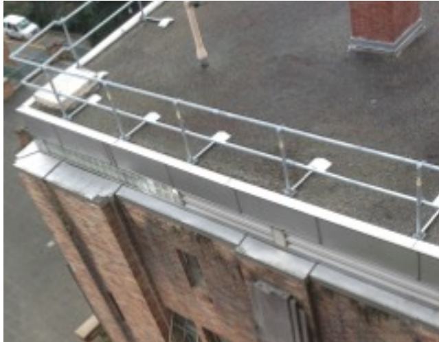
Detail of 1951 parapet wall at west wing
