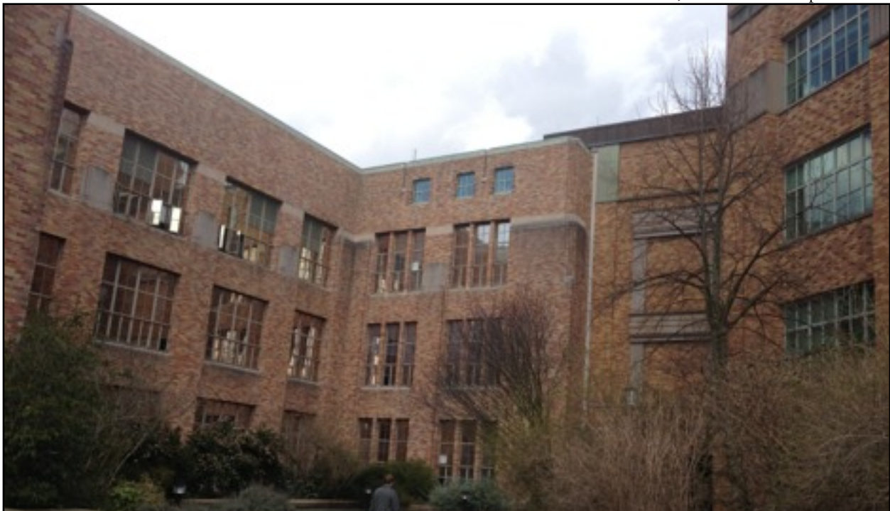
Viewing the eastern portion of the southern façade from the pedestrian plaza
