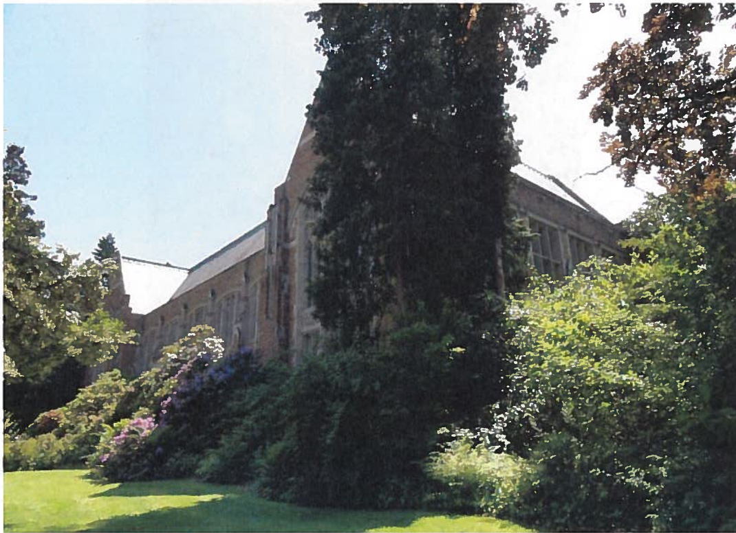
Figure 13: Exterior Photograph- Anderson Hall North and West Sides, 2011
