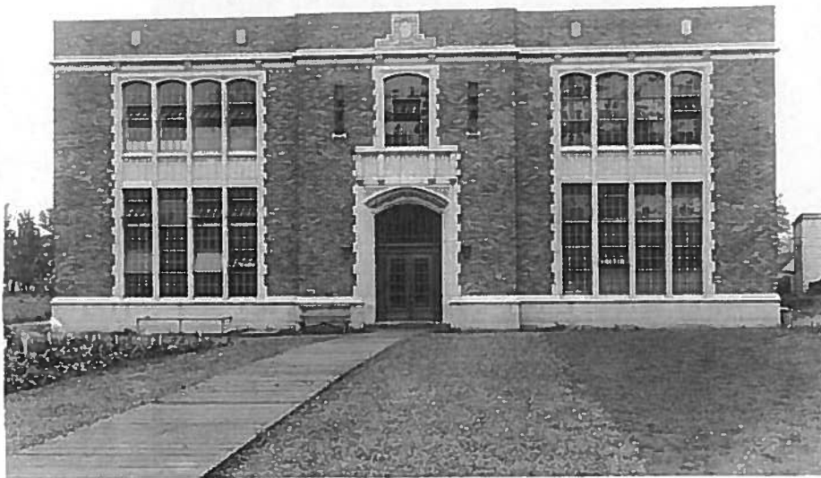
Figure 9: Historic Exterior Photograph- North façade of the Forest Products Laboratory, no date Photo property of MSCUA, University of Washington Libraries
