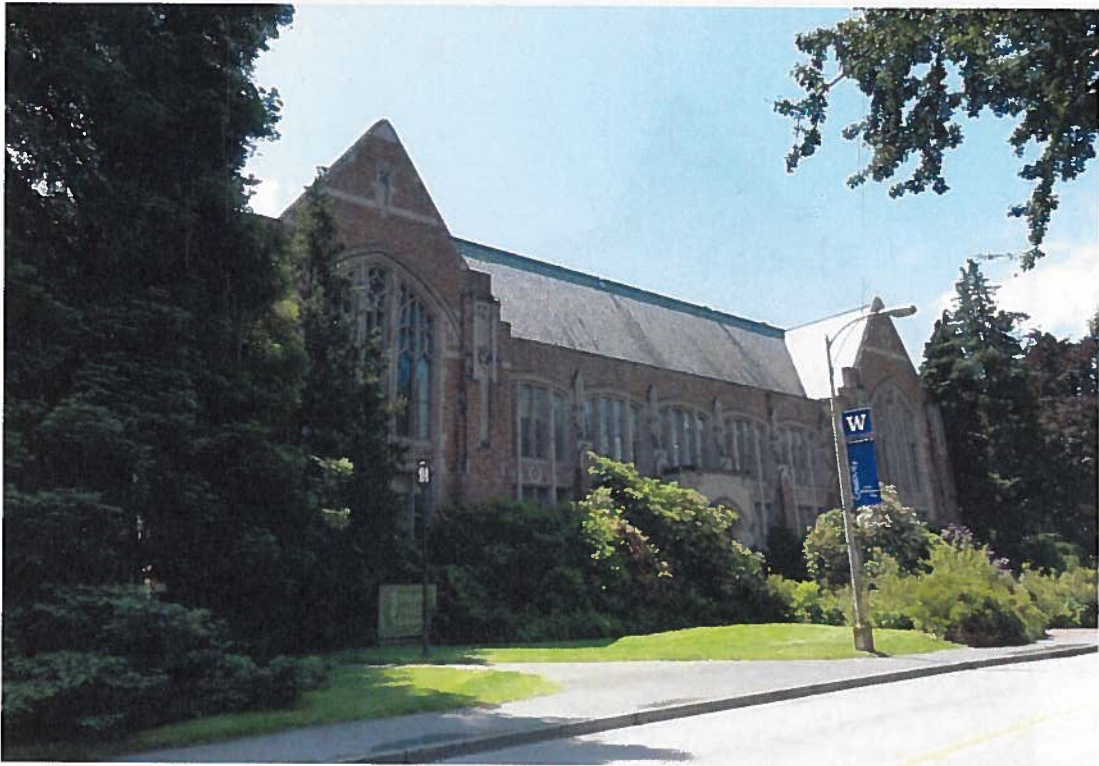
Figure 10: Exterior Photograph- Anderson Hall North façade, 2011
