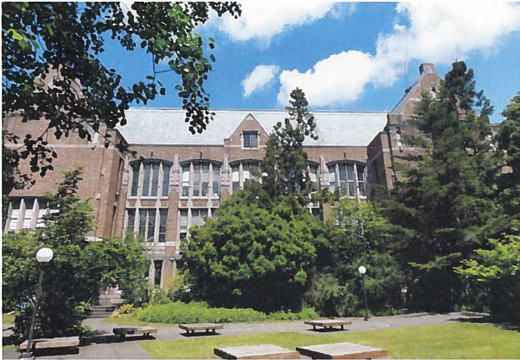
Figure 12: Exterior Photograph- Anderson Hall South Façade, 2011
