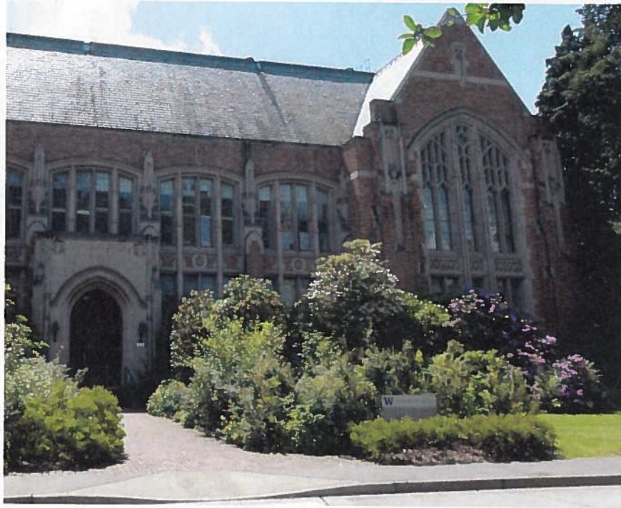
Figure 14: Exterior Photograph- Anderson Hall North-side Details, 2011
