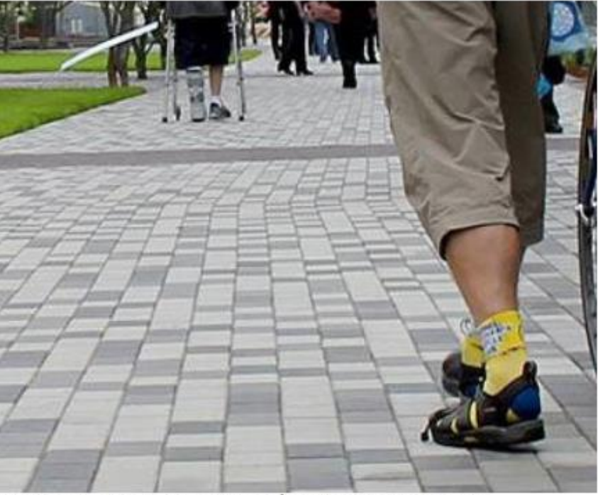
terrace placemaking | sandset pavers
