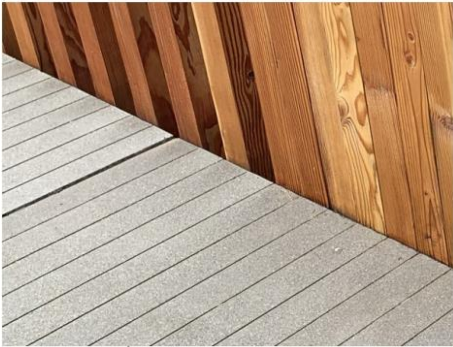
entry bridge | light touch planking
