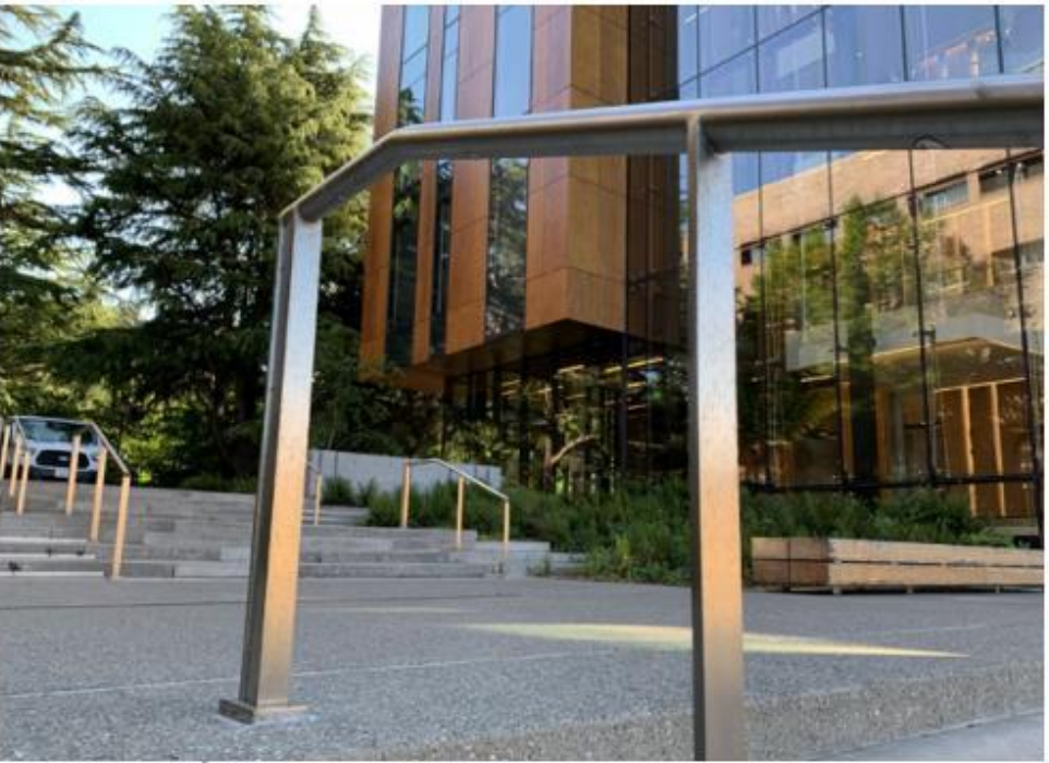
handrails | clean detailing
