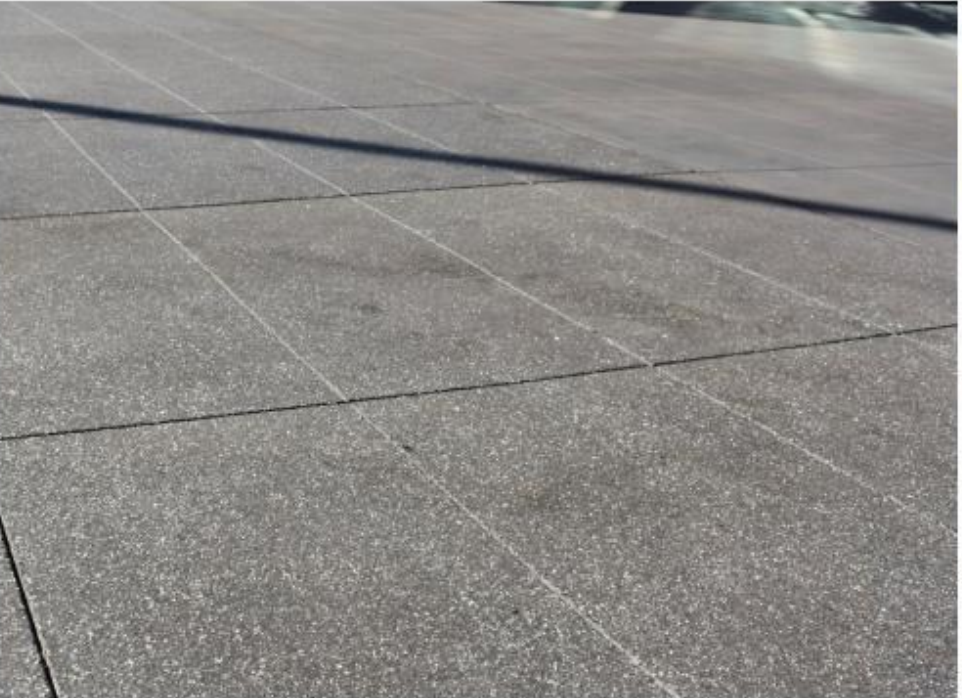
gathering plaza | accent finished concrete
