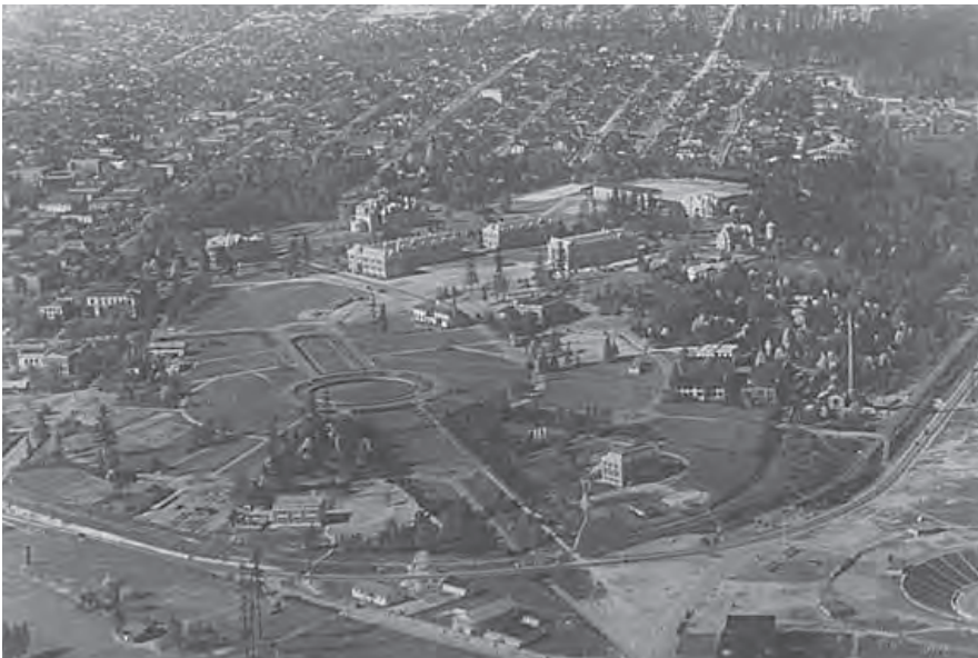
Mines Building First Phase, 1923
