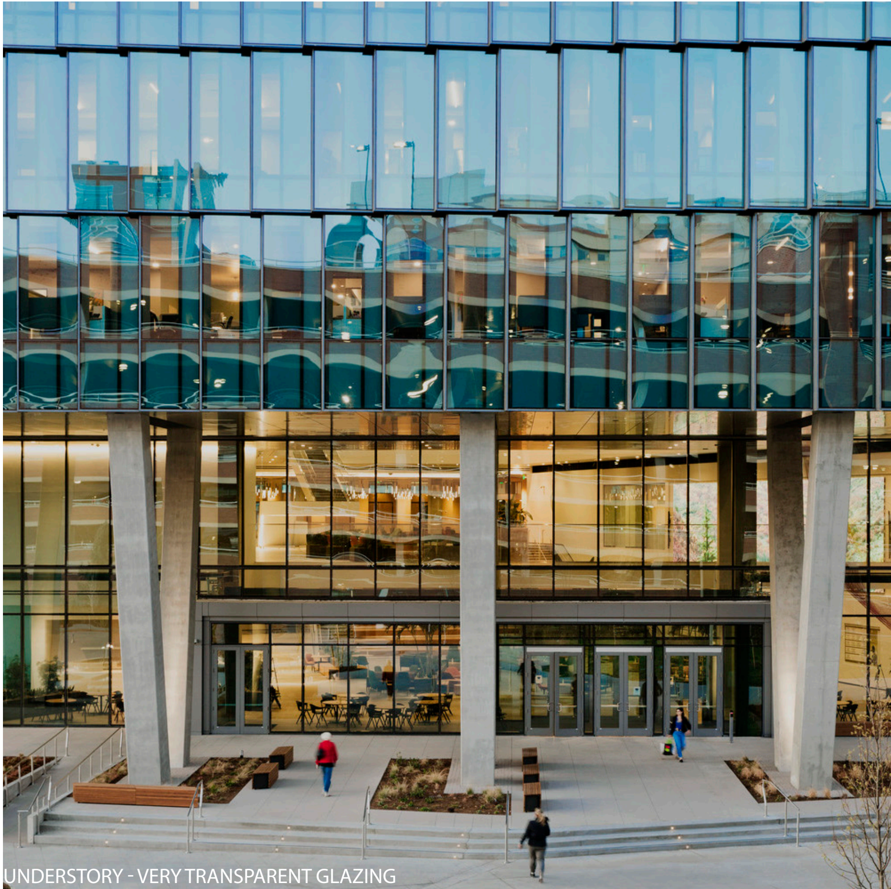
PIERS - BOARDFORM CONCRETE
