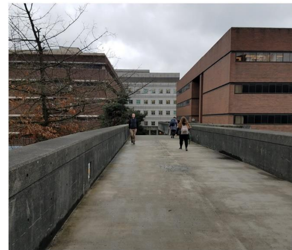
Pedestrian bridge crossing Pacific
