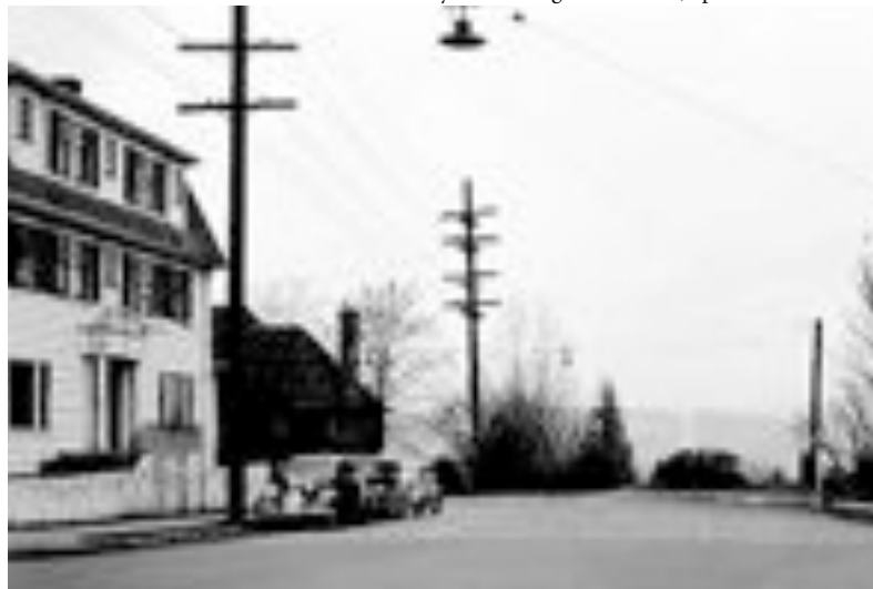
Subject building in 1938 just before the viaduct was started.
