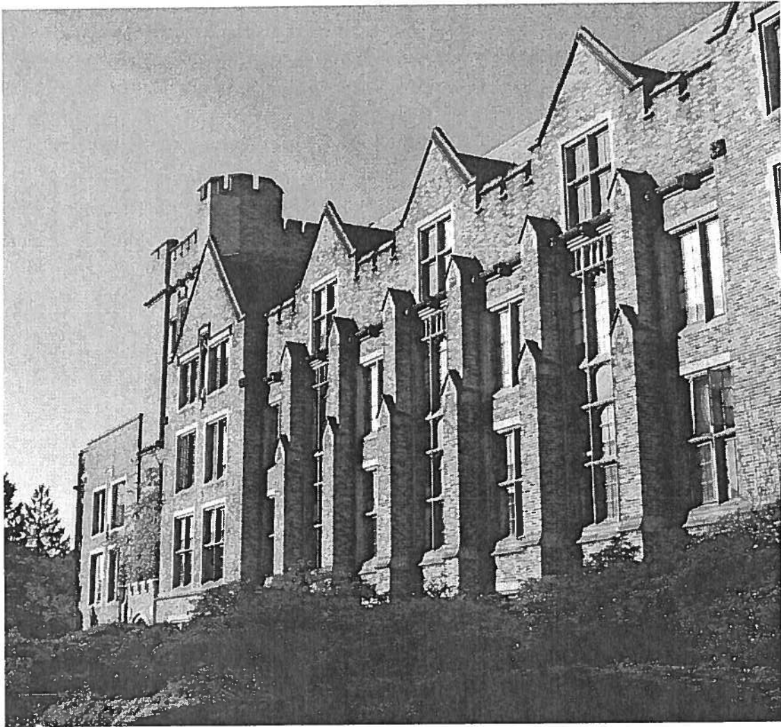
Johnson Hall East Elevation, September 2001
