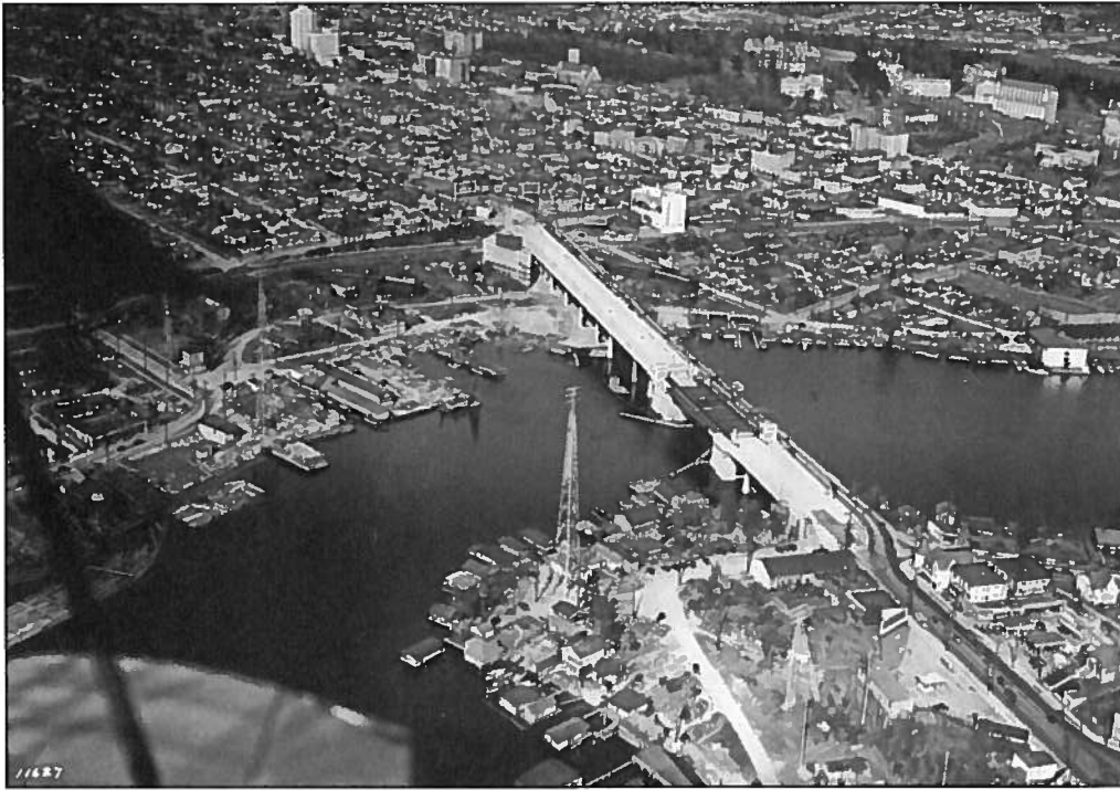
Above, an aerial view of the 1932 University Bridge construction and the north shore of Lake Union and Portage Bay.
