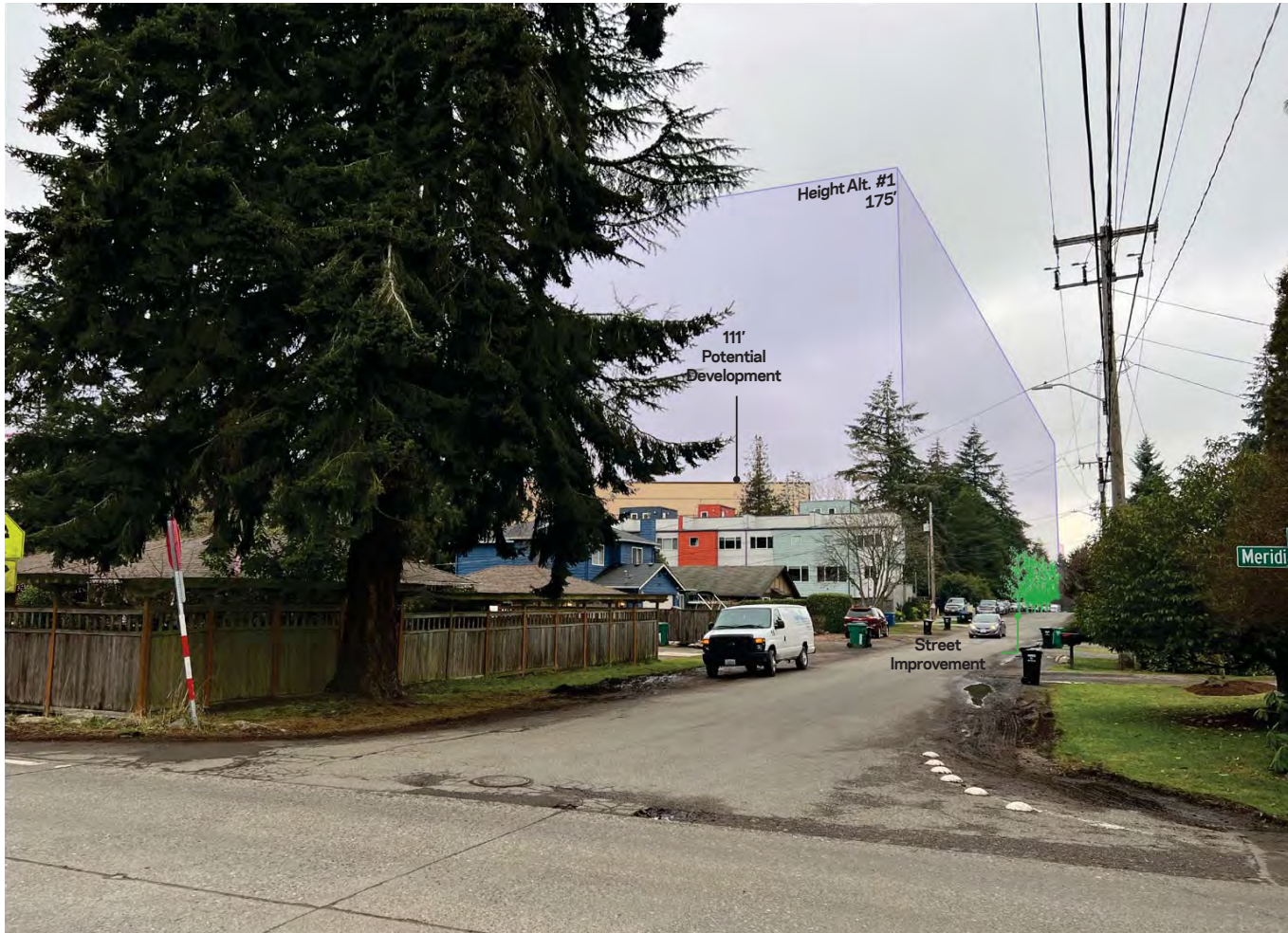
175' HEIGHT OVERLAY @ 30' SETBACK FROM PROPERTY LINE; @ 400' FROM CAMERA POTENTIAL DEVELOPMENT ALMOST 940' FROM CAMERA
