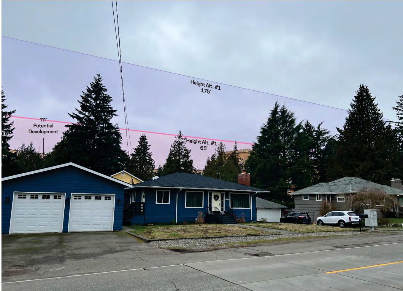
65' HEIGHT OVERLAY @ 40' SETBACK FROM PROPERTY LINE, @ 250' FROM CAMERA 175' HEIGHT OVERLAY @ 370' FROM CAMERA (APPROX. 160' FROM PROPERTY LINE) POTENTIAL DEVELOPMENT ALMOST 690' FROM CAMERA
