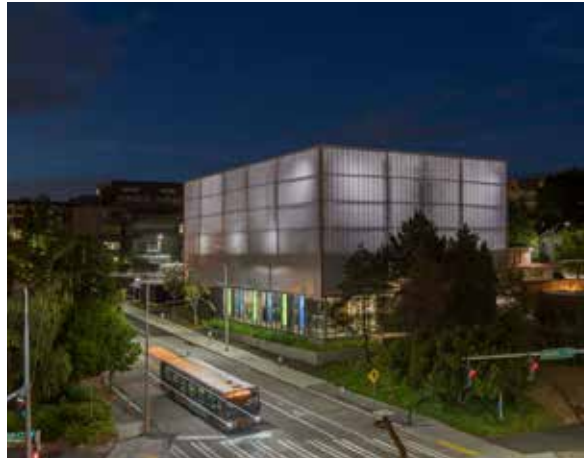
West Campus Utility Plant
