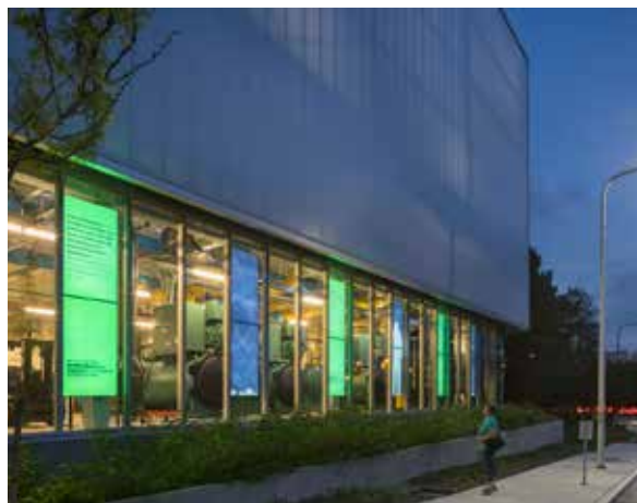
West Campus Utility Plant
