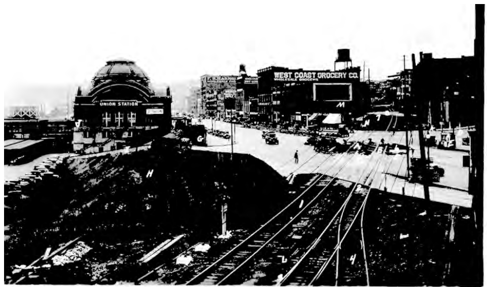
1929 Rail Book #2, No. 11-133 showing a view along the Prairie Line at the Pacific Avenue crossing. Photograph courtesy of Jim Frederickson.
