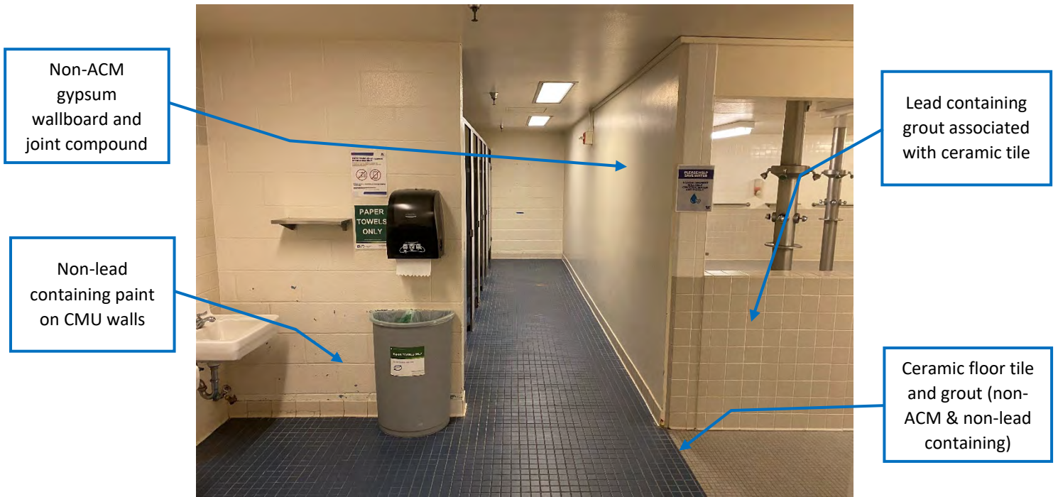
Photo 1: Women's Locker Room Restroom.
