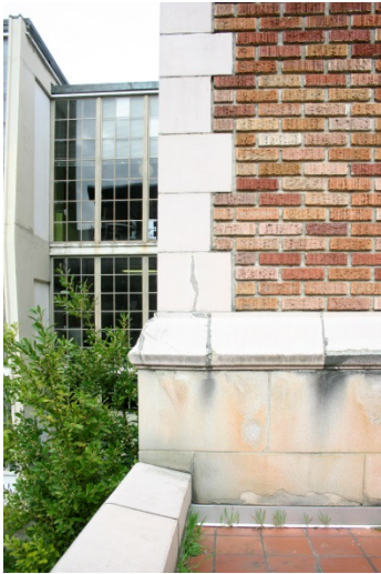
Intersection of pump room parapet and 1920 Laboratory Building – Current Condition
