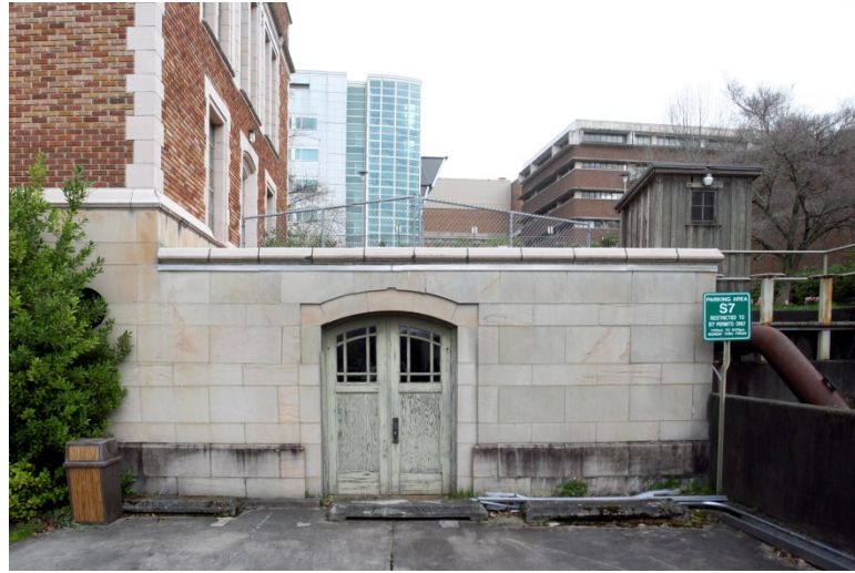
Pump Room, South Facade – Current Condition
