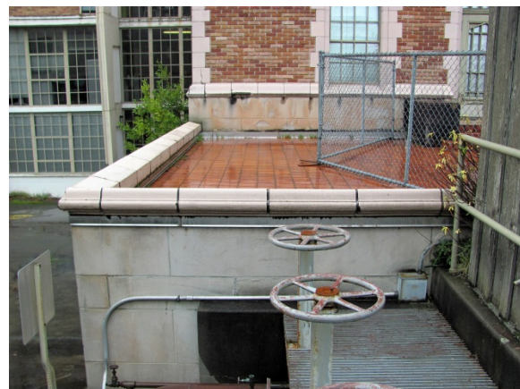
Patio above pump room viewed from the east – Current Condition
