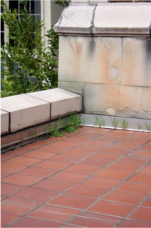
Southwest corner of patio – Current Condition
