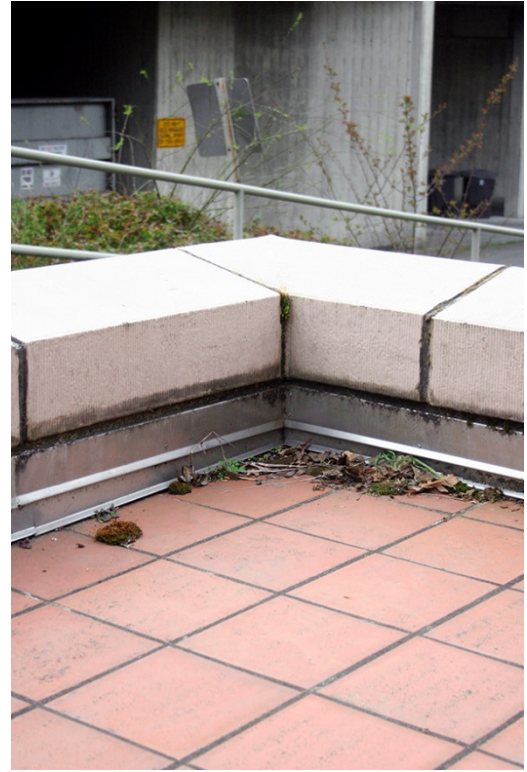
Southeast corner of patio – Current Condition
