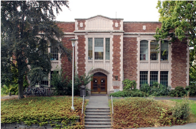
1920 Building, Northeast Façade – Current Condition
