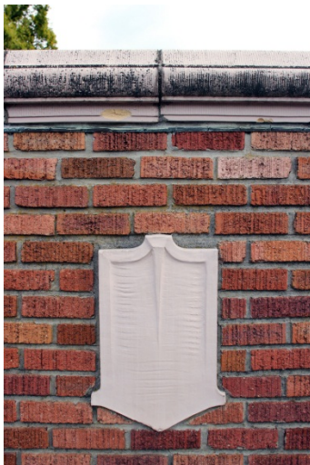
Detail on parapet of 1920 building
