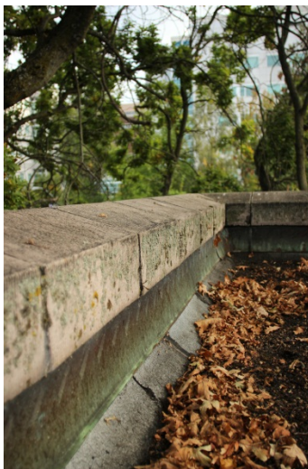
1920 Parapet – Current Condition
