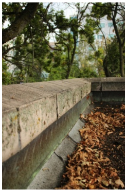
1920 Parapet – Current Condition
