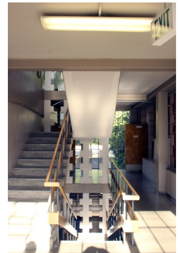
1961 Connector, Interior Stair Current Condition
