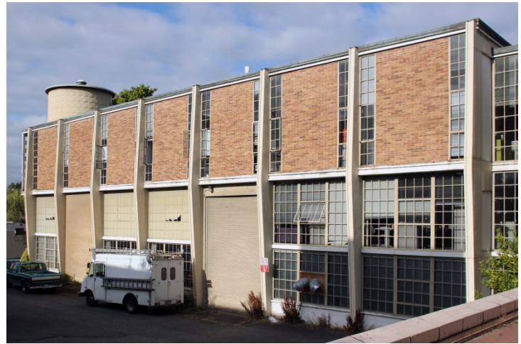
1961 Addition, Southeast Façade – Current Condition
