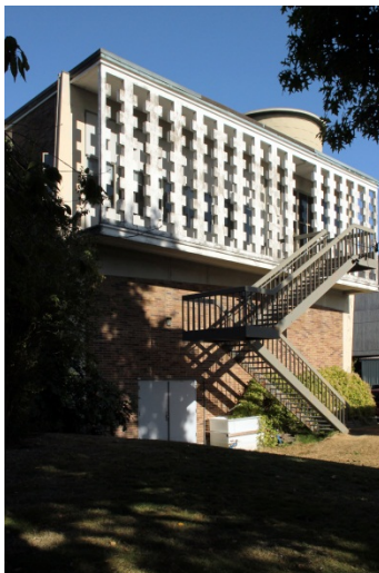
1961 Addition, Southwest Façade - Current Condition
