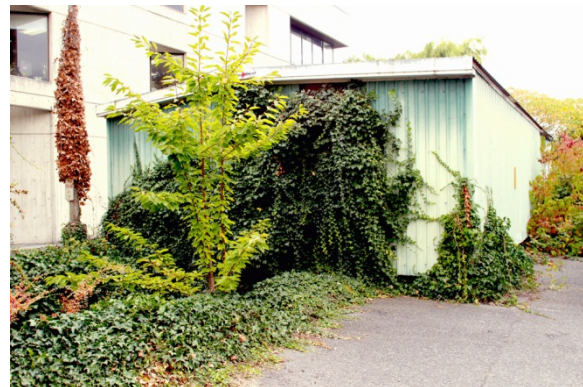
Mossyrock Dam Model Shed Current Condition
