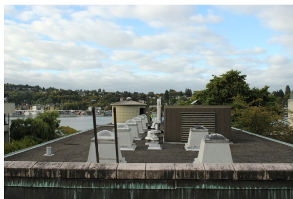
1961 Roof – Current Condition the 1920 Parapet is visible in the foreground
