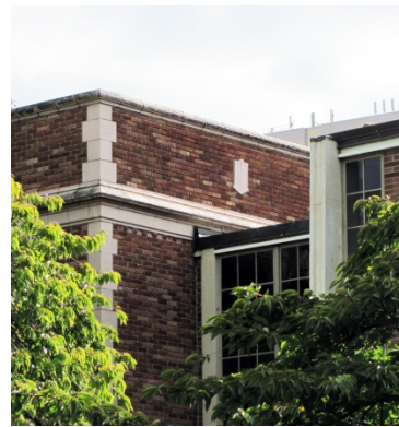
Detail of three roofs at connector Current Condition
