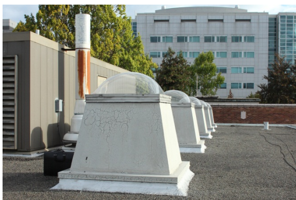
1961 Skylights – Current Condition
