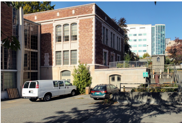
1920 Building, Southwest Façade – Current Condition
