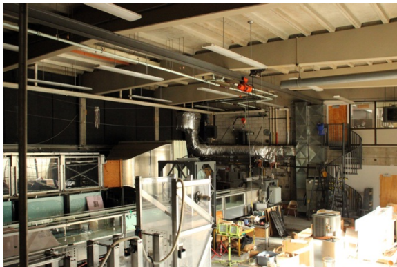
Interior of Harris Lab, lower level addition Current Condition
