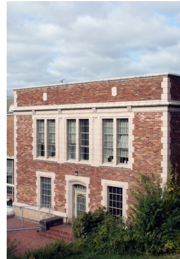
1920 Building, Northwest Façade – Current Condition
