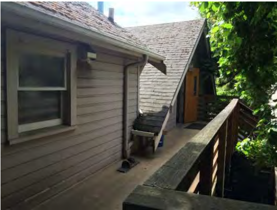
Plant Ops Annex 4_1184_7.JPG
