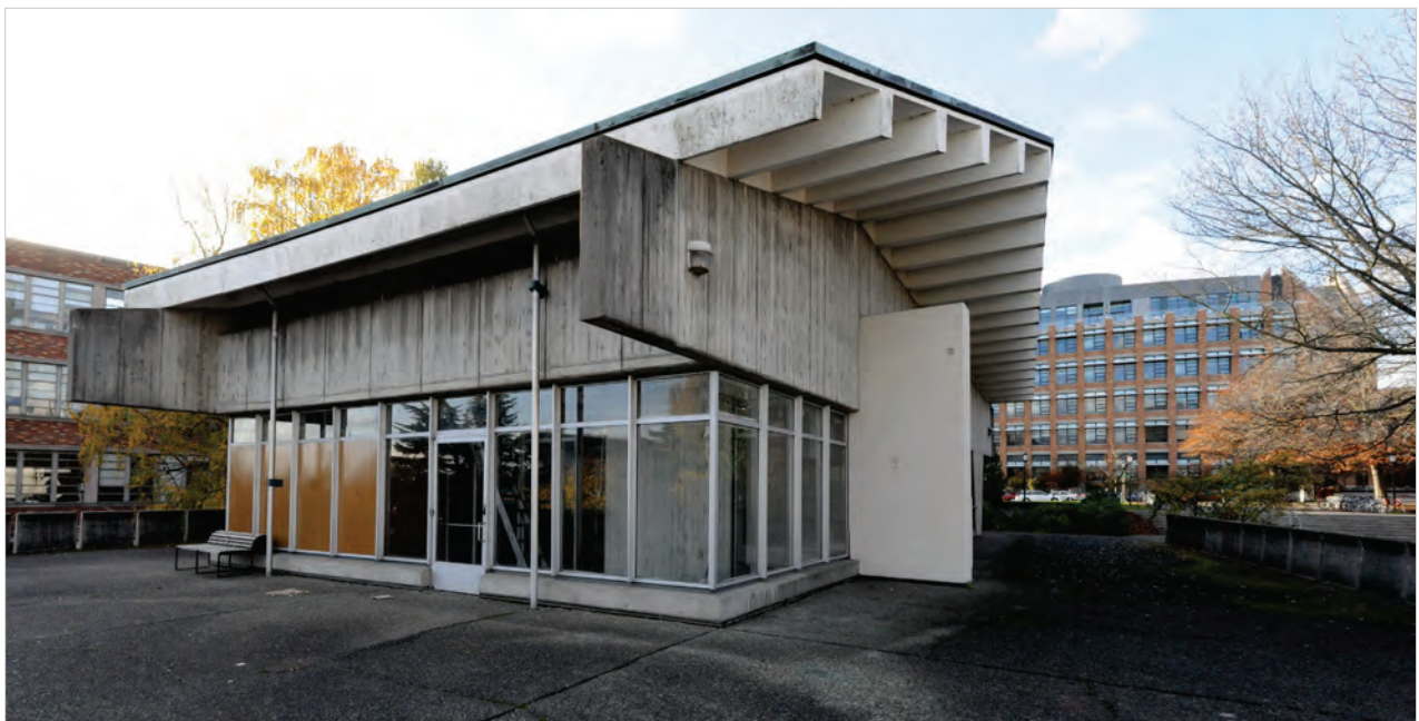
Figure 3-16. Nuclear Reactor Building (More Hall Annex), Now Demolished (courtesy Joe Mabel)
