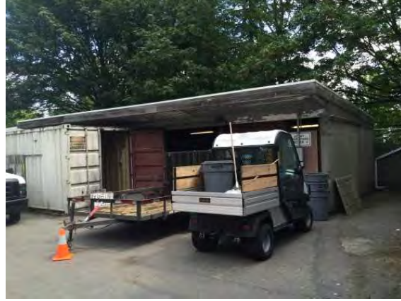
Plant Ops Annex 3_1039_2.JPG
