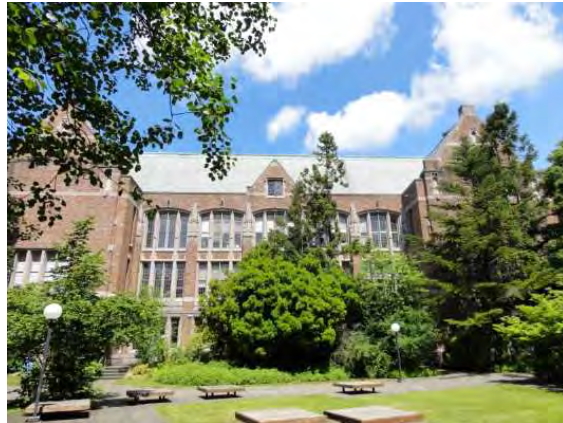
Anderson Hall south elevation
