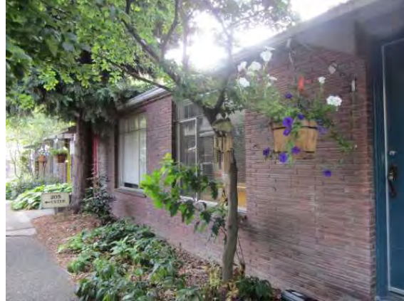
View of North Facade.jpg
