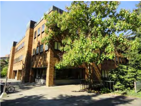
Southeast corner, view to the west
