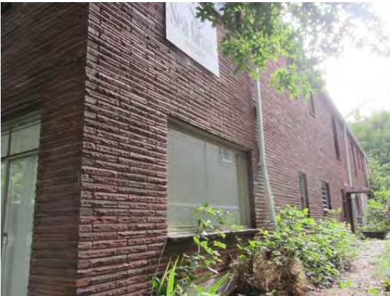
View of South Facade.jpg
