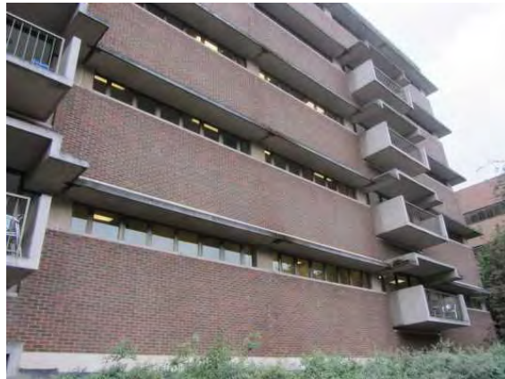
Wing J view to SE.JPG
