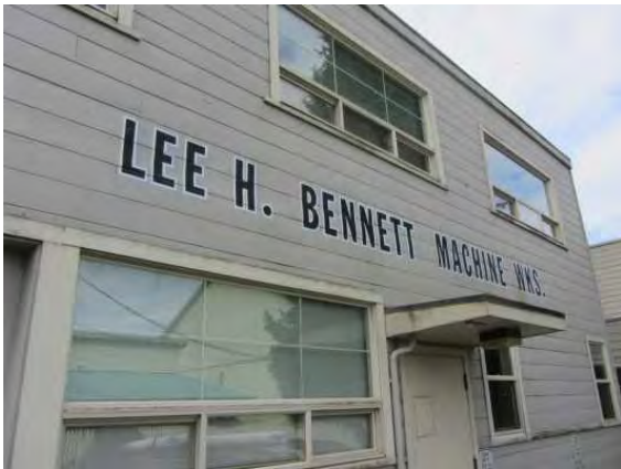
Front Facade Detail.jpg
