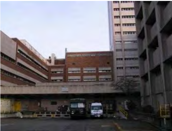
Rear loading dock of Wing AA and east elevation of Wing B. Agaard Tower on right.
