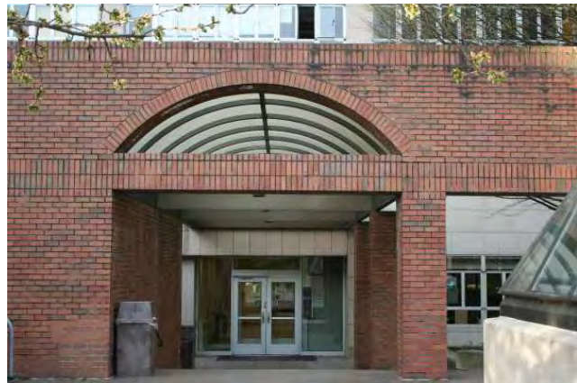
North (front) entry detail
