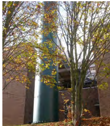
Base of ventilation tower
