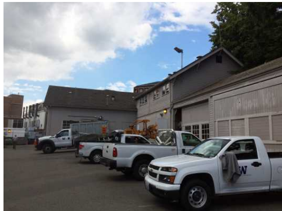
Plant Ops Annex 4_1184_3.JPG
