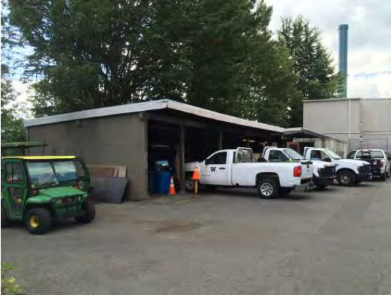
Plant Ops Annex 3_1039_1.JPG
