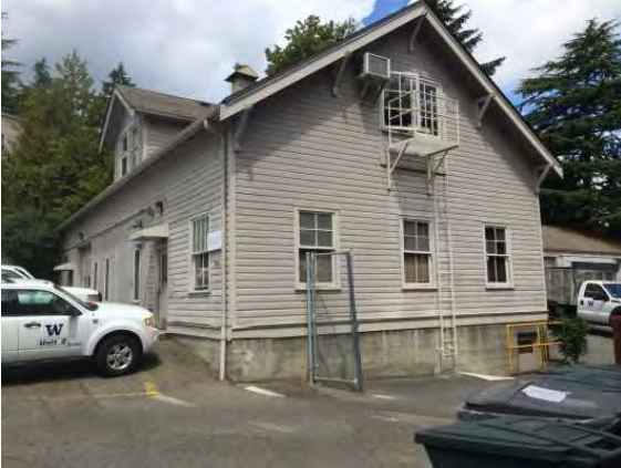
Plant Ops Annex 4_1184_1.JPG
