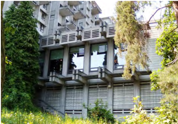
detail of south elevation
