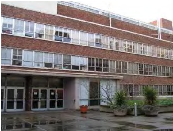
Front elevation of Wing C
