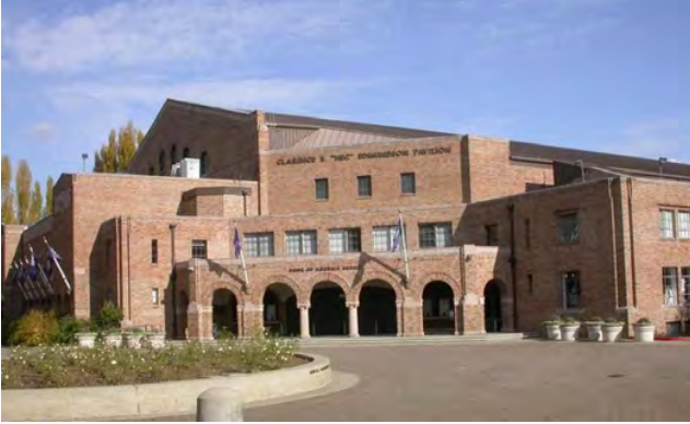
Front elevation with entry
