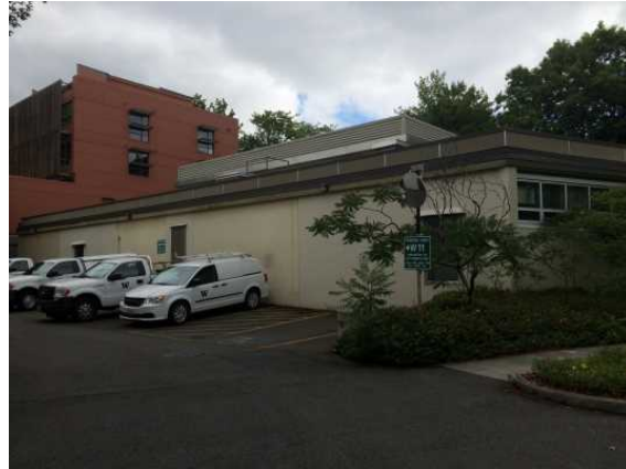
Brooklyn Trail Bldg_1115_5.jpg
