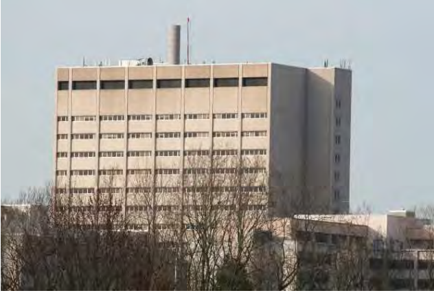
South and east elevations
