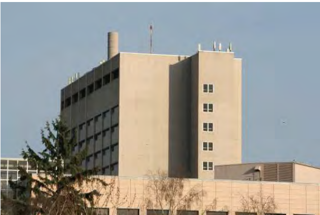
South and east elevations
