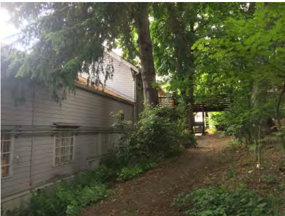
Plant Ops Annex 4_1184_5.JPG
