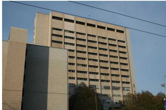
North (front) and east elevations
