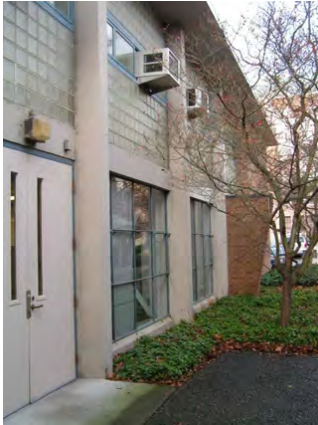
Main elevation, view west
