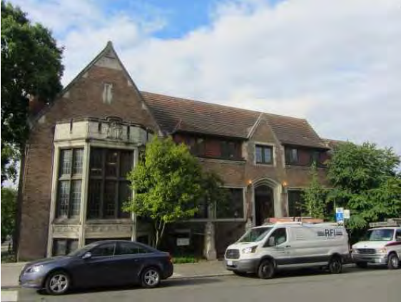
Primary (North) Facade.jpg
