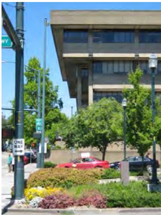
South Elevation (detail), Looking North
