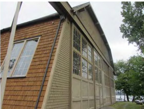
South Doors and Track with Outriggers.jpg
