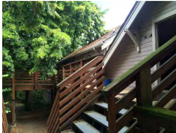
Plant Ops Annex 4_1184_6.JPG
