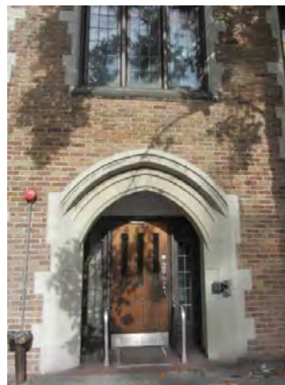
Entry on East Facade.jpg
