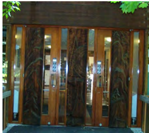
primary entry doors
