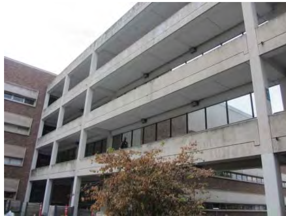
Walkway connecting Wings D and B.JPG
