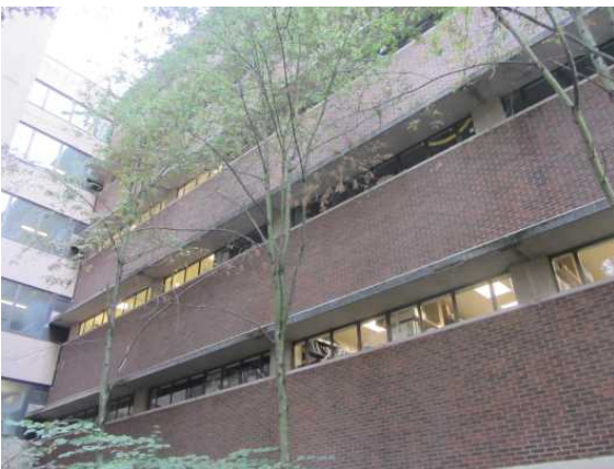
Wing J view to SW.JPG
