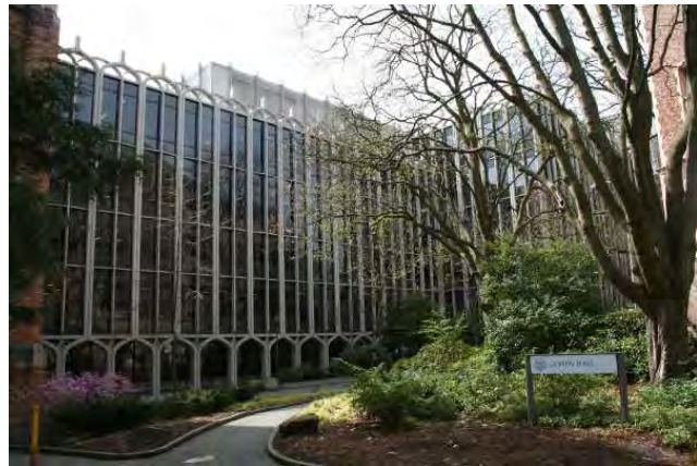
Suzzallo Library, 1963 building, north elevation
