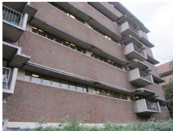
Wing J view to SE.JPG
