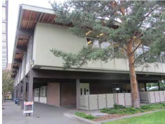
Northeast corner of building.jpg
