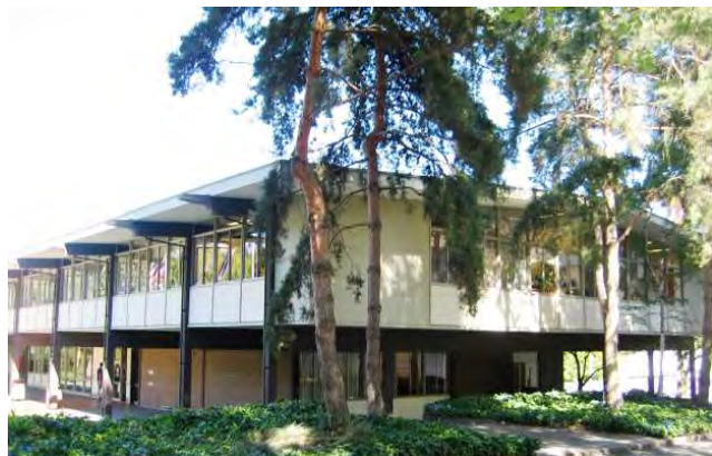
southwest corner of building
