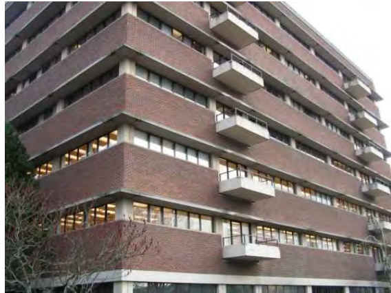
South elevation of Wing D
