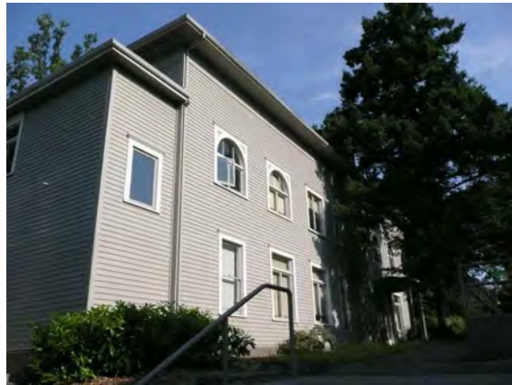
SE corner, southern portion of east (rear) façade
