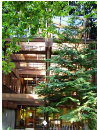
Atrium from south elevation
