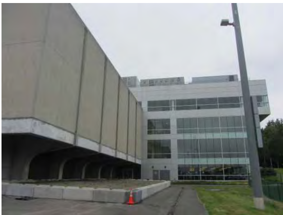
Intersection of new and old building.jpg
