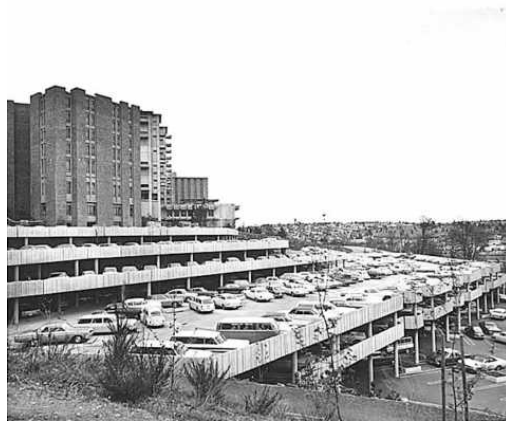
Padelford Garage_1160_5UWLSC UWC0755 1969.jpg
