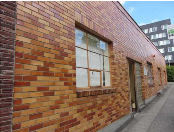
Front East Facade.jpg
