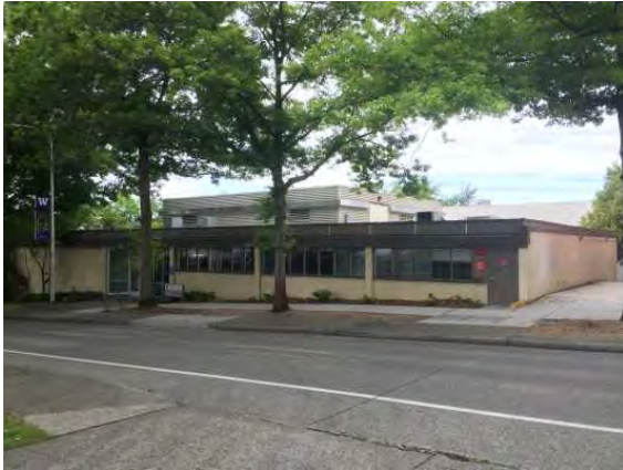
Brooklyn Trail Bldg_1115_1.jpg
