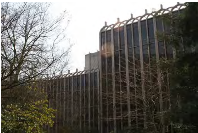
Suzzallo Library, 1963 building, north elevation
