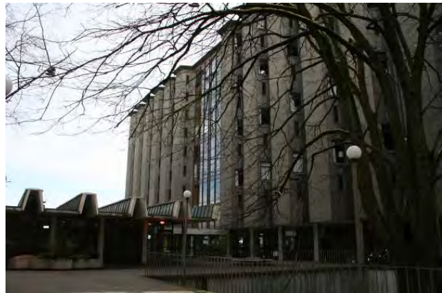
South wing, north elevation, central pavilion
