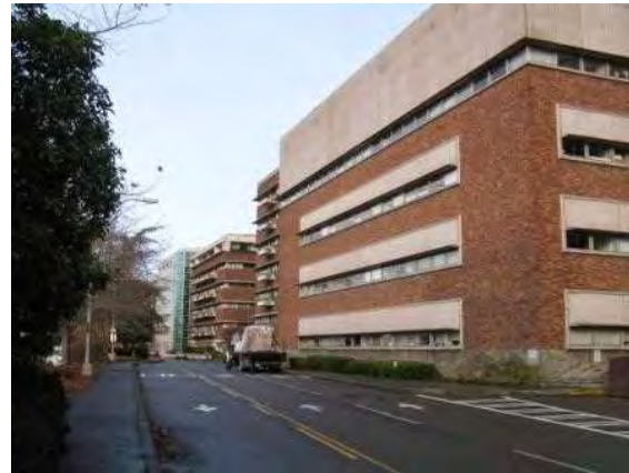
South elevations of Wings B, D, F, and H
