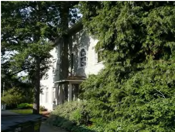
oblique view of east (rear) façade
