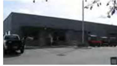
Physical Plant Building
