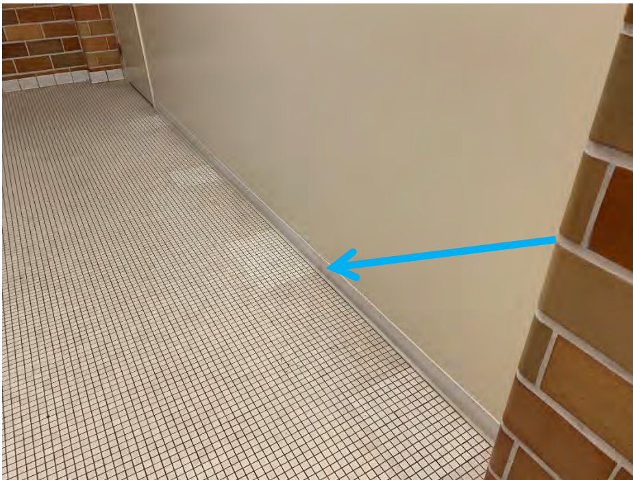
HSA 4. 4" white cove base, yellow mastic and trace joint compound with paint (M)
