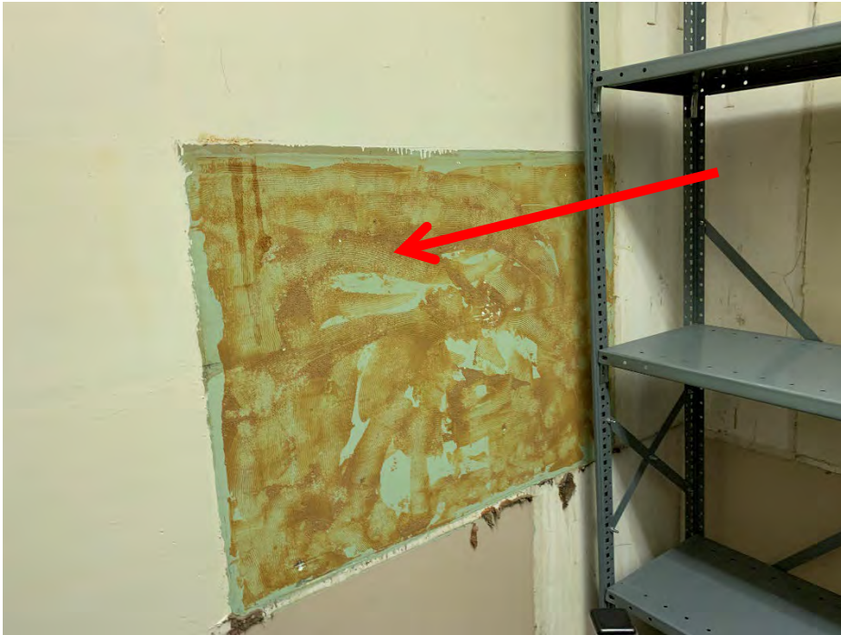
HSA 5. Tan mastic and white crumbly material with paint (M)
