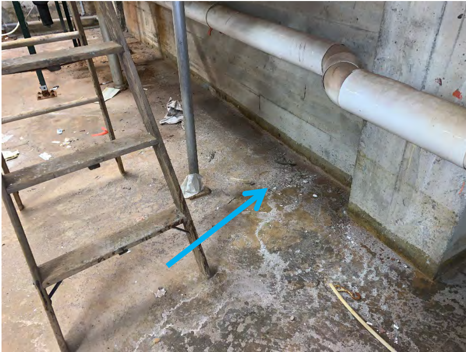
HSA 15. White crumbly material, off-white brittle material, brown/red crumbly material, gray cementitious material with yellow fibrous material, and gray cementitious material (M)
