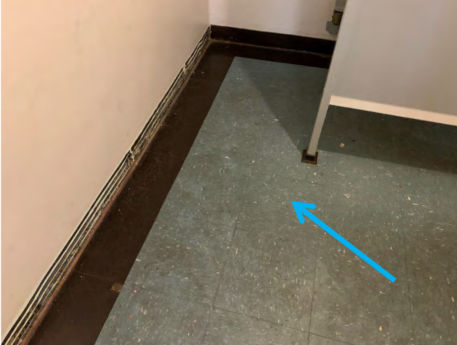
HSA 9. 12"x12" blue vinyl floor tile and black asphaltic mastic (M)
