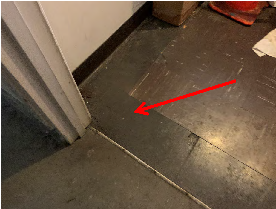
HSA 6. Various sized dark brown vinyl floor tile and black asphaltic mastic (M)
