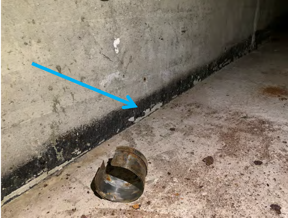
HSA 17. Black asphaltic waterproofing and gray concrete (M)
