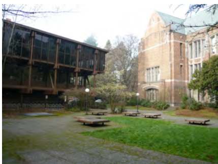
8. View from Courtyard
