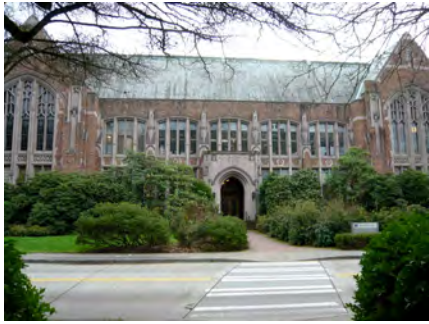
4. View from Island Lane NE
