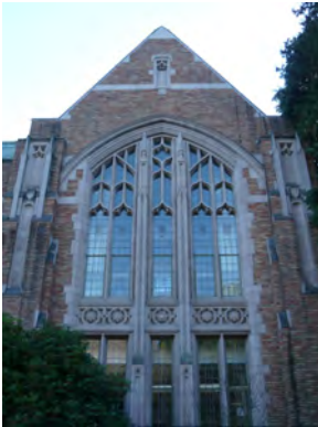
Gable End Windows
