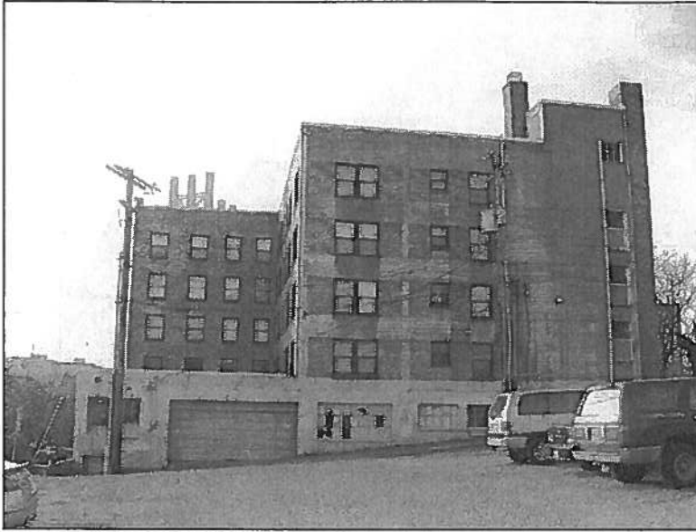
Cavalier Apartments, 1309 NE Campus Parkway, East Elevation
