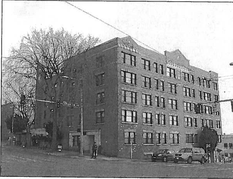
Cavalier Apartments, 1309 NE Campus Parkway, North & West Elevations
