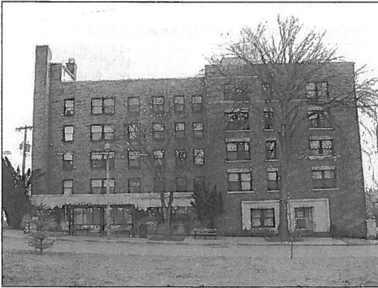
Cavalier Apartments, 1309 NE Campus Parkway, North Elevation
