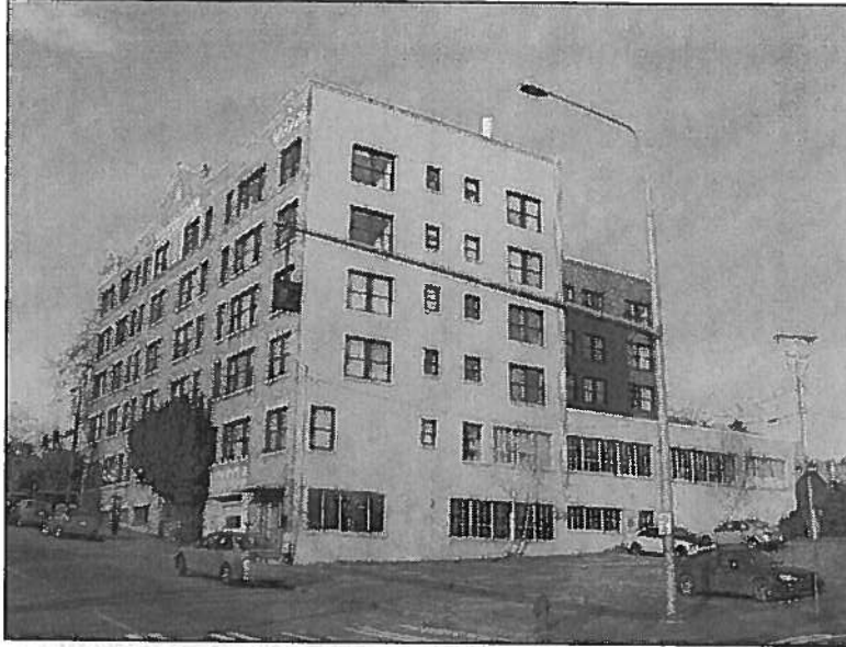
Cavalier Apartments, 1309 NE Campus Parkway, West & South Elevations
