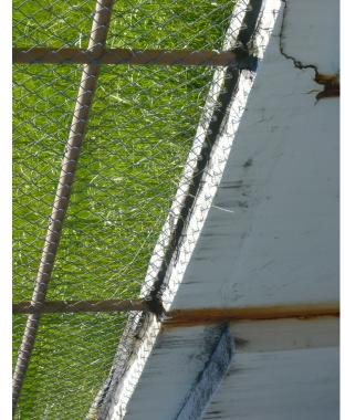
Damage Caused by Guardrail Mounting
