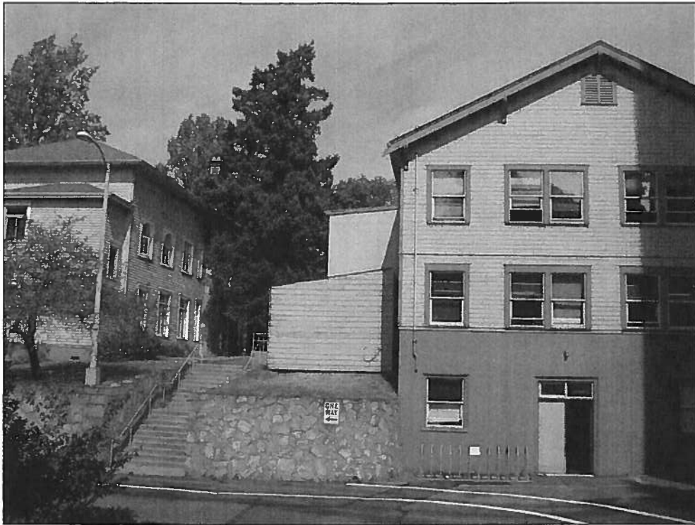
Looking north from the parking lot south of Johnson Annex, showing a partial view of the south facade. Also note the retaining wall and the close relationship to Cunningham Hall (at left).
