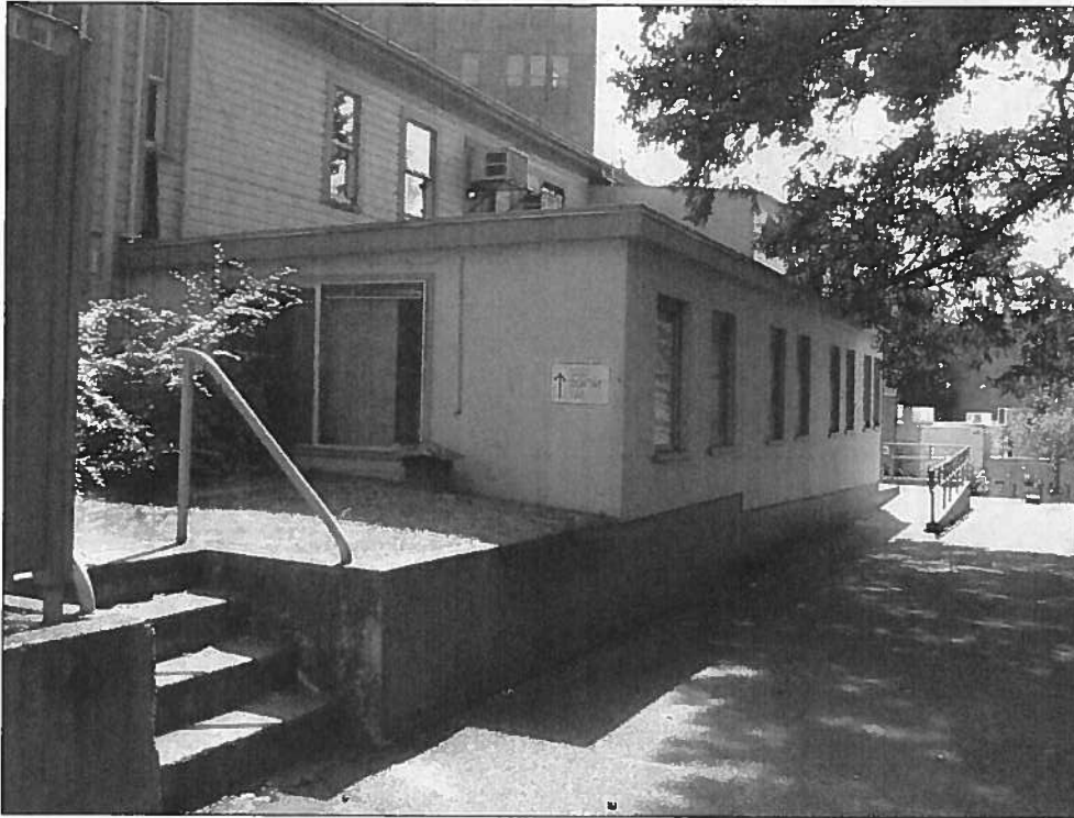
View looking southeast at the southern portion of the west side of the building.
