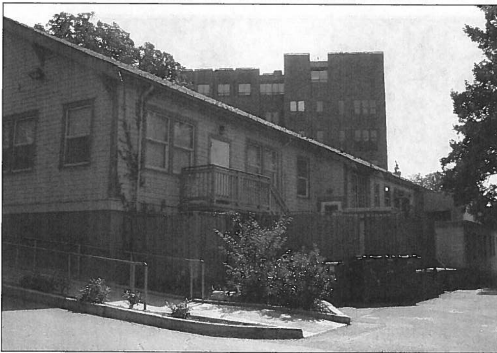
Looking southeast at the northern portion of the west side of the building.
