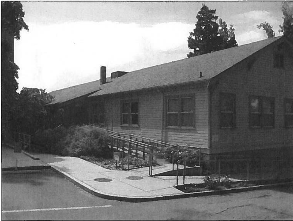
Two views looking southwest at the building, showing the north facade and the northern portion of the primary east facade. Due to the change in grade on the site, the north end of the building appears one-story.
