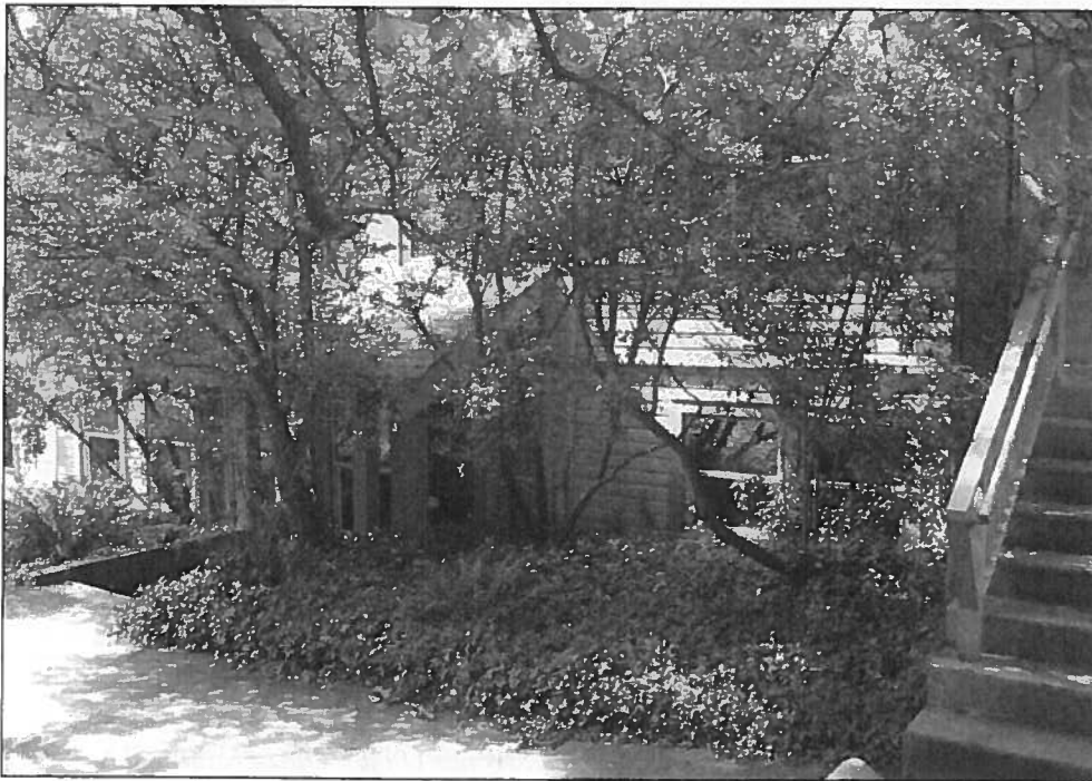
Looking southwest toward the lower level entry on the east facade, obscured by the shrubs. The steps at the far right of the photo lead to the main entry porch.
