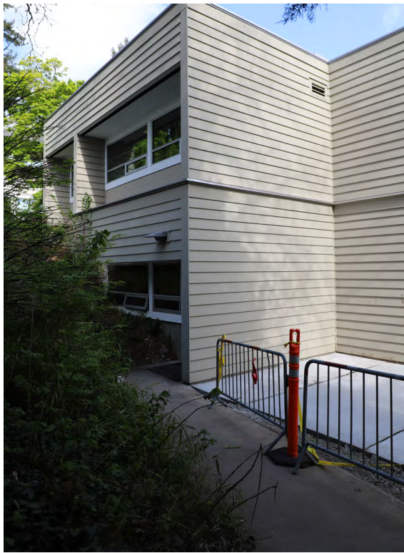
Fig. 6. 2019 view, south facade, looking west.
