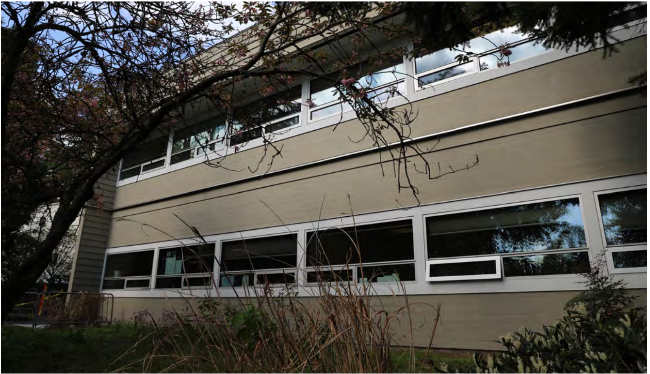
Fig. 4. 2019 view, east facade, looking southwest.
