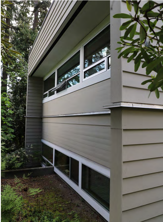
Fig. 3. 2019 view, north facade, looking east.
