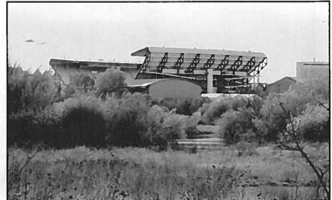
Figure 10 • View F, viewing southwest from the Center for Urban Horticulture
