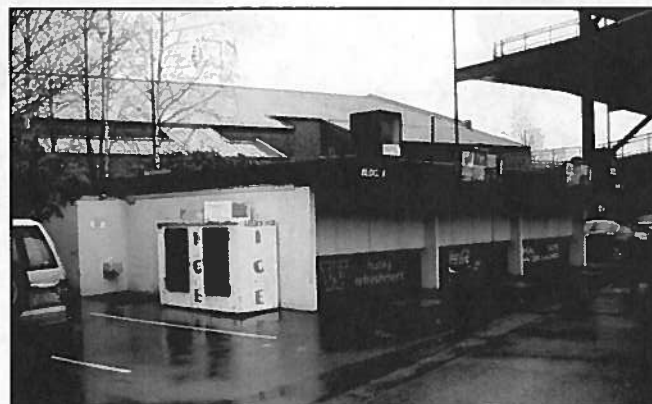
Figure 28 • Building 6, concessions and restroom
