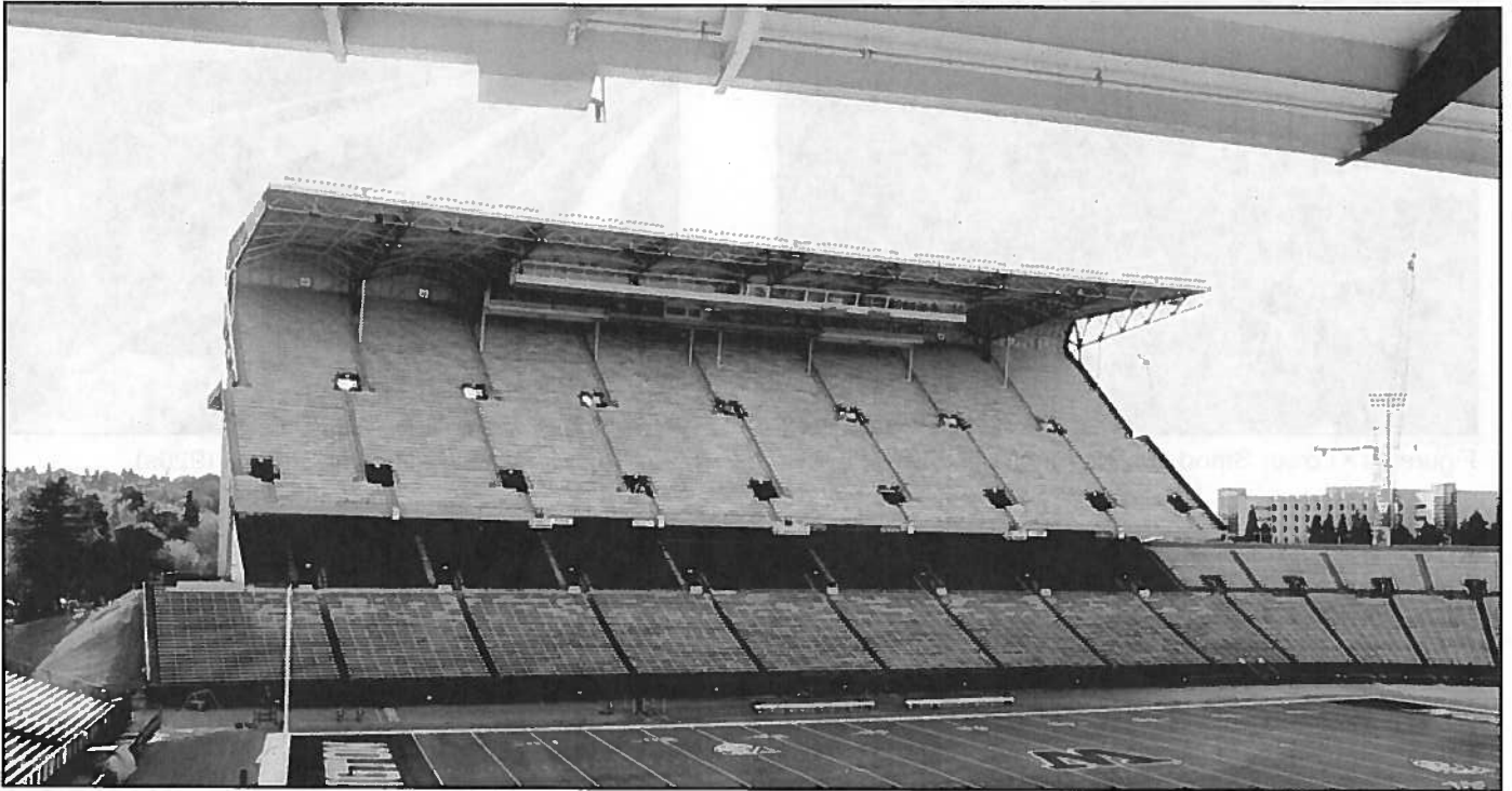
Figure 50 • Viewing south at South Stand Addition, northern side
