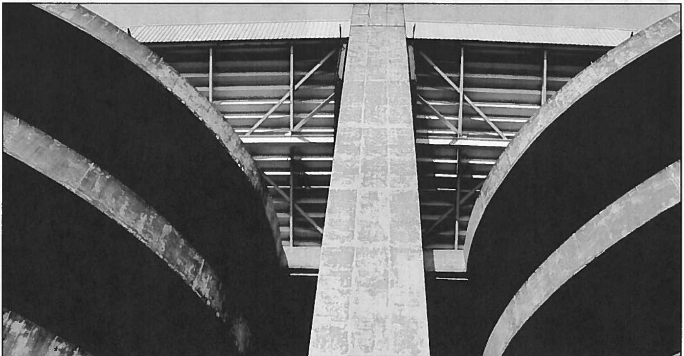
Figure 53 • Detail of South Stand Addition ramps and elevator shaft
