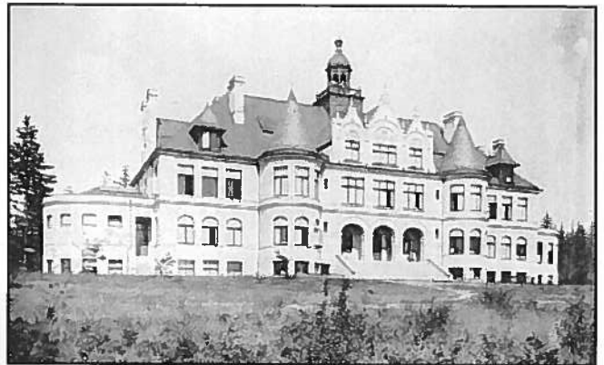
Figure 70 • Administration Building, now Denny Hall (1895, Charles Saunders )
