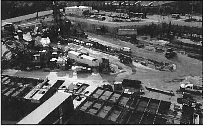
Figure 17 • Light Rail construction site
