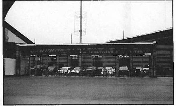
Figure 25 • Northwestern pedestrian entry gate
