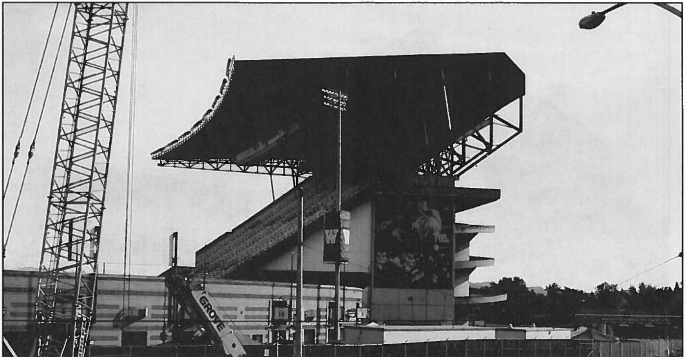
Figure 33 • Viewing east at South Stand Addition, western side
