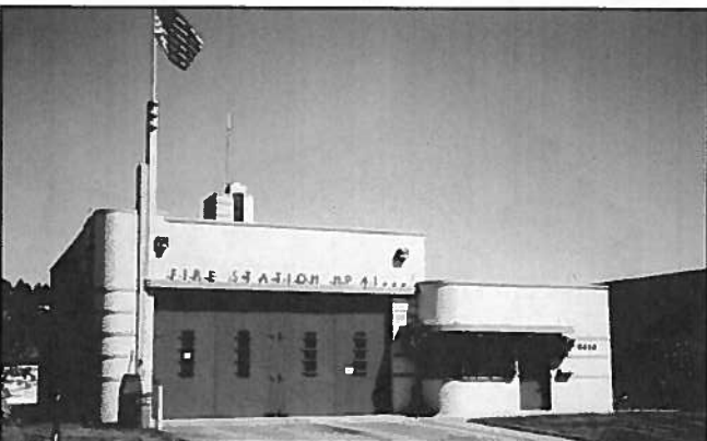
Figure 147 • Fire Station 41, Seattle (1934, Stoddard), n.d.
