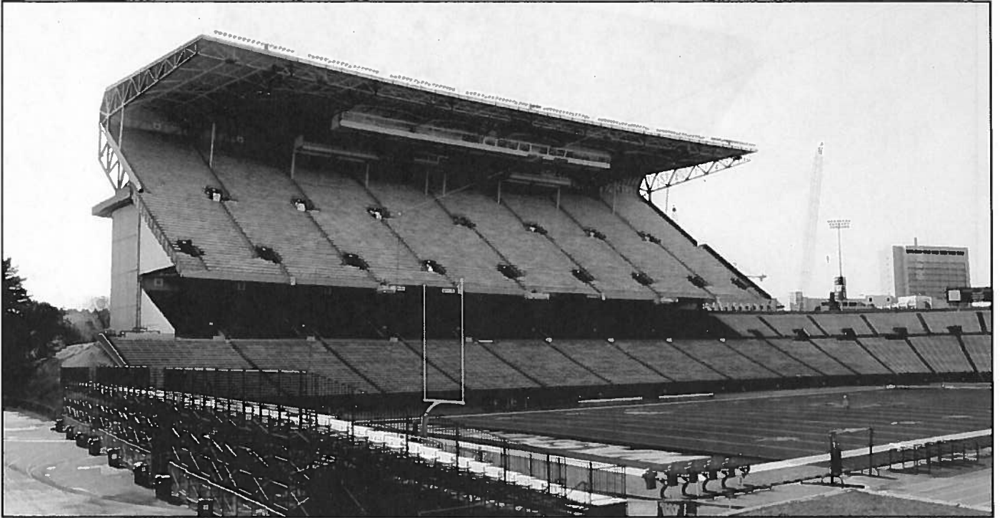
Figure 36 • Viewing southwest toward South Stand Addition
