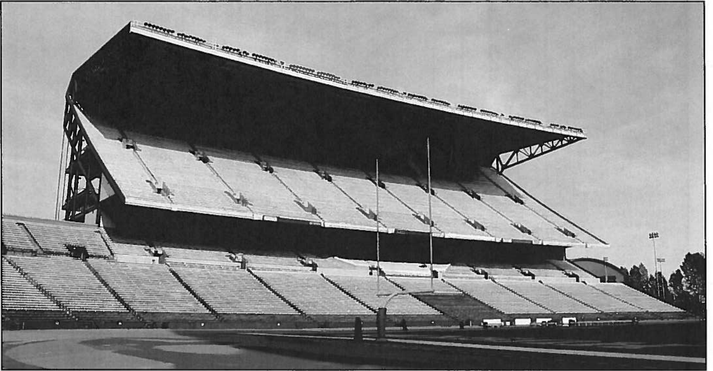
Figure 60 • Viewing north at North Stand Addition
