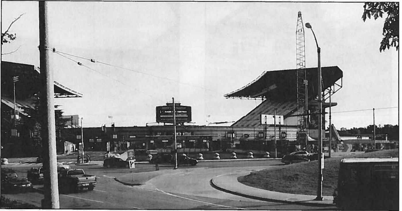
Figure 30 • Viewing east at Stadium entry
