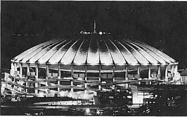
Figure 153 • The King County Domes Stadium, demolished (1972, NBBJ), ca. 1980
