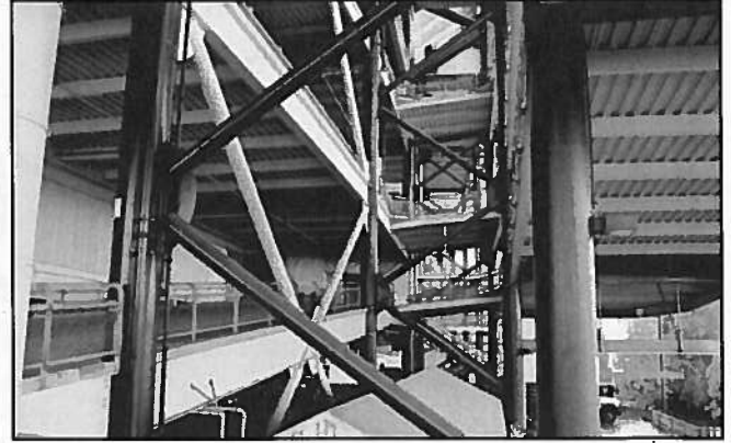
Figure 65 • North Stand Addition structure at upper concessions
