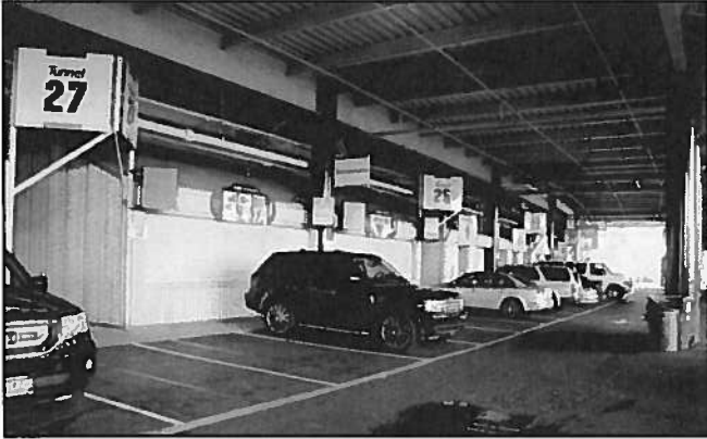
Figure 64 • North Stand Addition lower concessions
