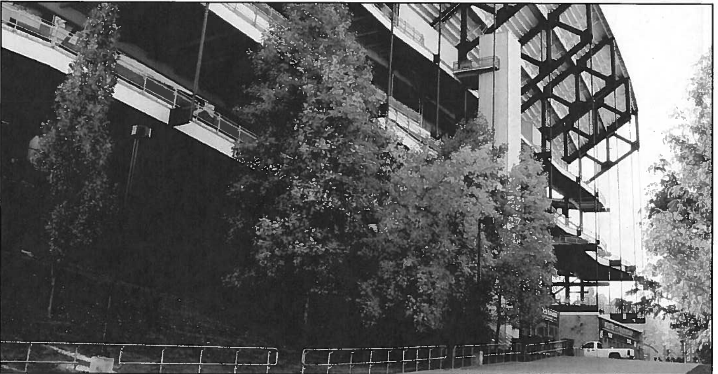
Figure 39 • Viewing west at North Stand Addition, northern side
