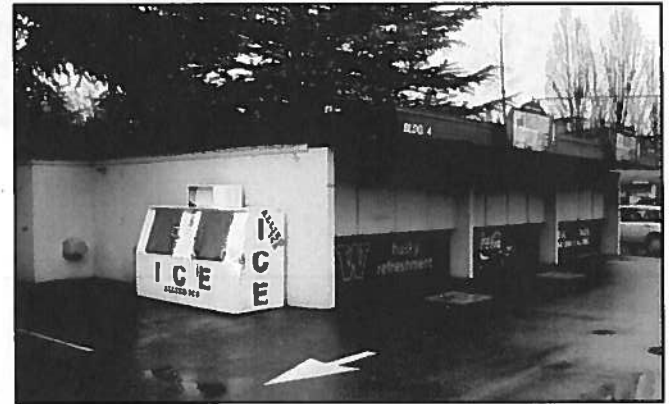
Figure 27 • Building 4, concessions and restroom
