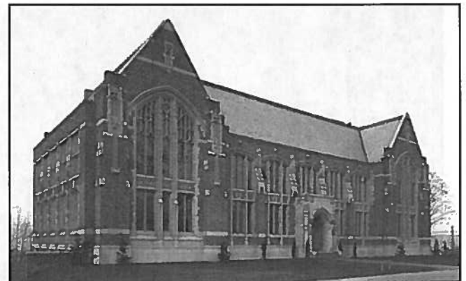
Figure 142 • Anderson Hall Exterior (1925, Bebb & Gould)
