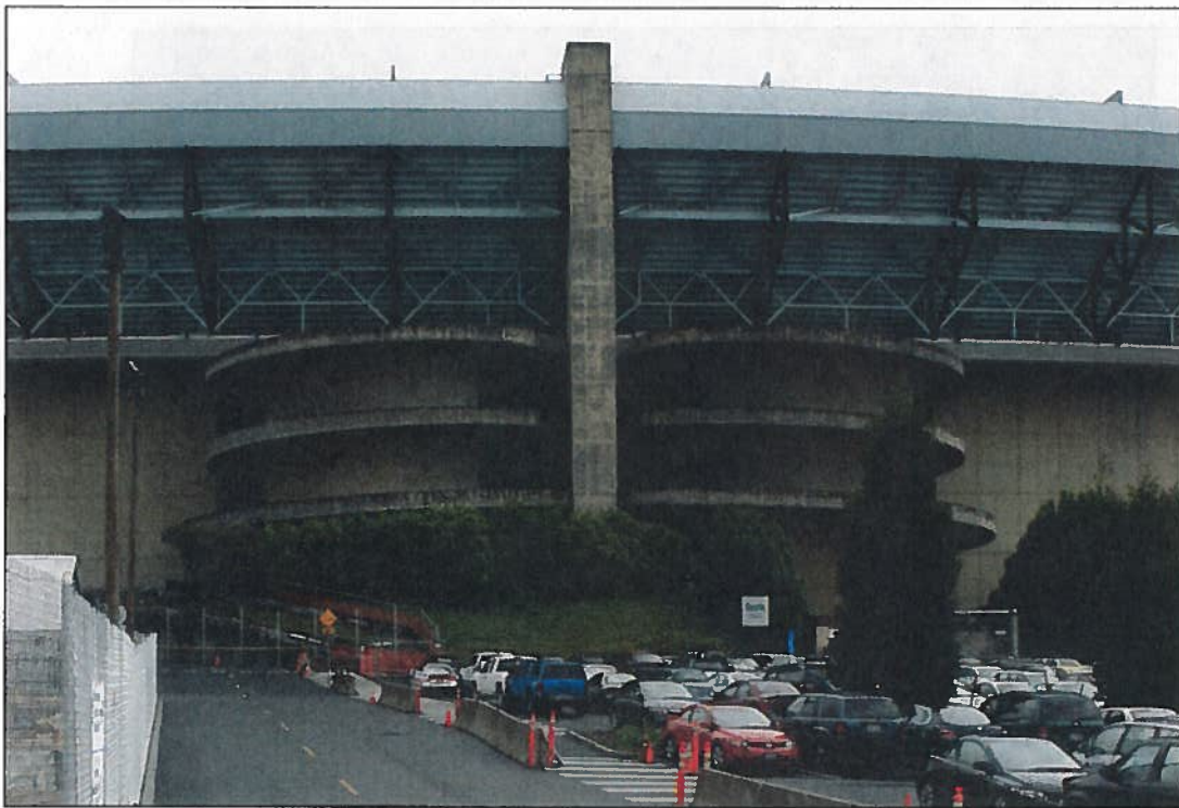
Ramps and partial view of the Stadium South Stands, south façade.
