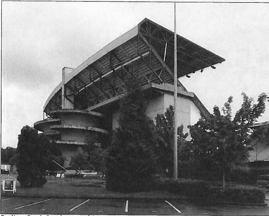
Stadium South Stands, view of the southeast corner.
