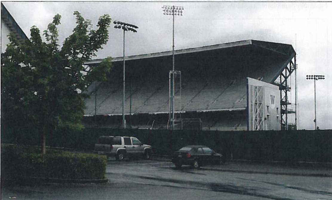
Husky Stadium North Stands, viewed from the southeast parking lot.
