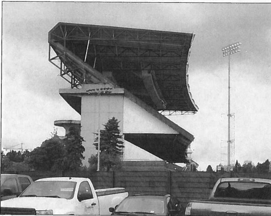
Stadium South Stands, the east elevation.
