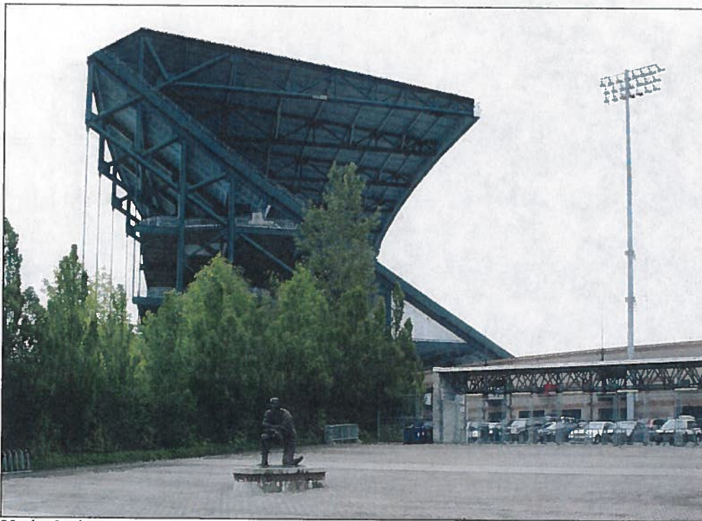
Husky Stadium North Stands, the west elevation and partial view of northwest entry.
