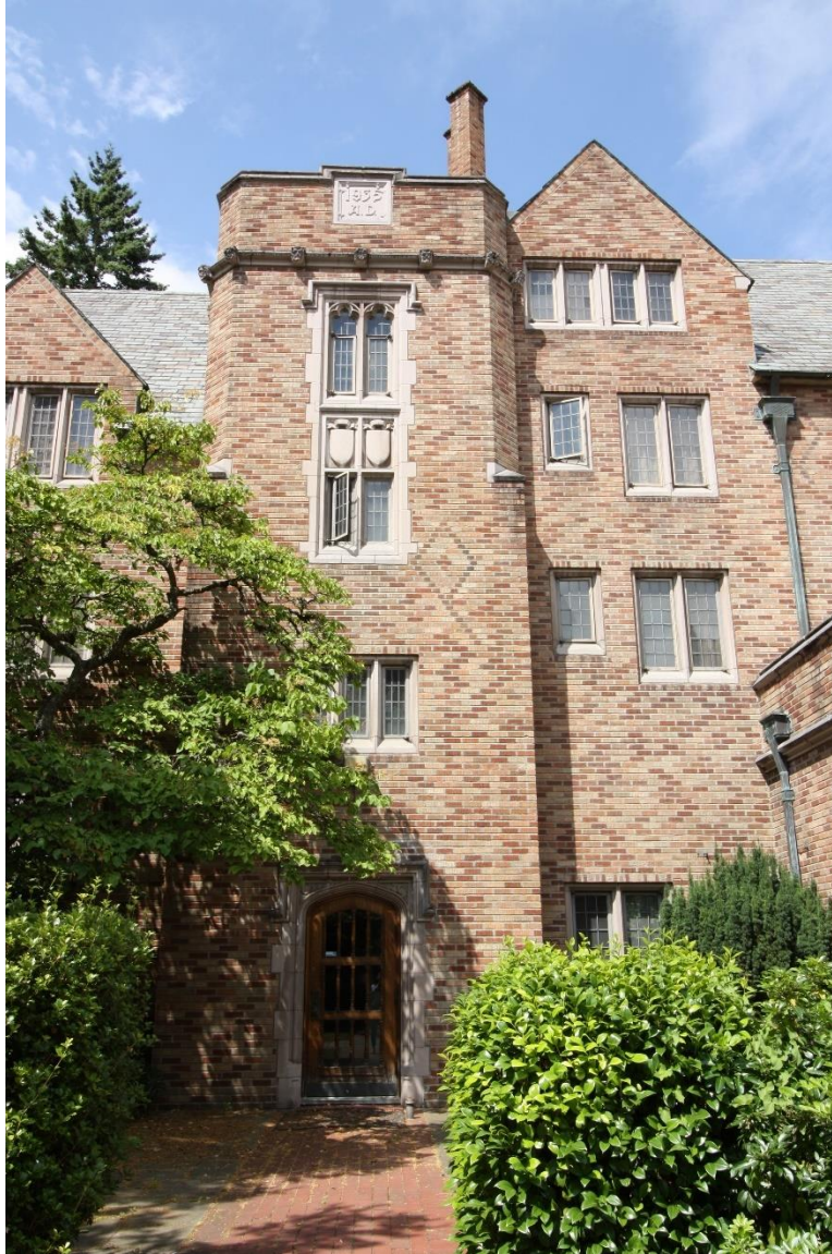
Figure 7: Example of trefoil arch windows, other window types, and example of stair tower.
