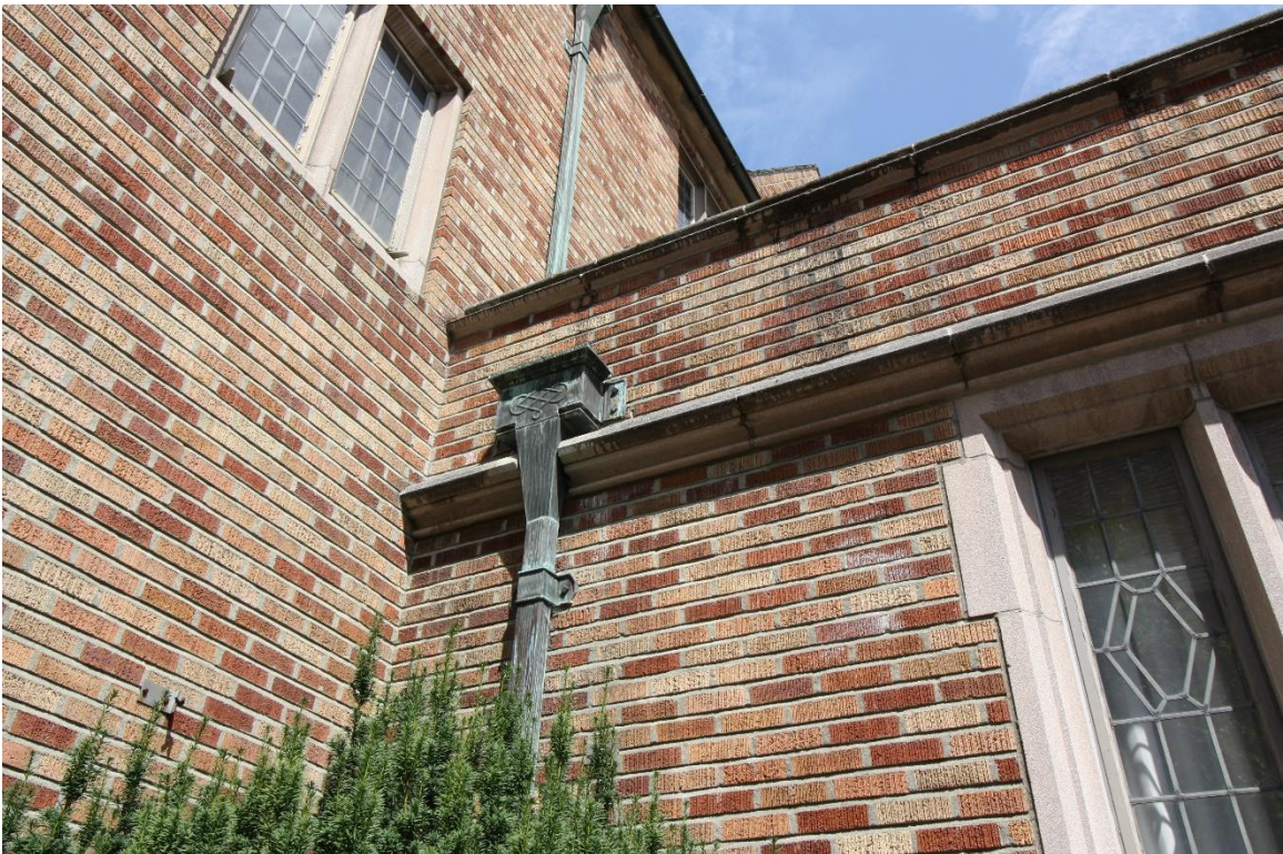
Figure 6: Example of copper leader head, downspout band, and downspout.
