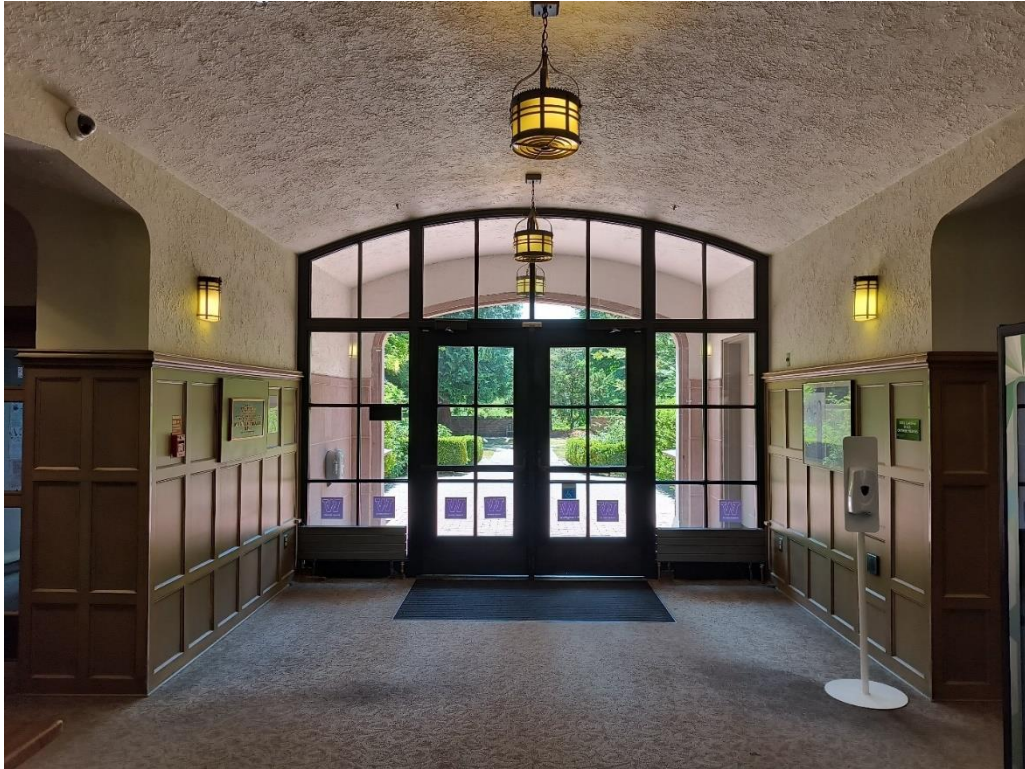
Figure 13: Primary entrance vestibule, facing south.
