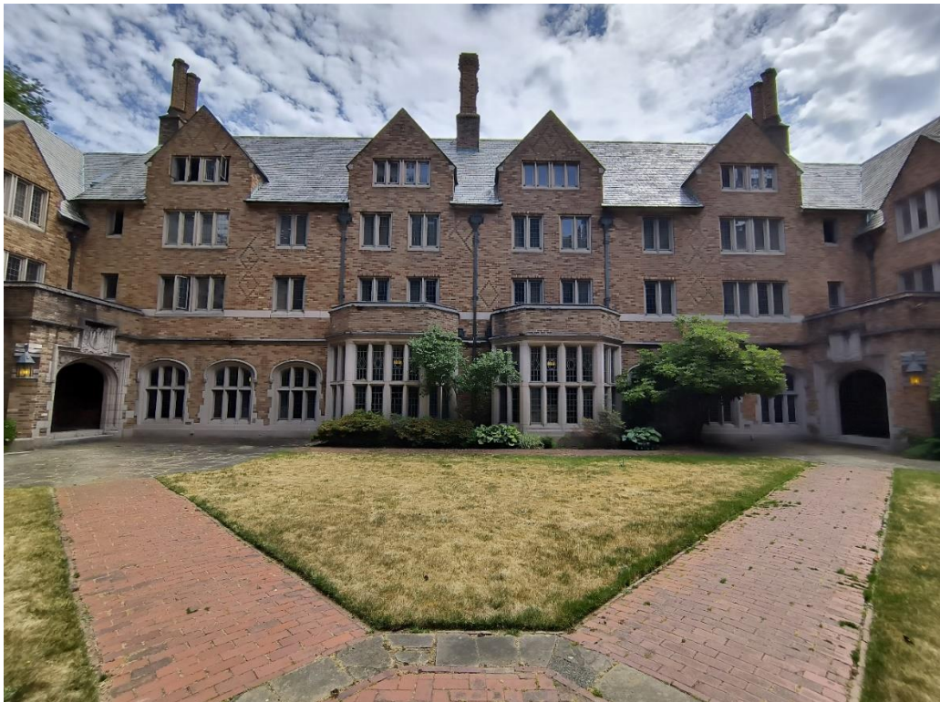
Figure 9: Example of three arched windows with decorative cast stone casing. West elevation in south courtyard, facing east.
