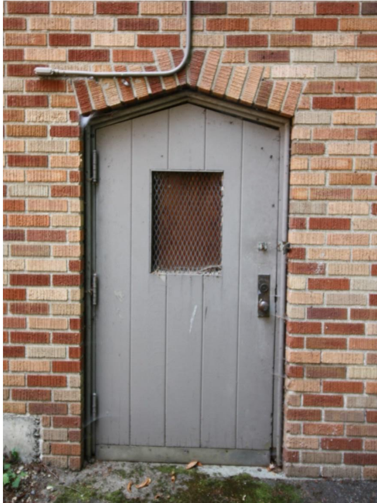
Figure 12: Example of wood plank maintenance door.
