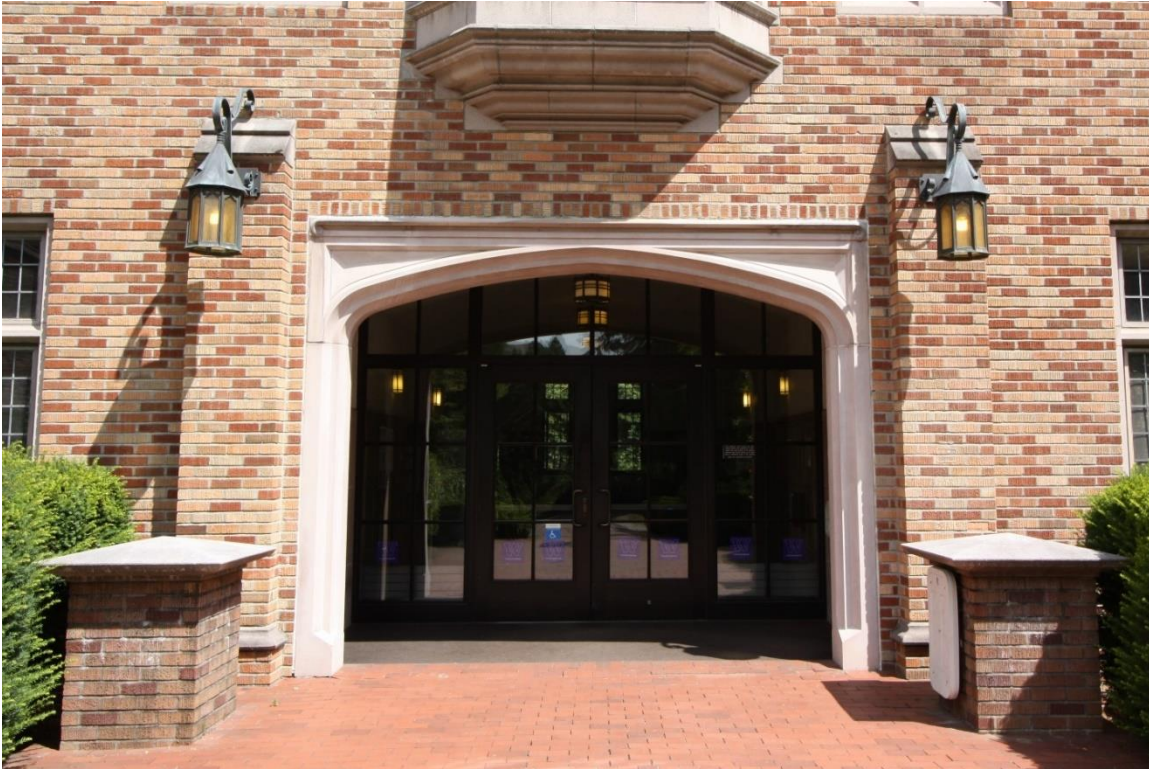
Figure 10: Primary entrance on south elevation, facing north.
